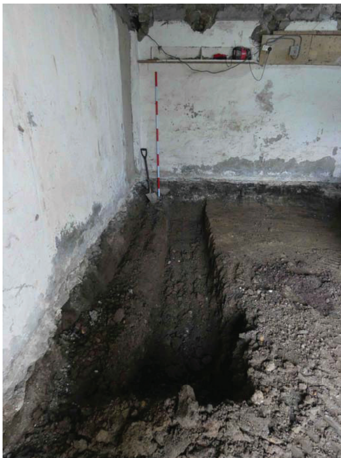
Plate 13: Trench along the south-west side of G1/G2
