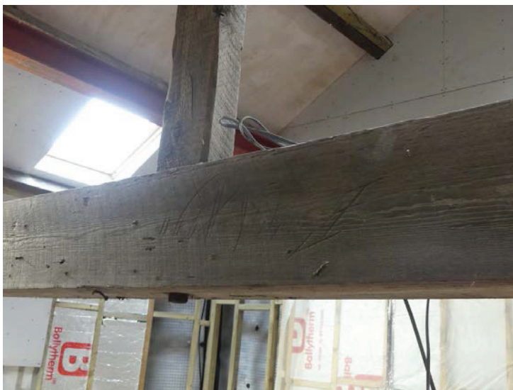
Plate 14 (left): Example of Baltic marks on the south truss, viewed from the north
