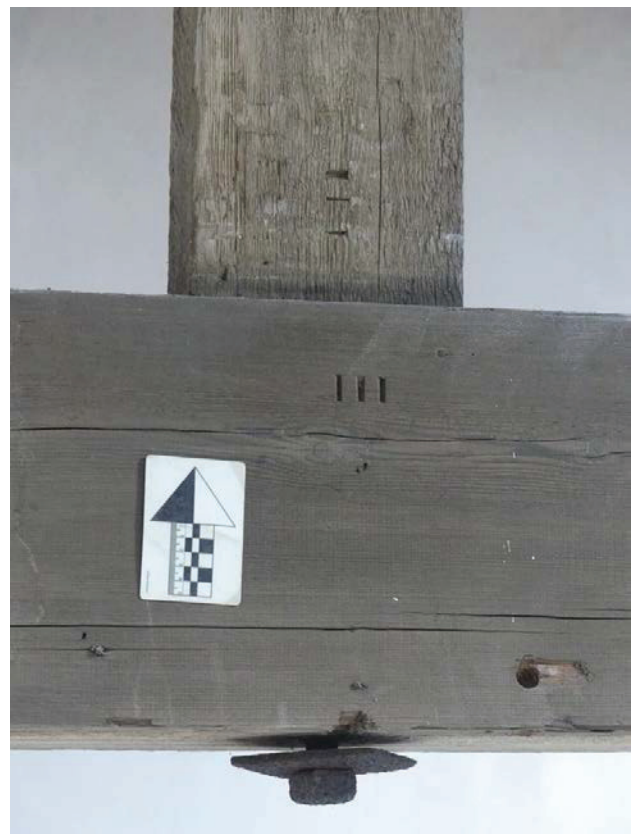
Plate 14 (left): Example of Baltic marks on the south truss, viewed from the north
