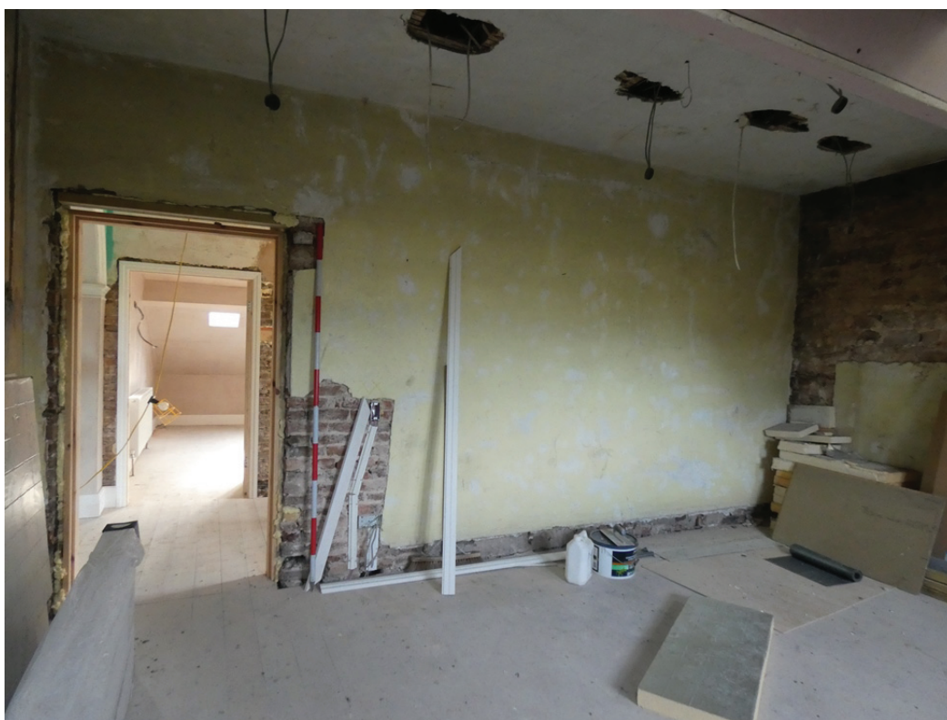
Plate 142: The south elevation in second floor Room 1, viewed from the north
