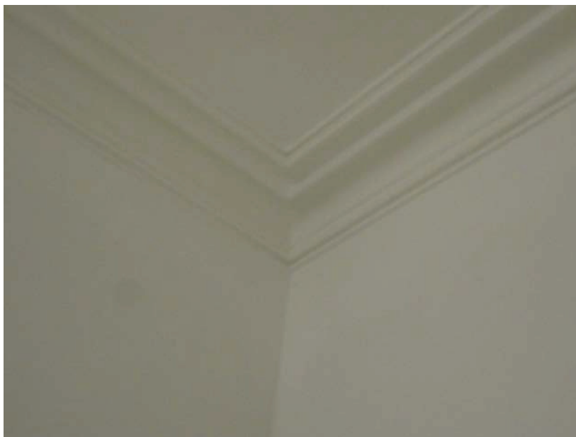
Plate 124: Cornice detail in first floor Room 8, viewed from the north-west
