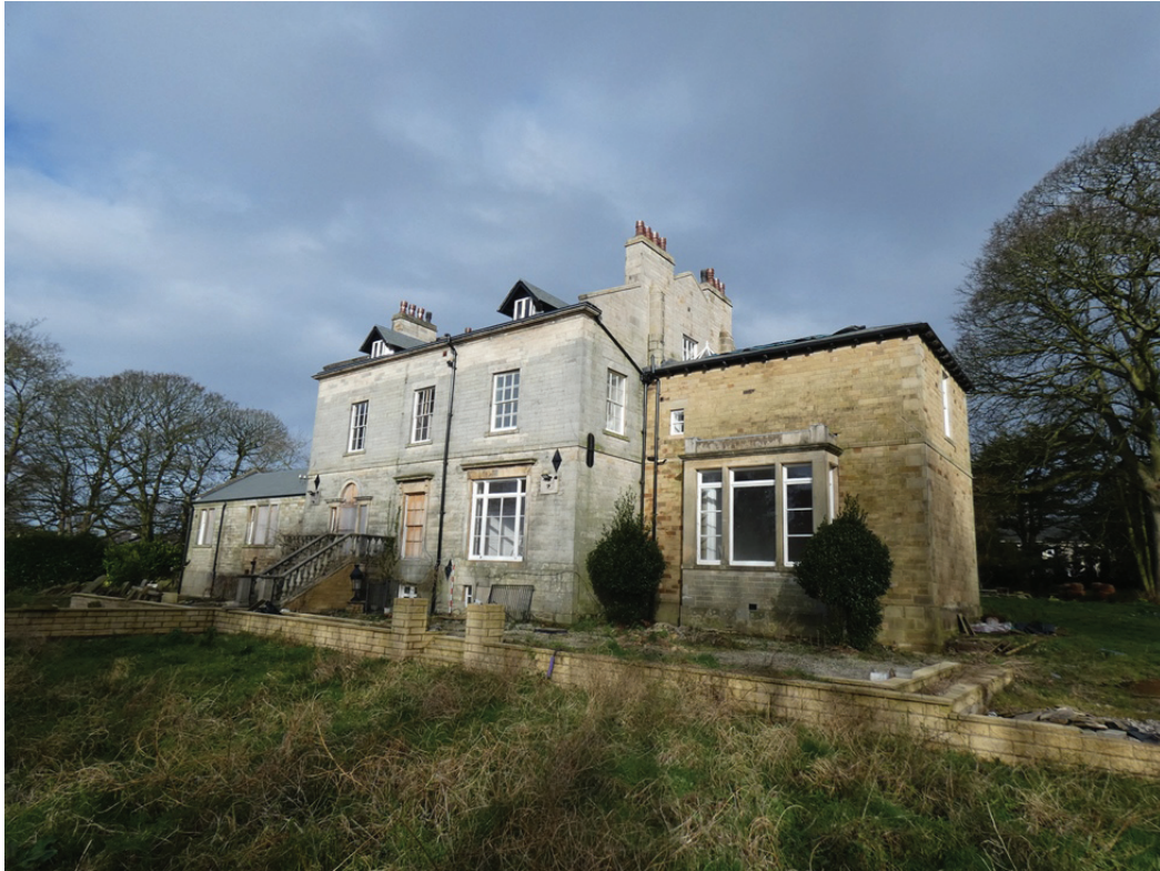
Plate 18: General view of the south external elevation, viewed from the south-east
