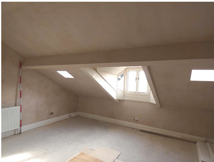
Plate 158: The south elevation in second floor Room 6, viewed from the north-west
