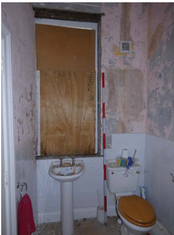
Plate 101: General view of ground floor Room 13, viewed from the north
