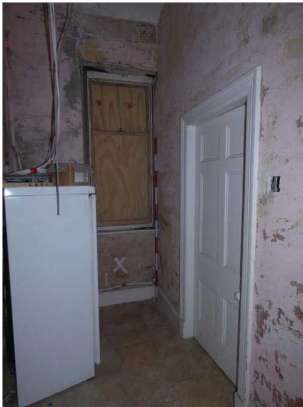
Plate 100: General view of ground floor Room 12, viewed from the north-east
