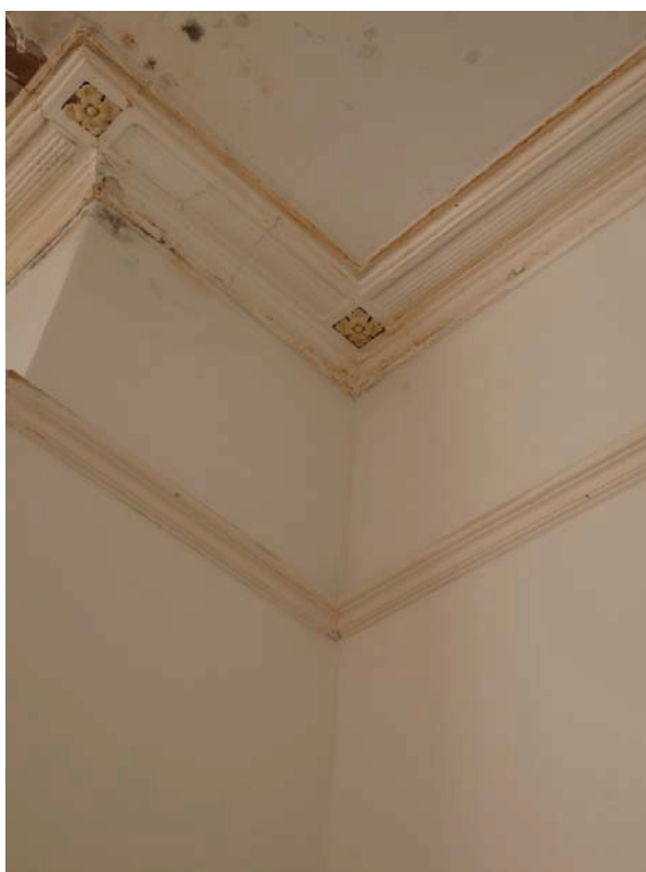
Plate 80: Cornice detail in ground floor Room 6, viewed from the north-east
