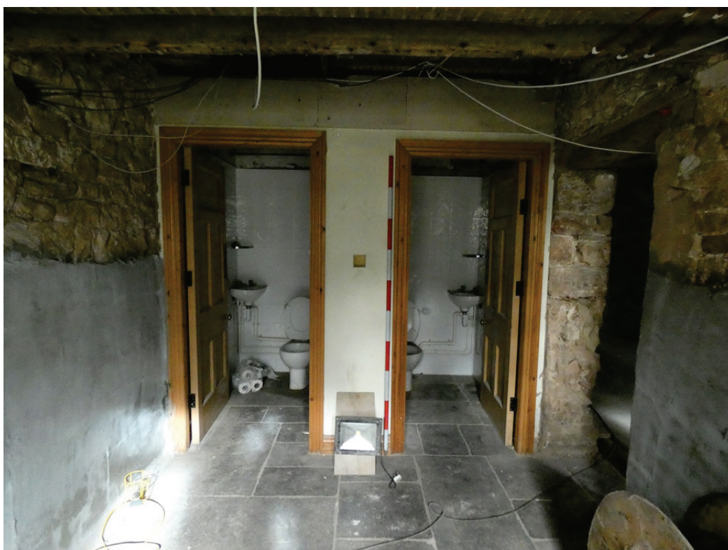
Plate 46: Lower ground floor Rooms 6 and 7, viewed from the south
