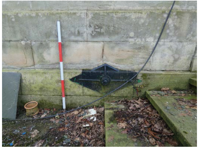
Plate 13 (left): The central and north-west end of the north external elevation, viewed from the north Plate 14 (right): Tie rod plate east of the main entrance in the north external elevation, viewed from the north
