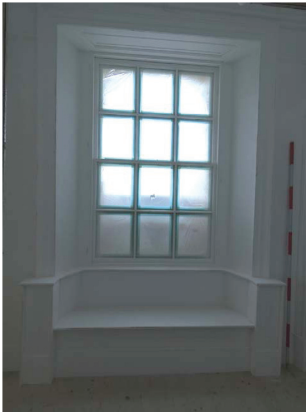
Plate 114: Window seat in the north elevation of first floor Room 2, viewed from the south
