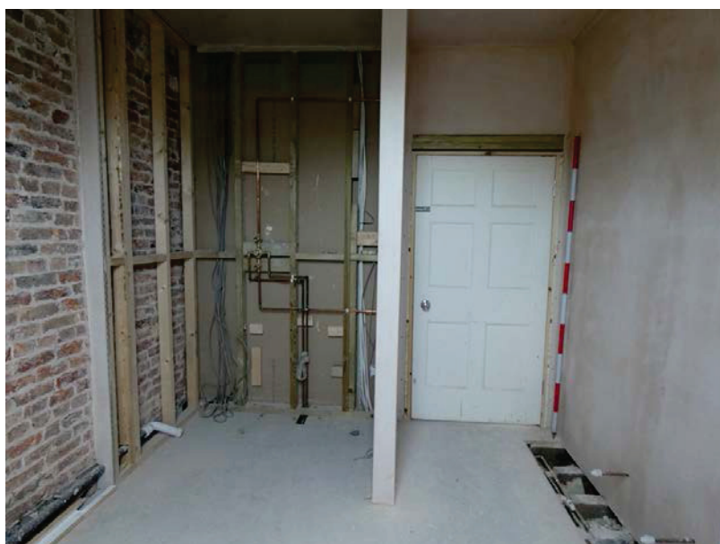
Plate 145: The south elevation in second floor Room 2, viewed from the north
