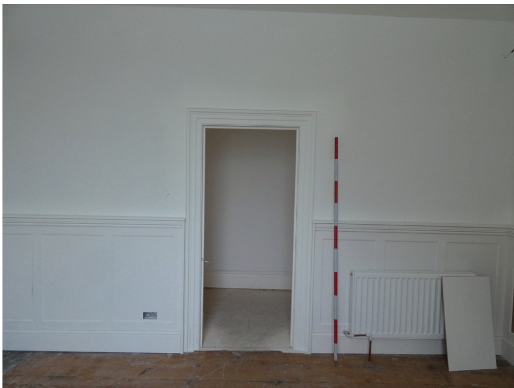
Plate 71: The south elevation in ground floor Room 3, viewed from the north
