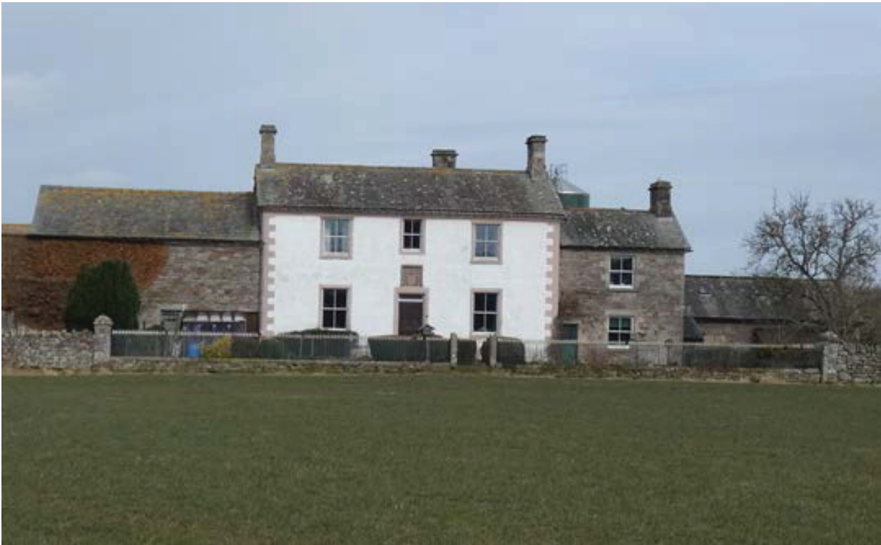
Plate 20: Detailed view of the front (south) elevation of Site 07, viewed from the proposed development area
