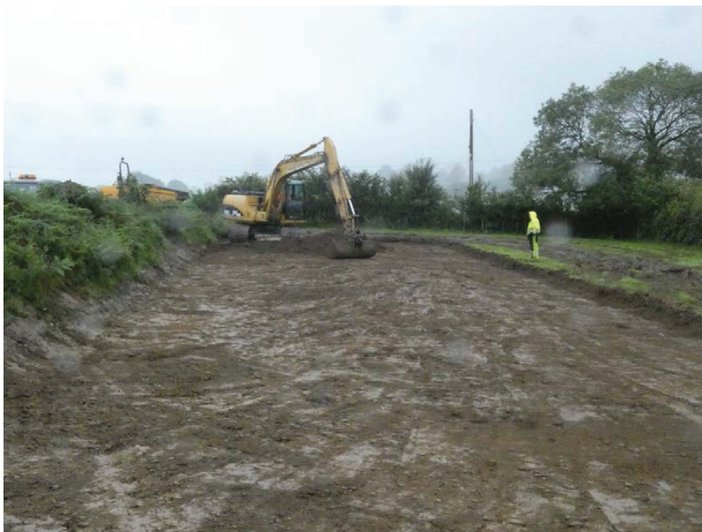
Plate 9: Stripping topsoil
