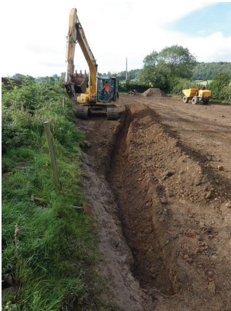
Plate 13: Exposure of the electricity cable, looking south-west
