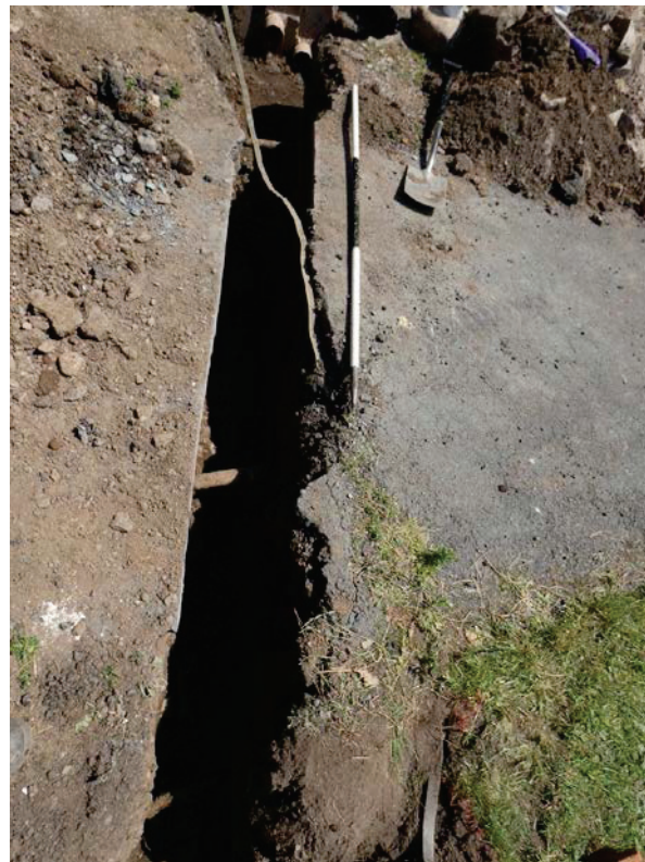
Plate 11 (right): The east end of Trench 2 fully excavated, viewed from the north-west
