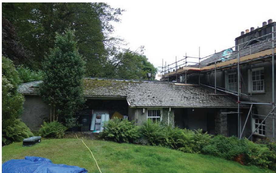
Plate 24: The north elevation of the eastern outshuts, viewed from the north
