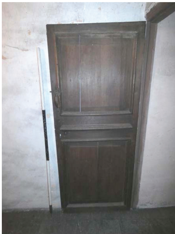
Plate 118: Early door as viewed in Room G6
