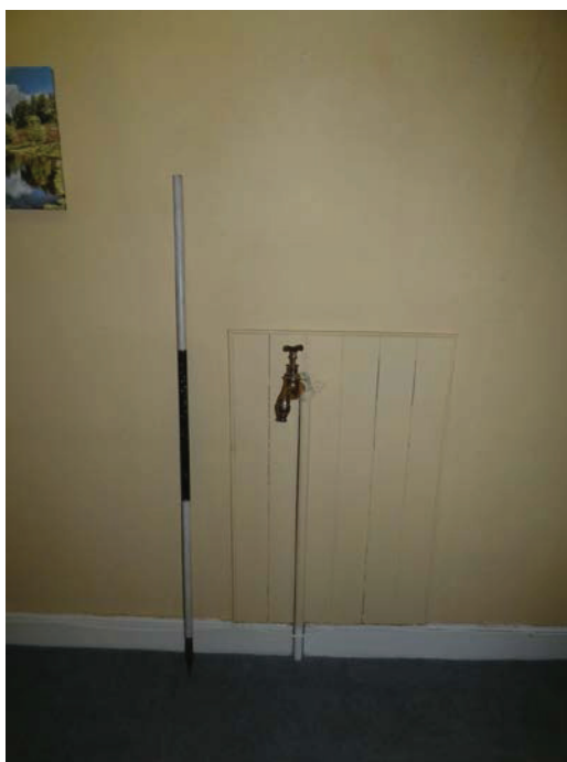
Plate 94: Brass tap and panelling at the north-east end of Room F5, viewed from the north
