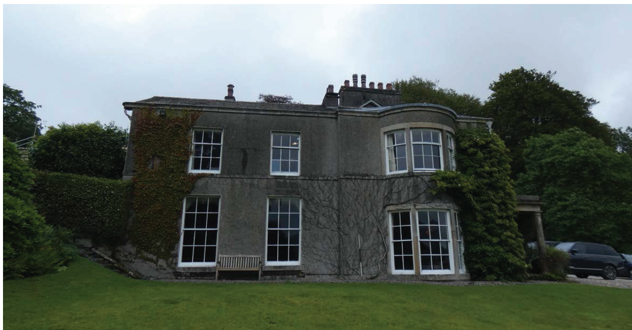
Plate 17: The west external elevation, viewed from the west
