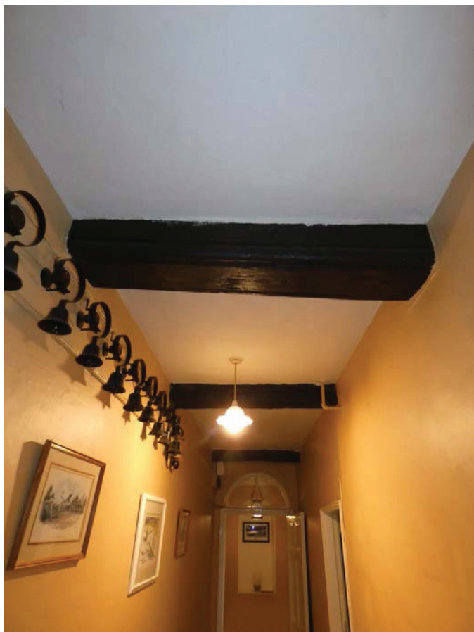
Plate 41 (left): Beams in the ceiling of Room G4, showing the beading, viewed from the east
