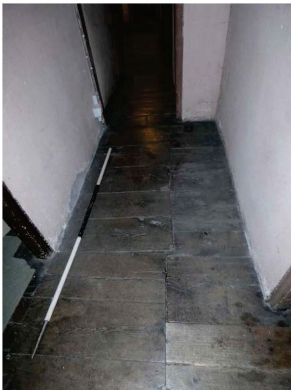
Plate 107: Floorboards in Room S2, viewed from the east
