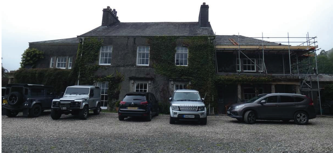
Plate 12: The south external elevation, viewed from the south
