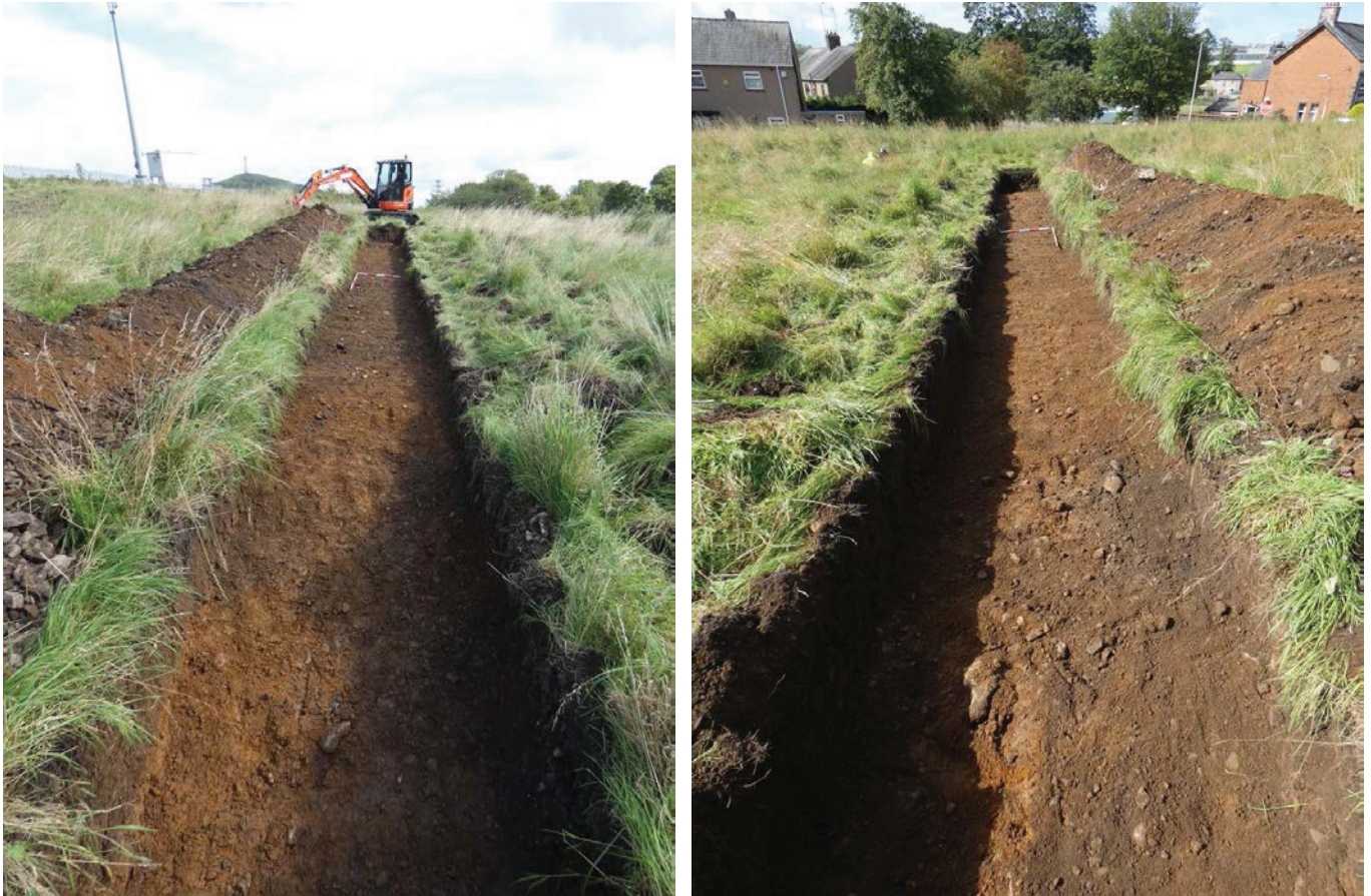
Plate 23 (left): Trench 4 excavated, viewed from the south-west
