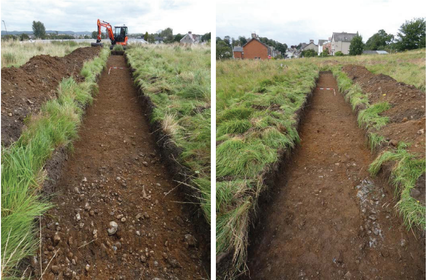
Plate 25 (left): Trench 5 excavated, viewed from the west
