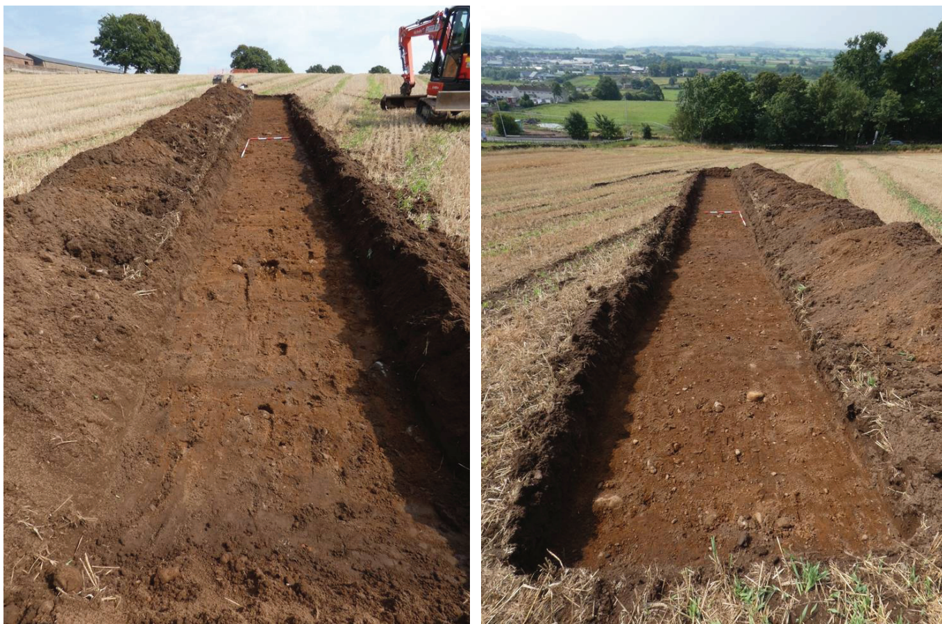
Plate 36 (left): Trench 8 following excavation, viewed from the south-west
