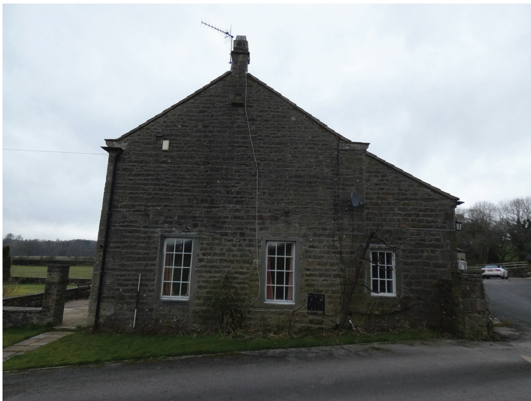
Plate 19: The south external elevation, viewed from the south
