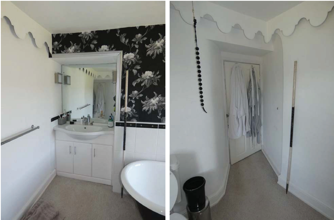
Plate 76 (left): Alcove on the east side of the south elevation, viewed from the north
