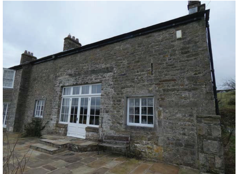
Plate 22 (left): The blocked doorway and inserted window in the south end of the west external elevation, viewed from the west
