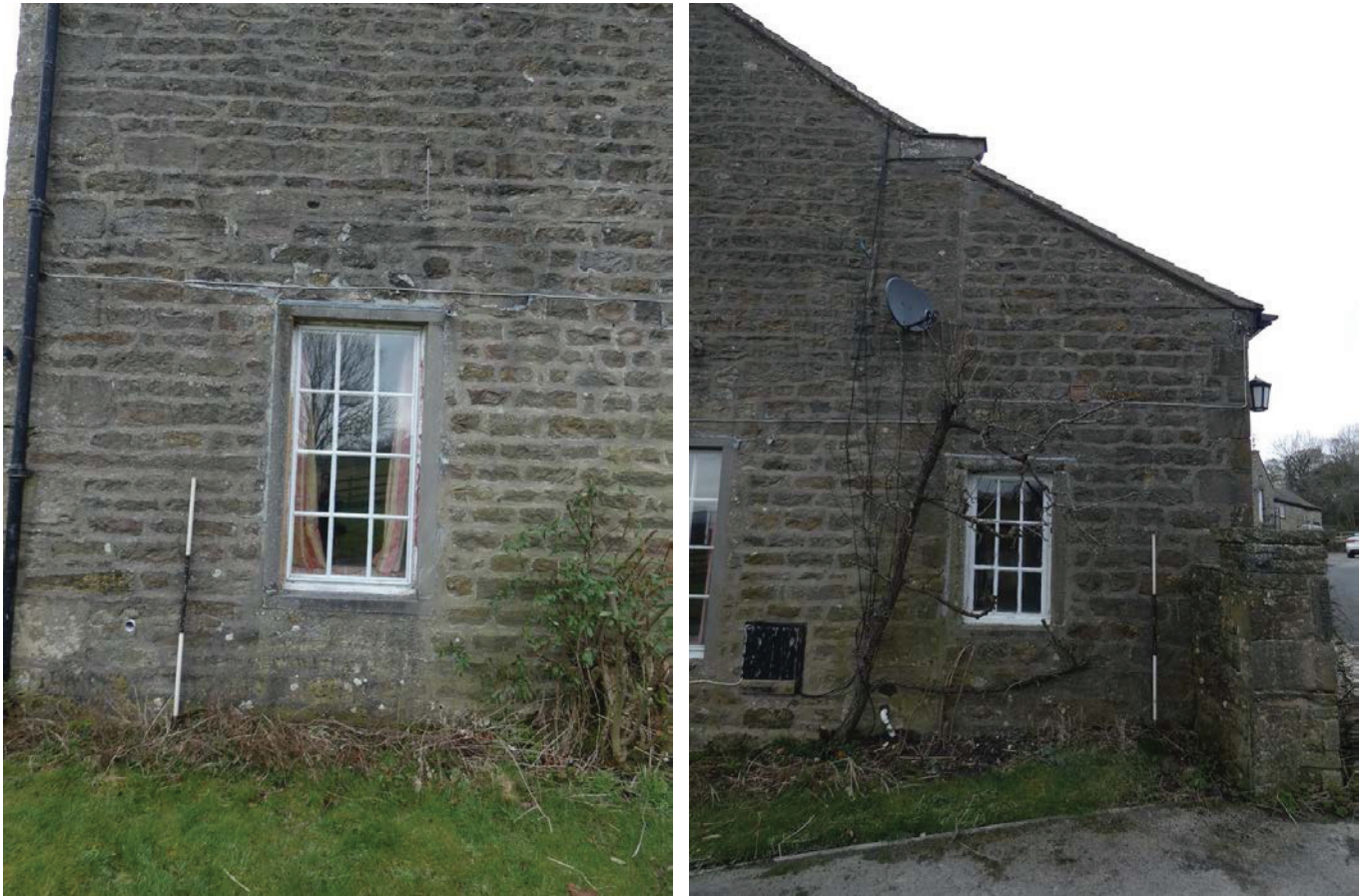
Plate 20 (left): Detail of inserted window in the south external elevation, viewed from the south
