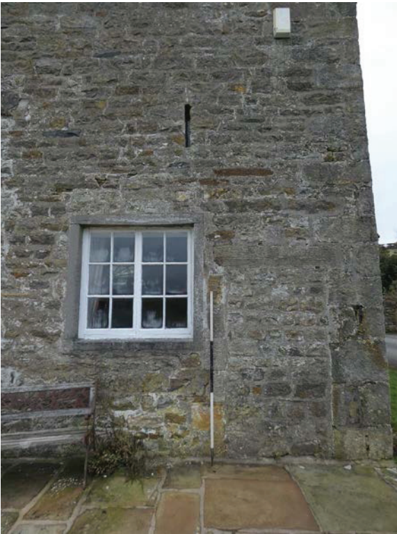
Plate 22 (left): The blocked doorway and inserted window in the south end of the west external elevation, viewed from the west
