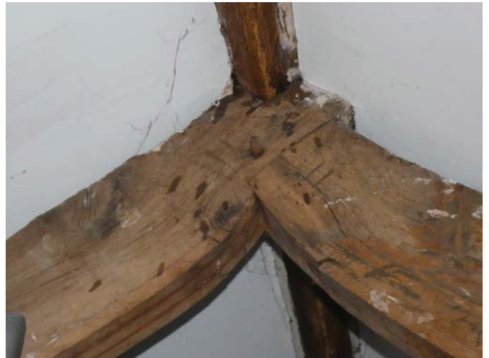
Plate 80 (left): Carpenter's marks 'I' at the top of the north truss, viewed from the north
