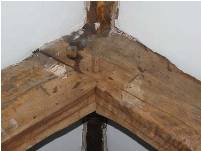
Plate 80 (left): Carpenter's marks 'I' at the top of the north truss, viewed from the north
