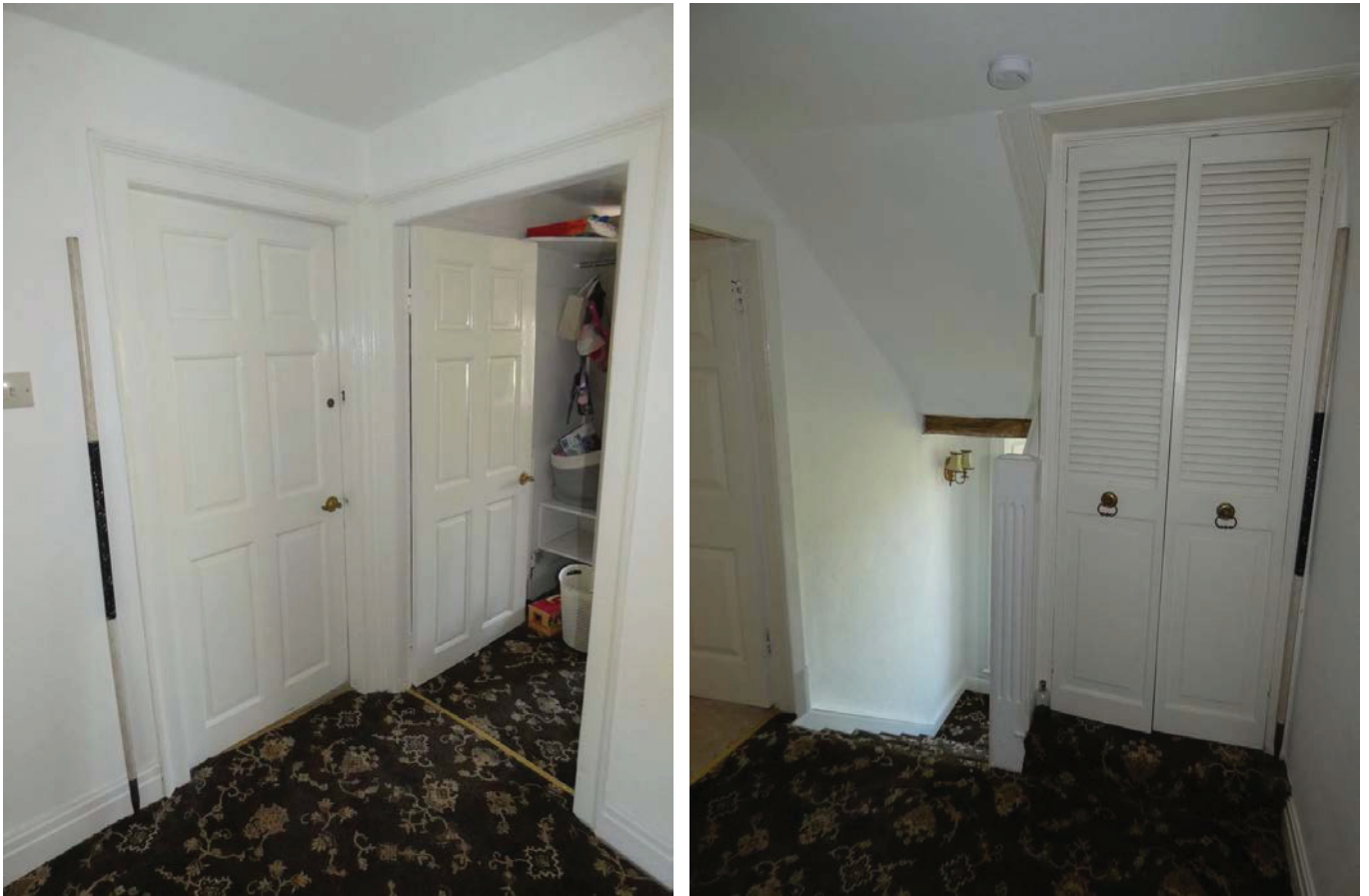
Plate 69 (left): Doors to the north and east in Room G2, viewed from the south-west
