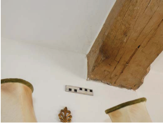
Plate 54 (left): Detail of a chamfered beam in Room G5, viewed from the south-west
