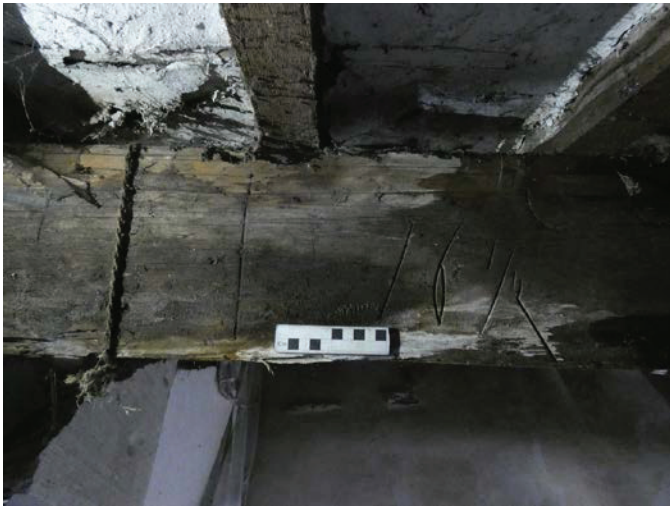
Plate 51 (left): Baltic timber marks in the roof of Room S1, viewed from the north-west
