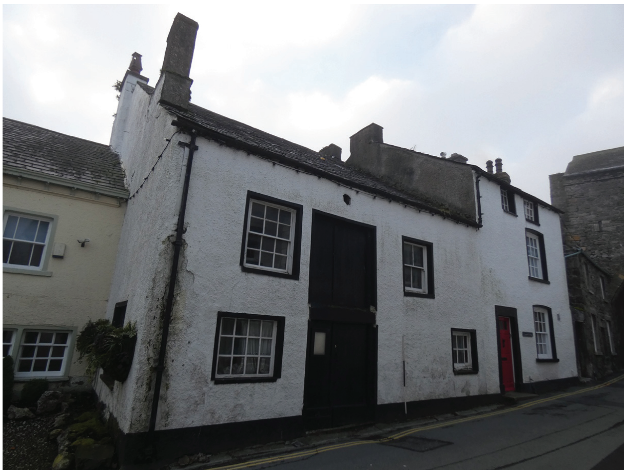
Plate 10: The north-west external elevation, viewed from the north
