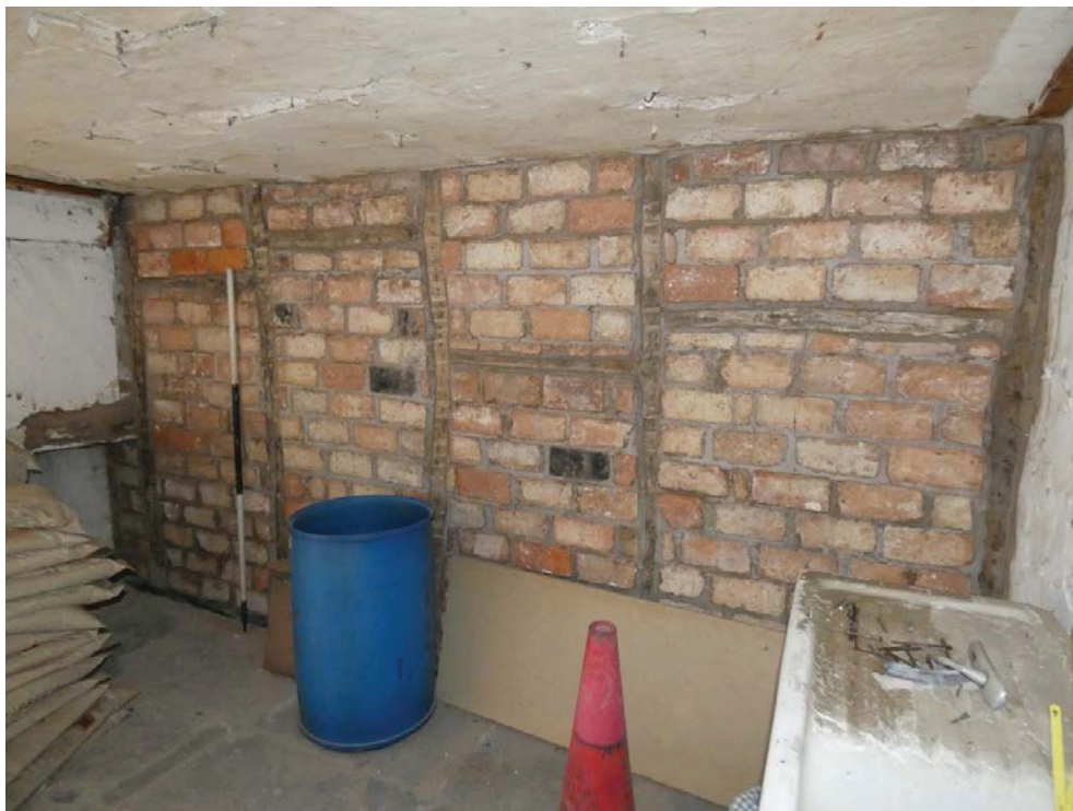
Plate 31: The south-west elevation in Room G2, viewed from the north-east
