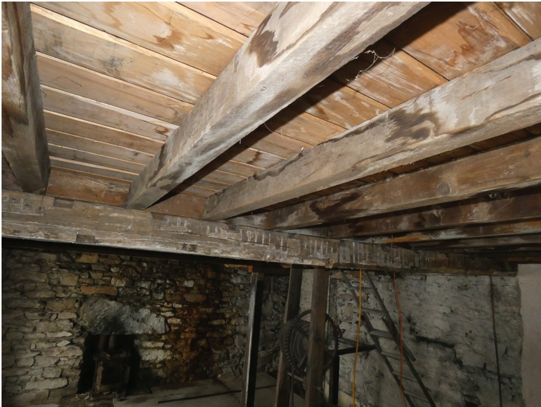
Plate 34: The central beam in Room F1, showing slots, viewed from the south-west
