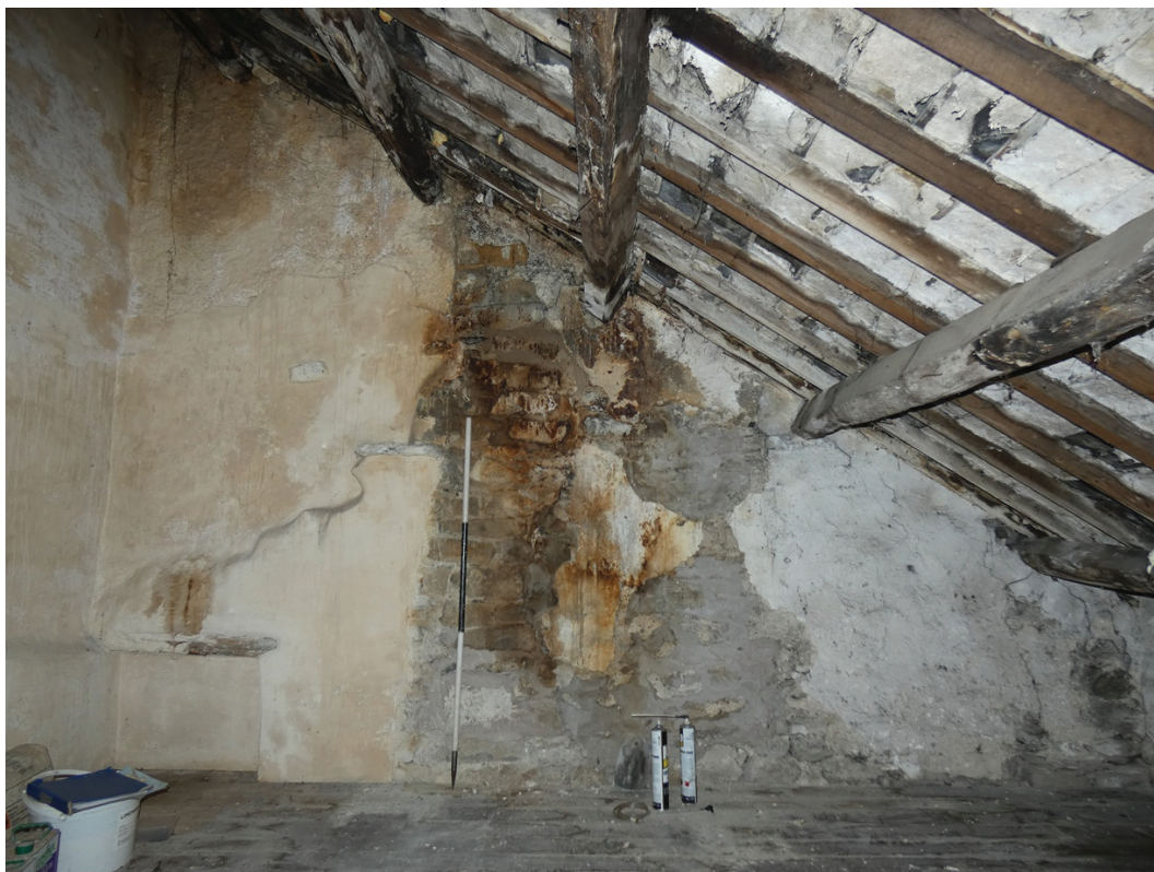
Plate 57: The south-west elevation of Room S1, viewed from the north-east
