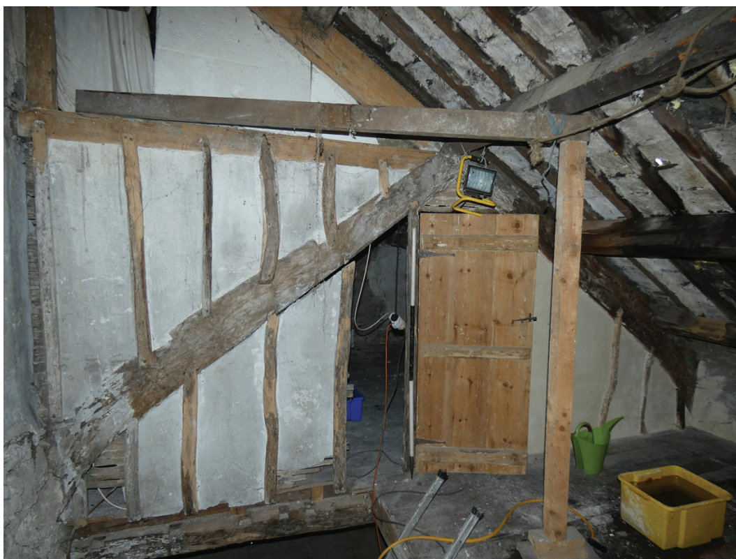
Plate 64: The south-west elevation, Room S2, viewed from the north-east
