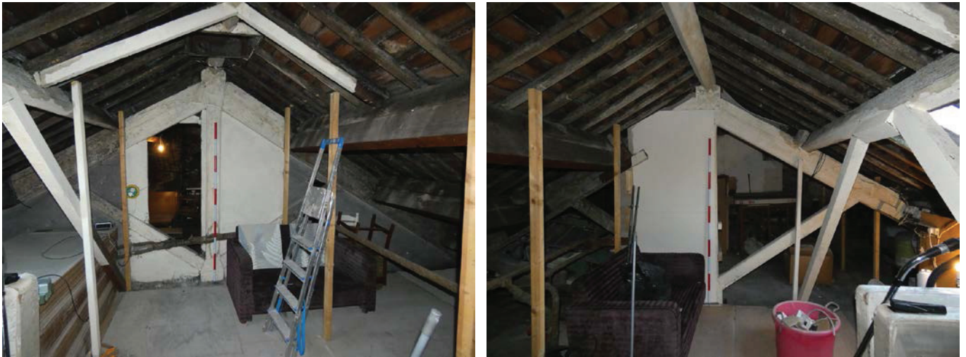
Plate 38 (left): The eastern truss, viewed from the west
