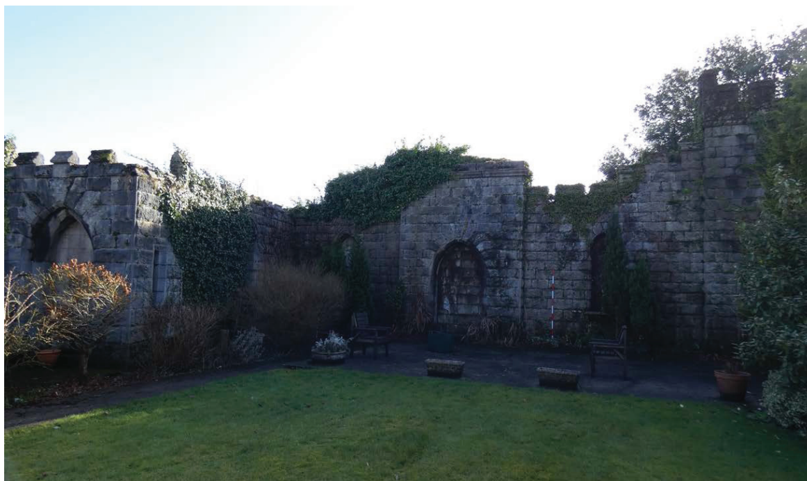
Plate 12: The folly in the garden to the south of the house, viewed from the north
