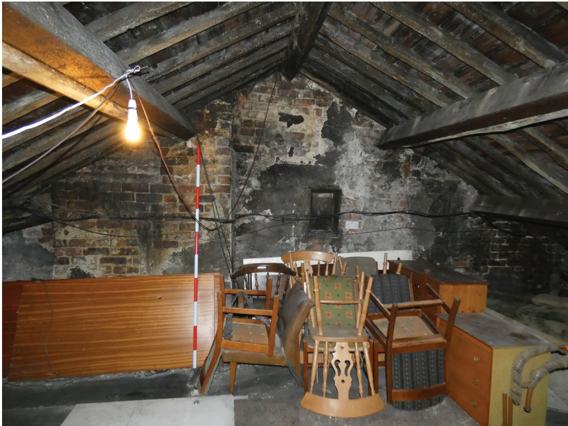
Plate 40: The east elevation within the attic, viewed from the west
