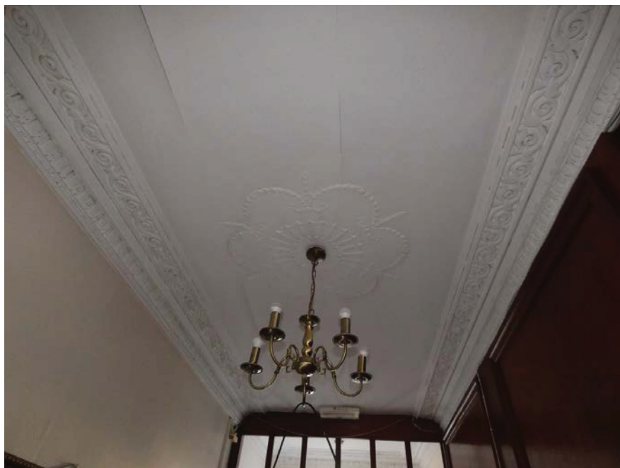
Plate 19: The plaster ceiling in the entrance hall, viewed from the south
