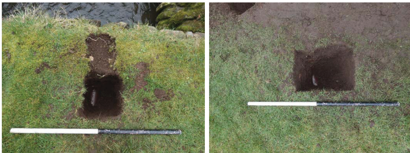
Plate 8 (left): Drainage Pit 1 excavated, showing the pipe, viewed from the west
