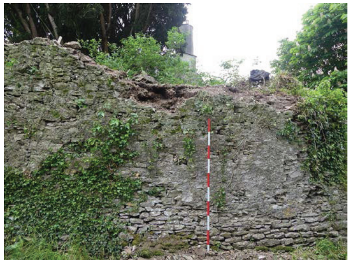
Plate 21 (left): The junction of the main wall ( 1001 ) and lower northern section ( 1002 ) showing the different fabrics
