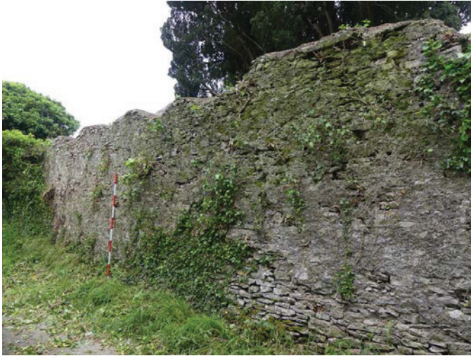
Plate 13 (left): The undulating parapet along the main part of the wall following the removal of the ivy, viewed from the north-east
