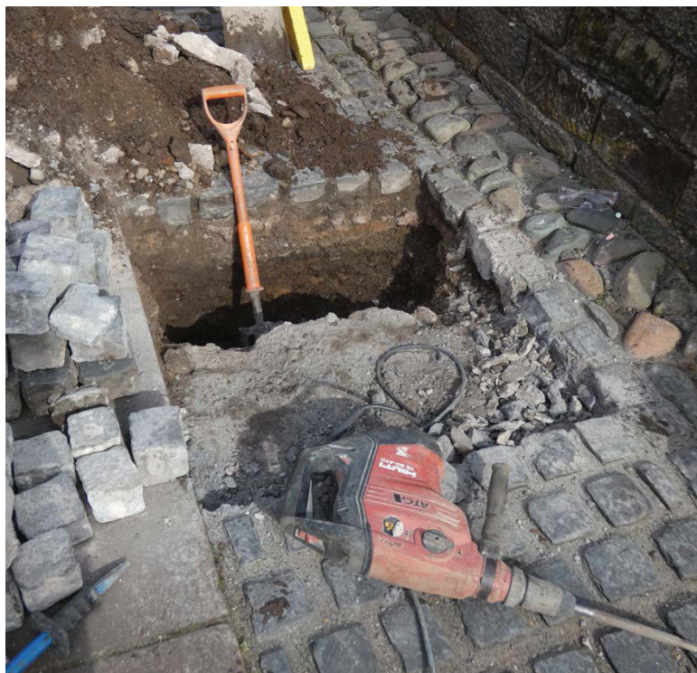
Plate 3 (left): Removal of the sett paving
