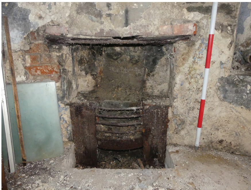
Plate 24: Detail of the fireplace on the north-west side of the ground floor room, viewed from the south-east
