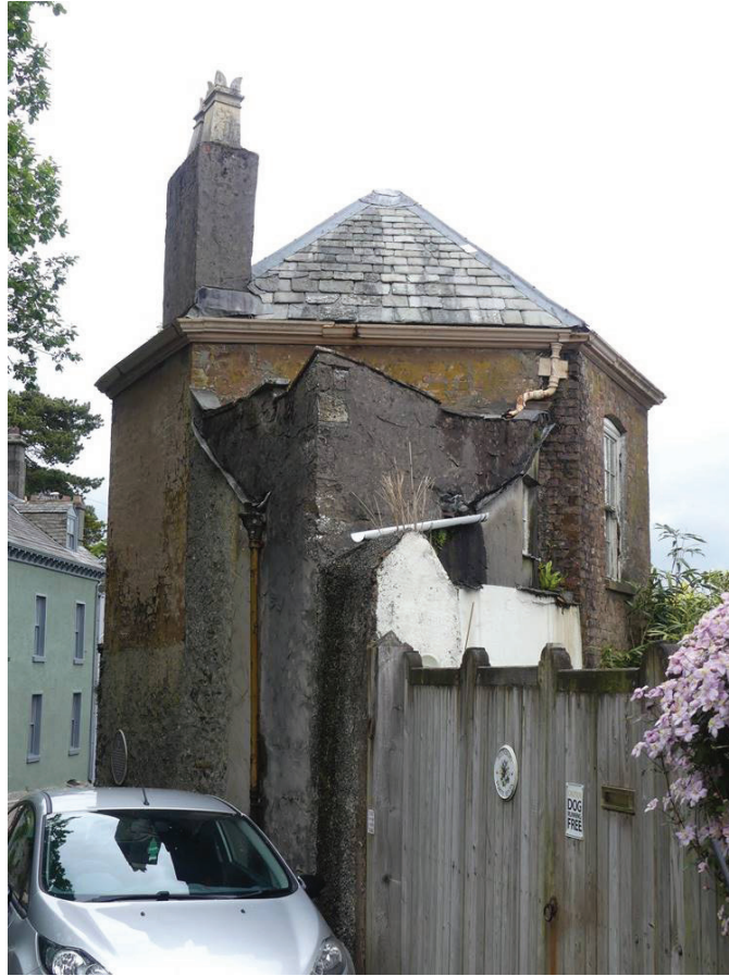
Plate 11: The south-west side of the building, viewed from the south-west
