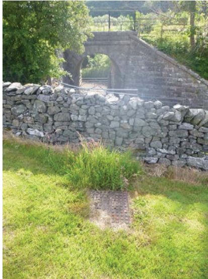
Plate 14: Manhole on the east side of the south-eastern field, viewed from the west
