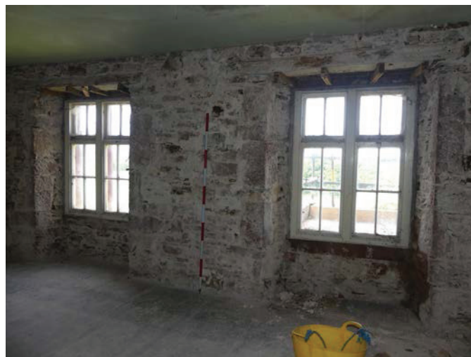
Plate 87: The north-west elevation, Room G7, viewed from the east
