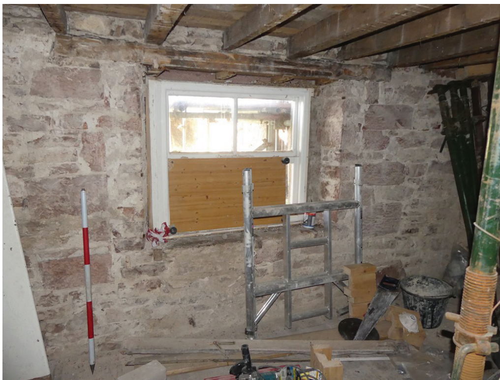
Plate 47: Window in the south-west elevation, Room G6b, viewed from the north-east
