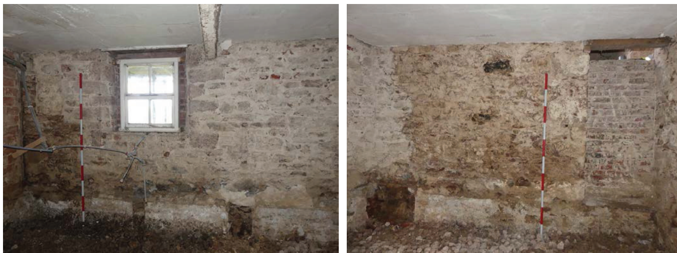
Plate 29 (left): The south-west elevation, Room G3, viewed from the north-east
