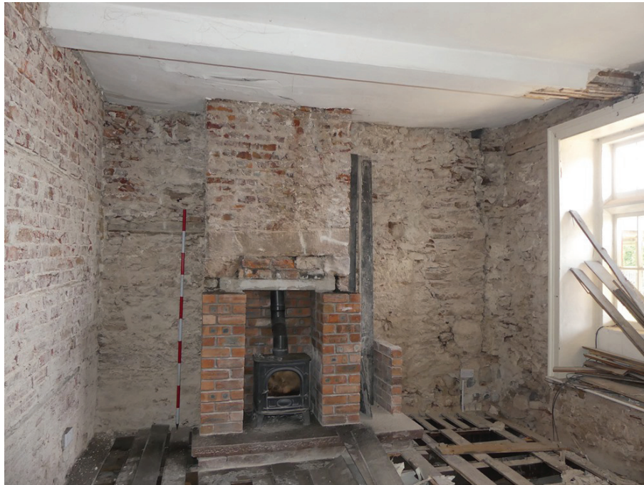
Plate 40: The north-west elevation in Room G5, viewed from the south-east
