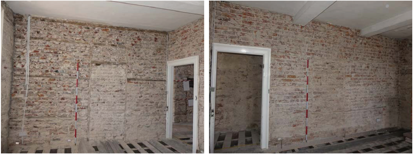
Plate 38 (left): The south-east elevation in Room G5, viewed from the north-west
