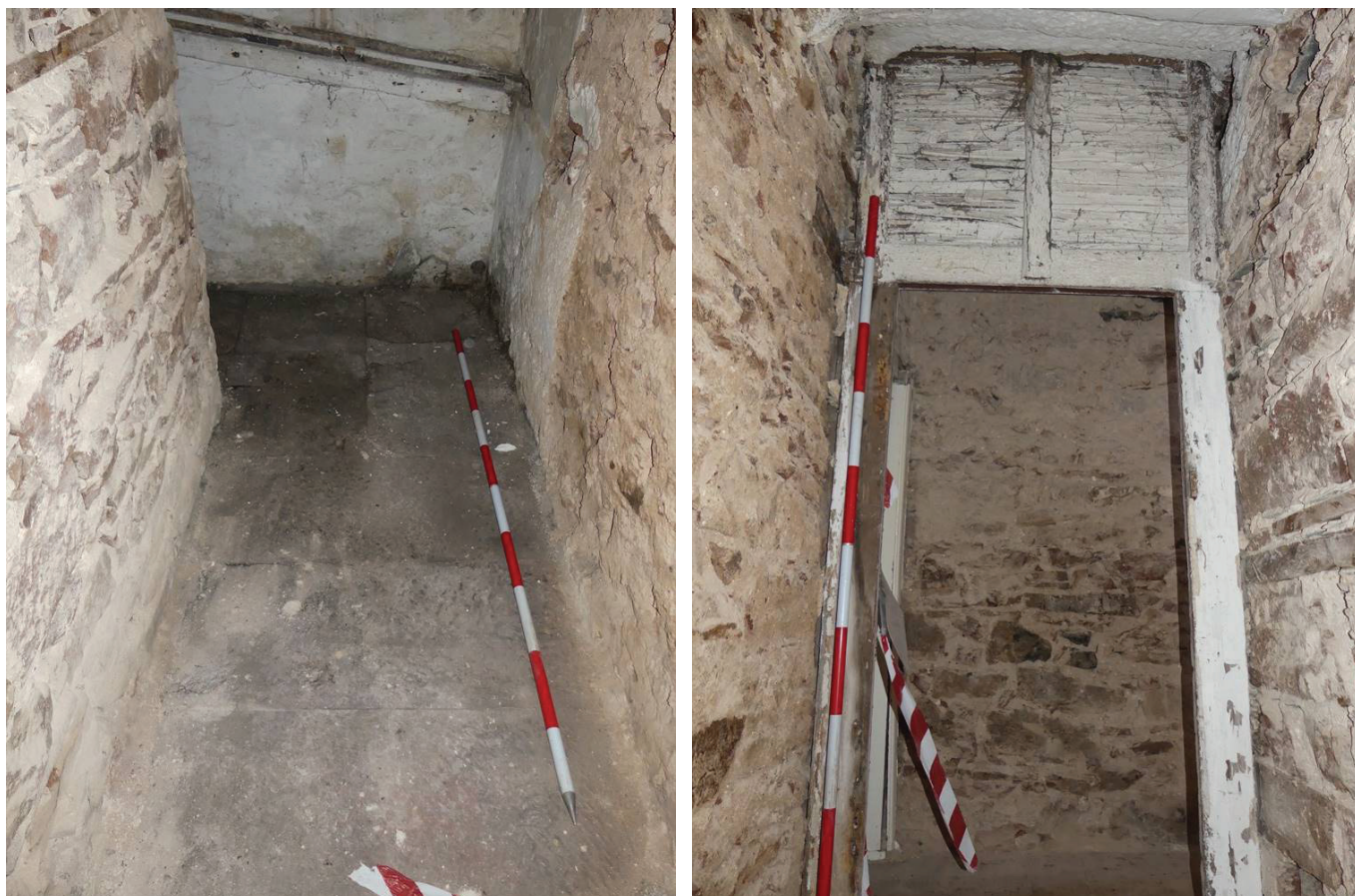
Plate 41 (left): Sandstone flag floor in Room G6a, viewed from the north-east
