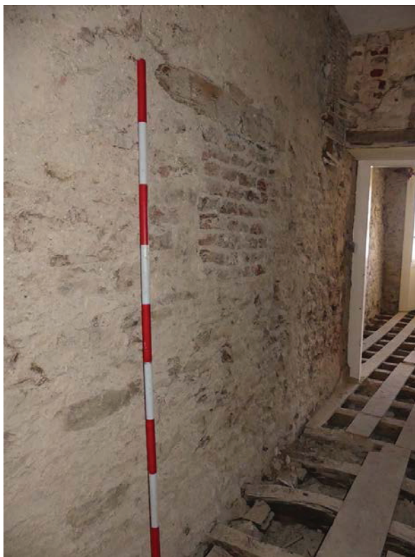
Plate 35: The blocked window in the south-west elevation of Room G4, viewed from the east
