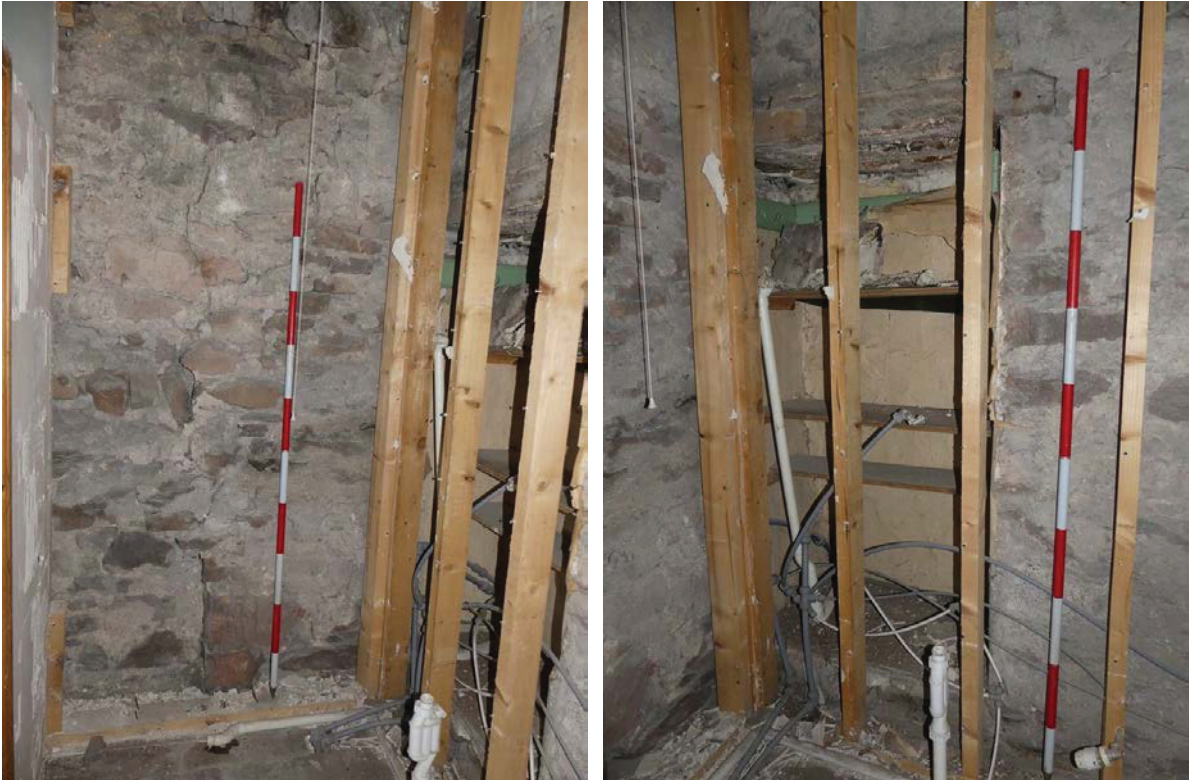
Plate 62 (left): Butt joint on the south-west side of the south-east elevation, Room F1, viewed from the north-west
