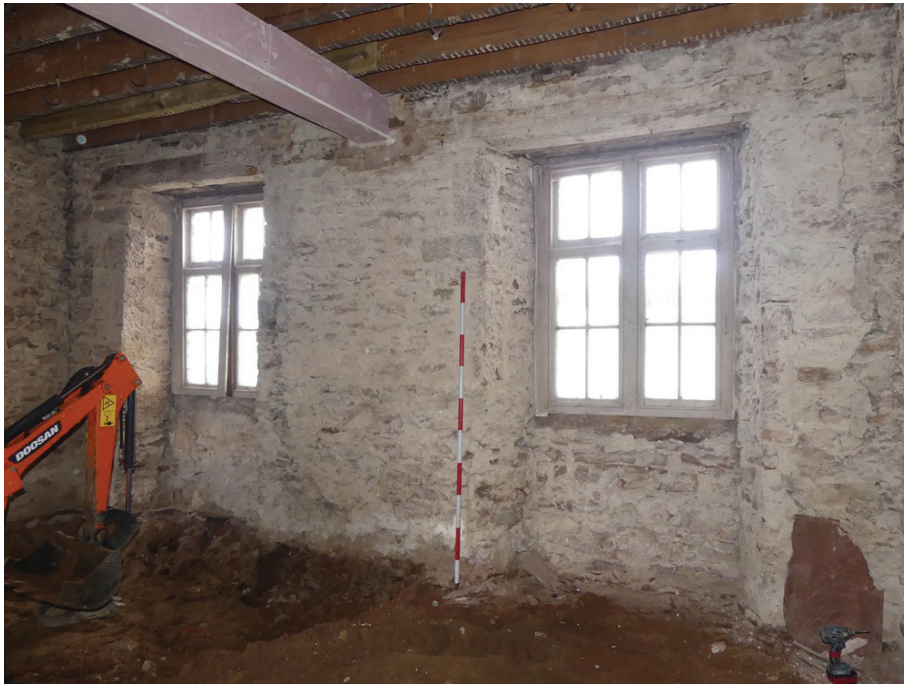
Plate 57: The north-west elevation in Room G8, viewed from the east
