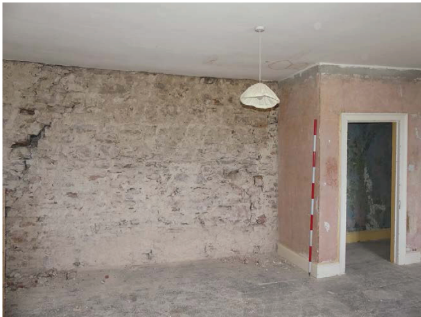
Plate 80: The south-east elevation, Room F6, viewed from the north-west
