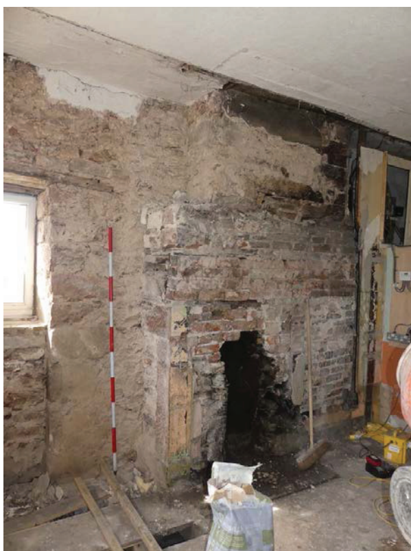
Plate 19 (left): Chimney breast and fireplace in the south-east elevation, Room G1, viewed from the north
