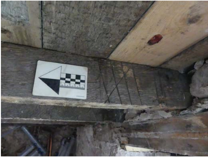
Plate 43 (left): Baltic timber marks in the ceiling of Room G6b, viewed from the north-west
