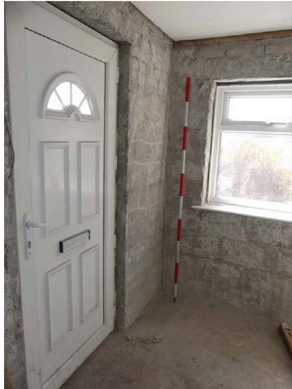
Plate 26: General view of Room G2, from the north-west
