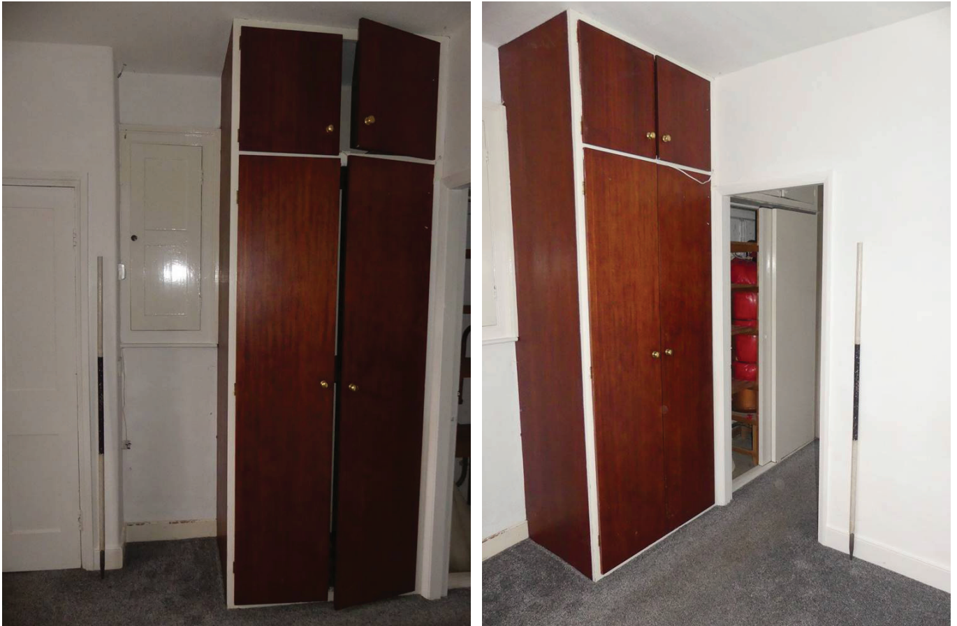
Plate 33 (left): West side of the south elevation of G2
