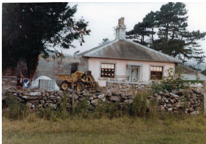
Plate 12: The east elevation of Greenfield Lodge during the rebuilding of c1984
