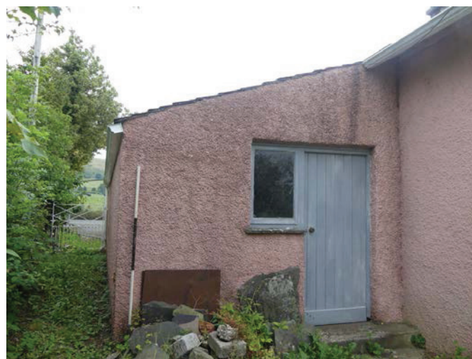
Plate 26: Garage to the north end of the west external elevation
