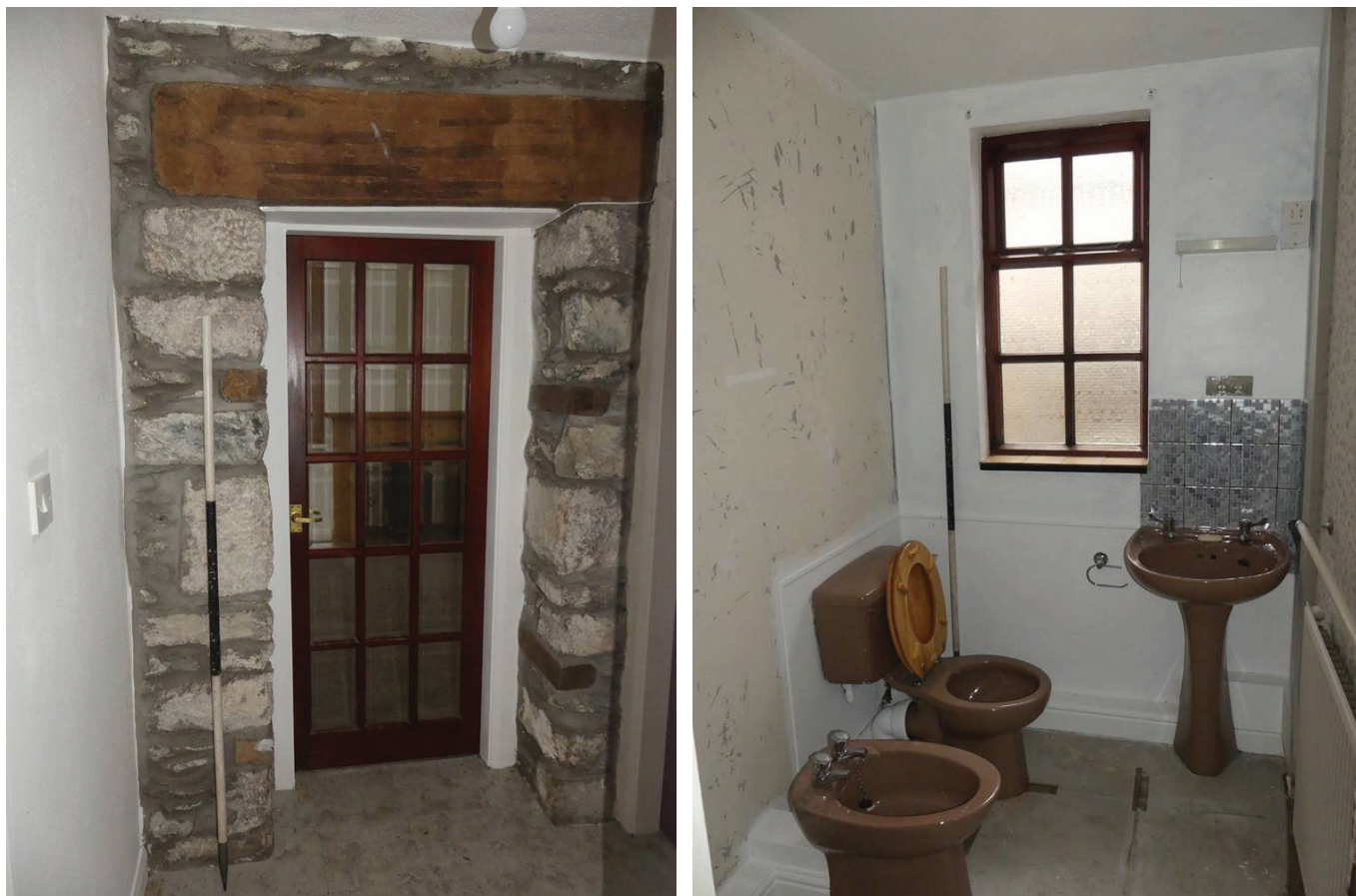
Plate 55 (left): Doorway in the north elevation of G9
