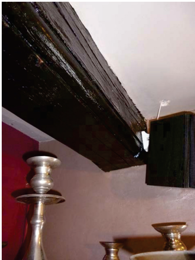
Plate 29 (left): Ovolo-moulded chamfer in Room G1
