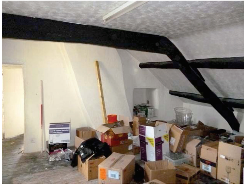
Plate 49: South elevation and west end of south truss, Room S1
