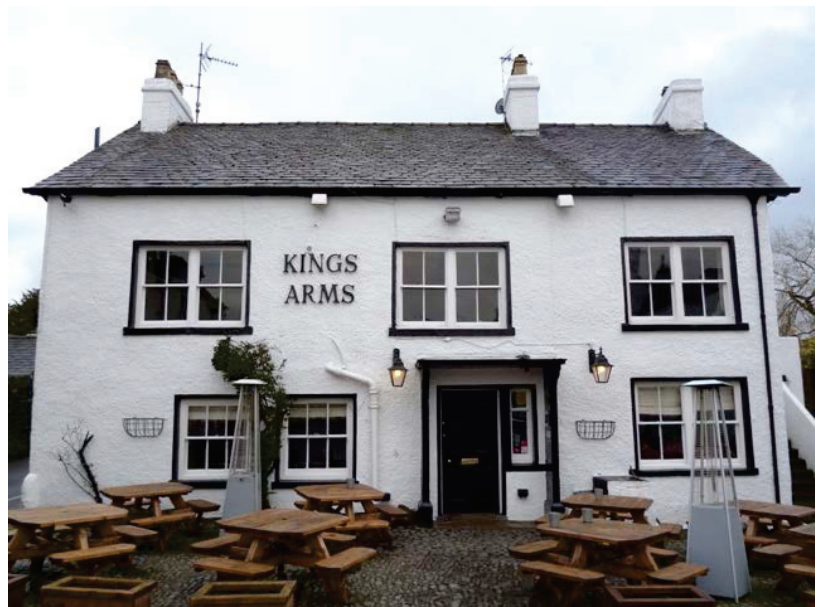
Plate 25 (left): North external elevation
