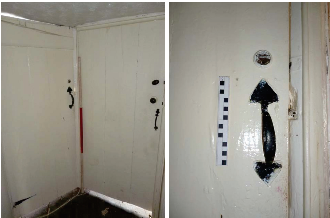
Plate 50 (left): Early doors on the north side of Room S2
