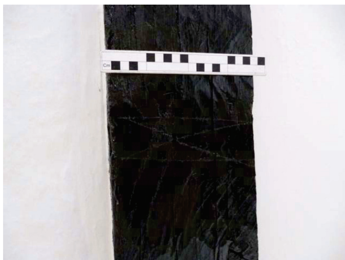
Plate 35 (left): Levelling mark on the beam in Room F4
