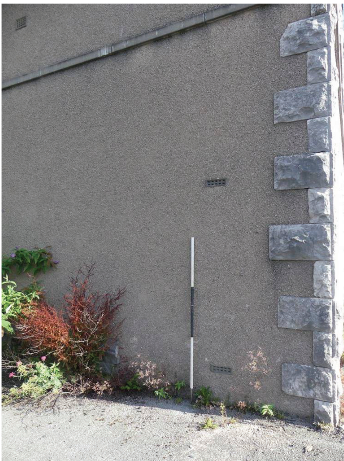
Plate 46 (left): The gap in the plinth in the return of the south-east external elevation of the courthouse, viewed from the south-west
