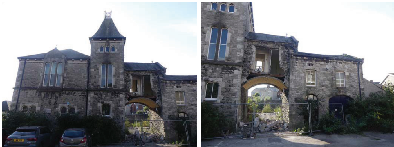
Plate 37 (left): The north-east side of the north-west external elevation of the courthouse, viewed from the north-west
