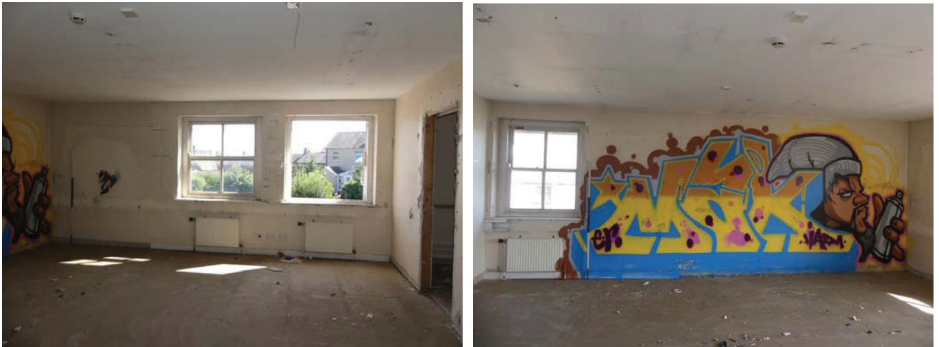
Plate 136 (left): The south-east elevation of Room F1 of the courthouse, viewed from the north-west
