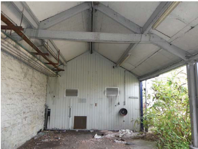
Plate 50 (left): Example of a truss in the centre of the open-fronted building extending from the south-east side of the courthouse, viewed from the south-east
