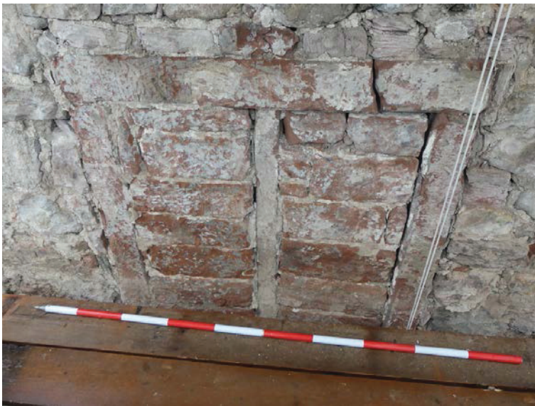
Plate 21 (left): Blocked mullion window in the centre of the south-east elevation, viewed from the south-east
