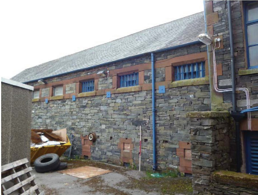
Plate 40: High-level windows in the cells at Millom police station (after Greenlane Archaeology 2013)
