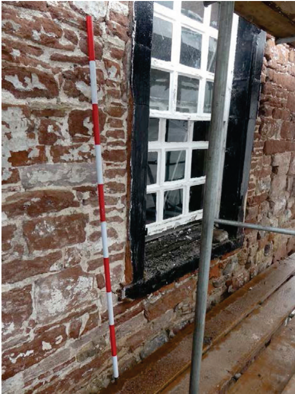
Plate 23 (left): First floor window on the south-east side of the south-west elevation showing rebuild around the jambs, viewed from the west
