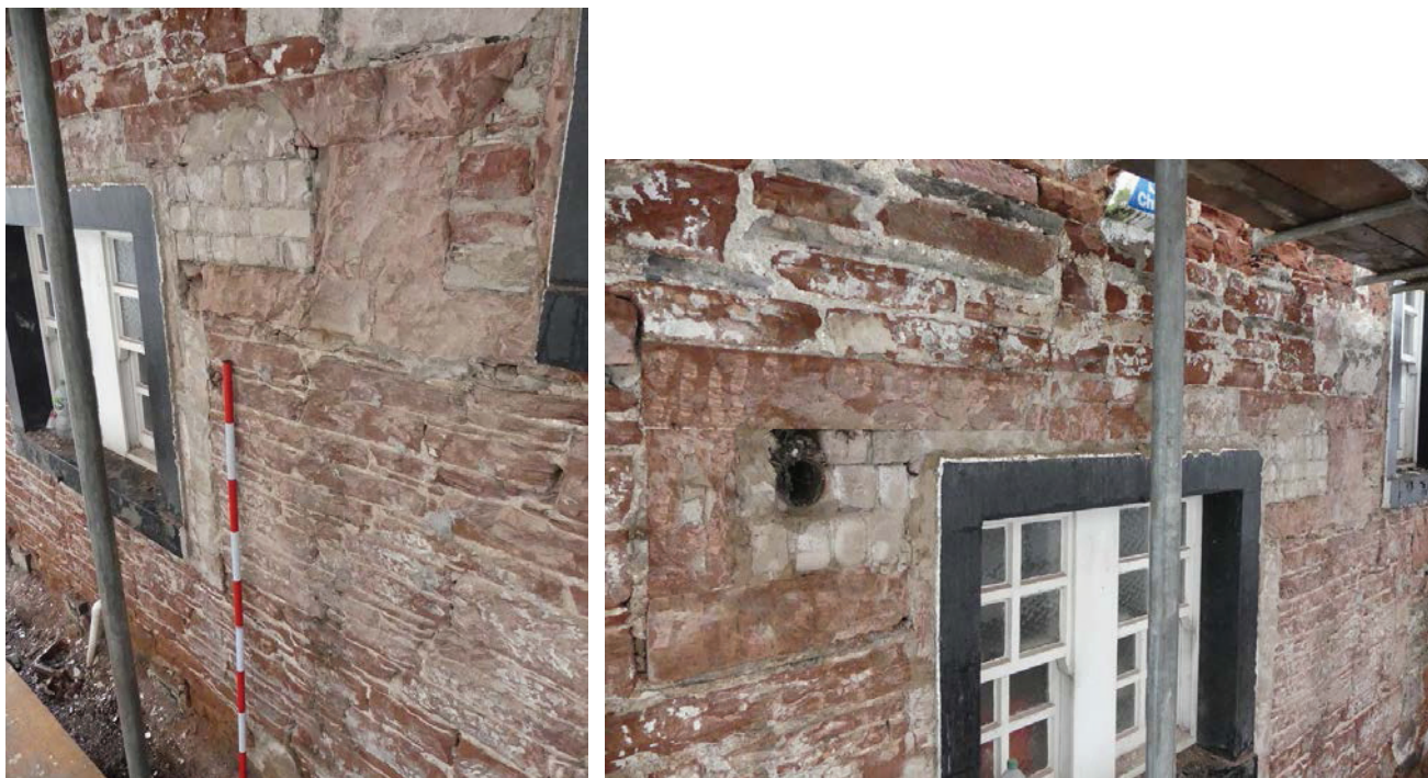
Plate 38 (left): Blocked apertures at the north-west end of the ground floor of the south-west elevation, viewed from the south
