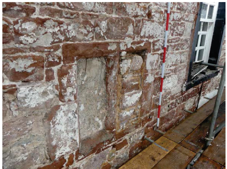
Plate 25 (left): V-jointed quins on the north-west side of the south-east elevation, viewed from the south
