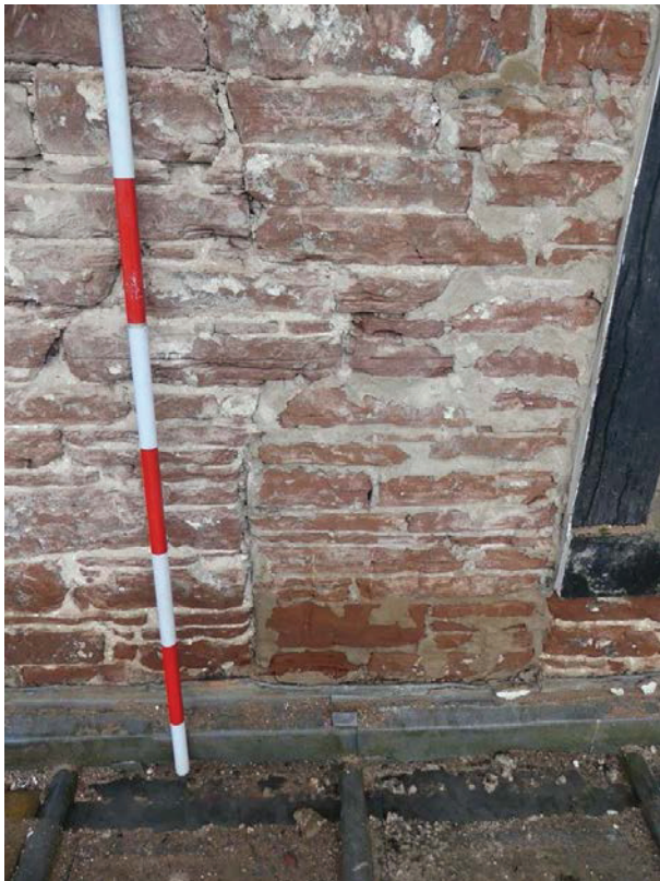
Plate 3 (left): Butt joint between the two first floor windows in the north-west elevation, viewed from the north-west
