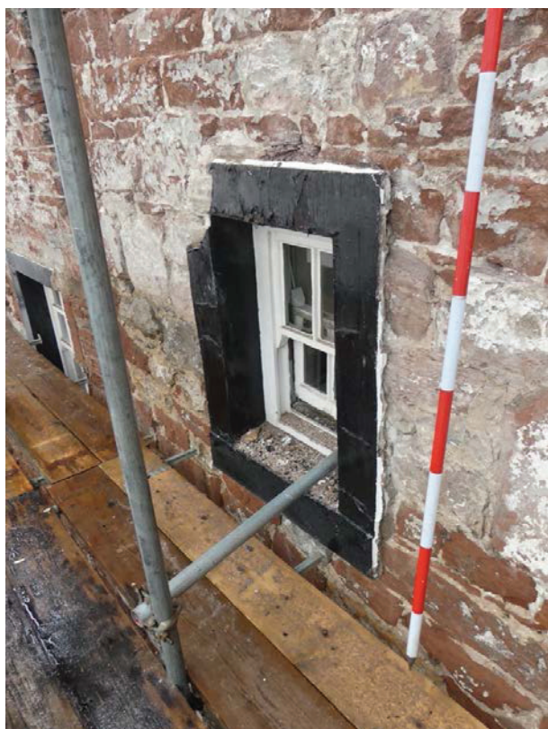
Plate 28 (left): First floor window with concrete band in the south-west elevation, viewed from the south
