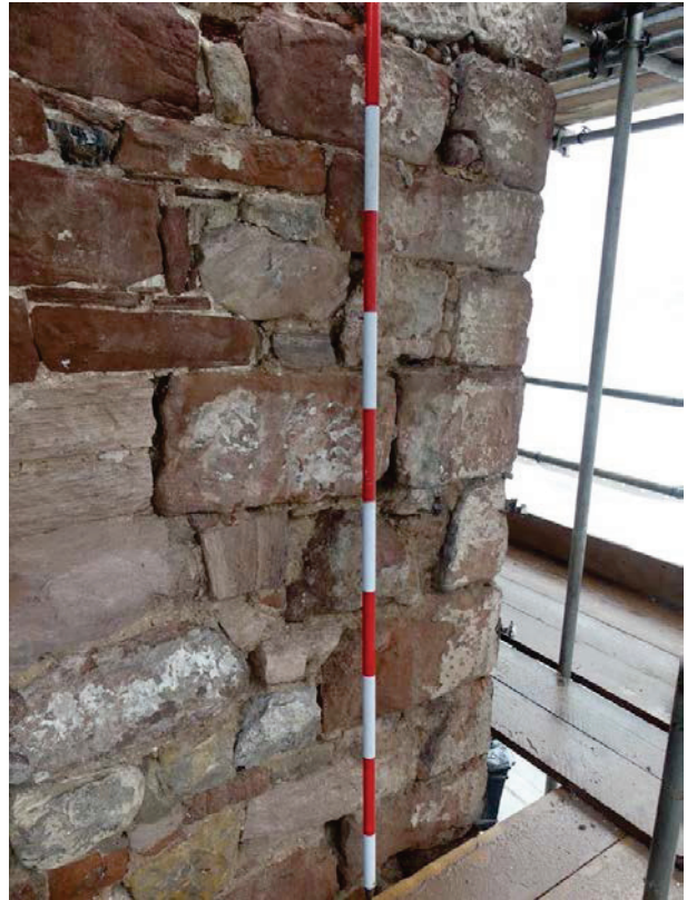
Plate 23 (left): First floor window on the south-east side of the south-west elevation showing rebuild around the jambs, viewed from the west
