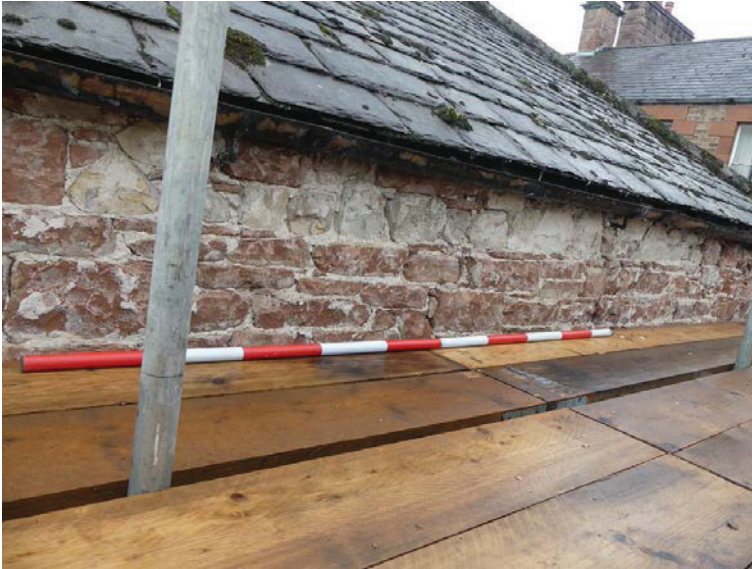
Plate 1 (left): Different build at the top of the north-west elevation, viewed from the north
