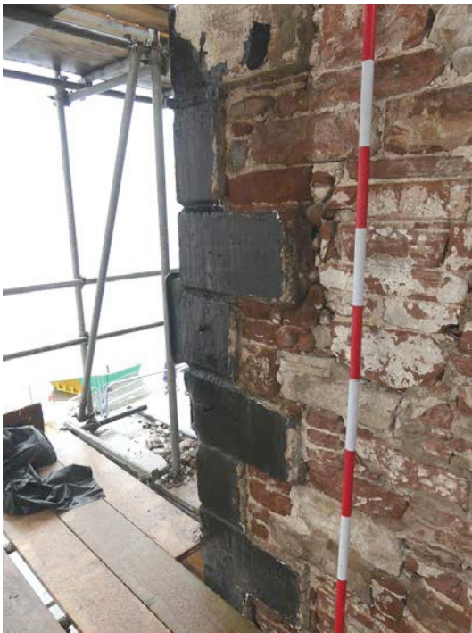
Plate 25 (left): V-jointed quins on the north-west side of the south-east elevation, viewed from the south
