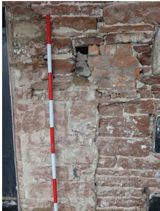
Plate 3 (left): Butt joint between the two first floor windows in the north-west elevation, viewed from the north-west
