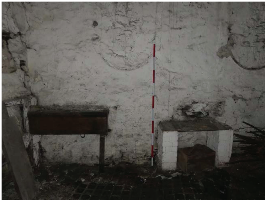
Plate 42 (left): Detail of scar from feed holders and brick base against south-east elevation of Room G2
