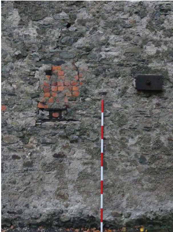
Plate 22 (left): Brick section, iron I-beam end and tie rod plate in the south-west end of the south-east external elevation, viewed from the south-east
