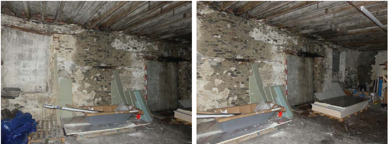
Plate 32 (left): South-east end of the south-west elevation of Room G1
