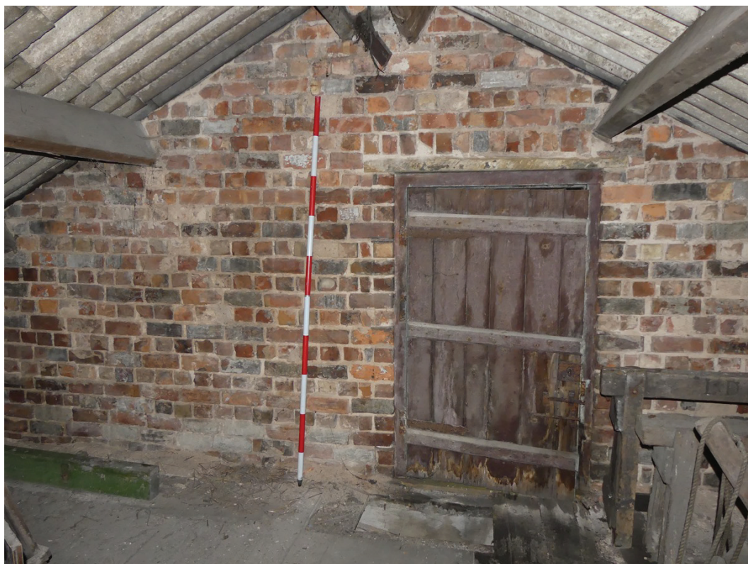
Plate 55 (left): North-west elevation of Room F1
