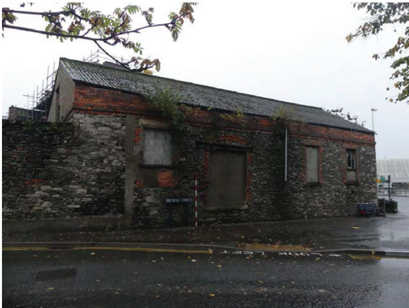
Plate 10: General view of the south-west external elevation, from the south-west
