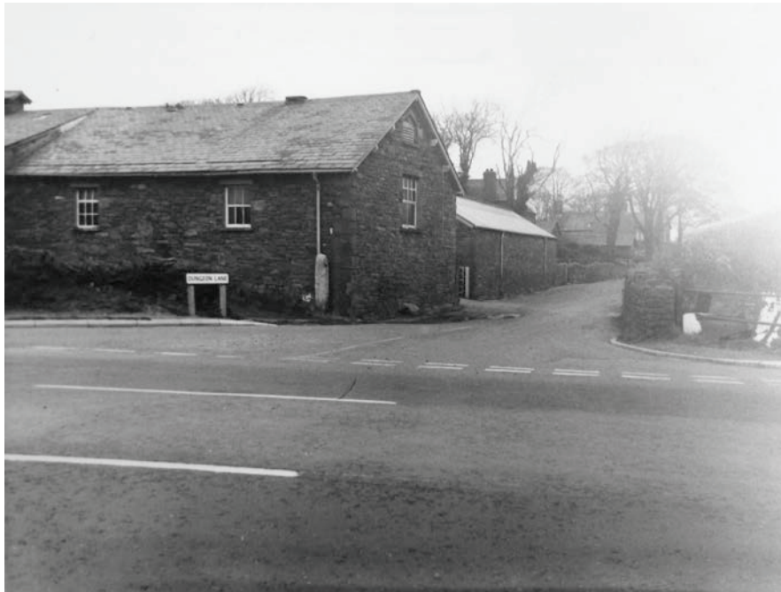
Plate 8: The farm buildings (Buildings 3 and 4) at the junction of Rampside Road and Dungeon Lane in 1973 (CAC(B) BLC/265/VBROO22)
