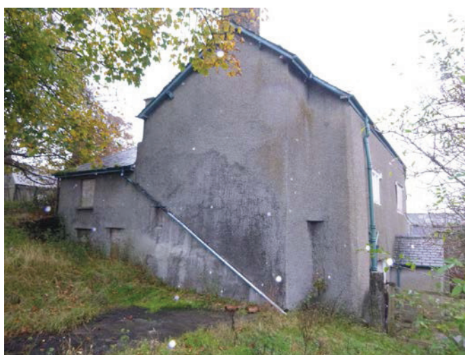
Plate 17: West elevation of the farmhouse, viewed from the west
