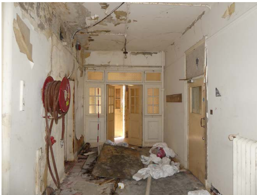
Plate 49: General view of the east end of Room G5, from the west
