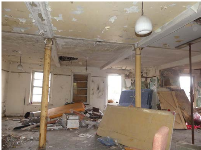
Plate 40 (left): Beams and columns between Rooms G3 and G4 exposed following the soft strip, viewed from the west
