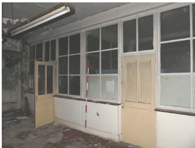
Plate 39: North elevation of Room G2, viewed from the south-east
