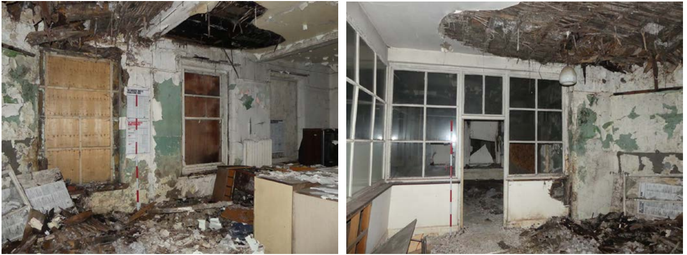
Plate 44 (left): The west elevation of Room G4, viewed from the south-east
