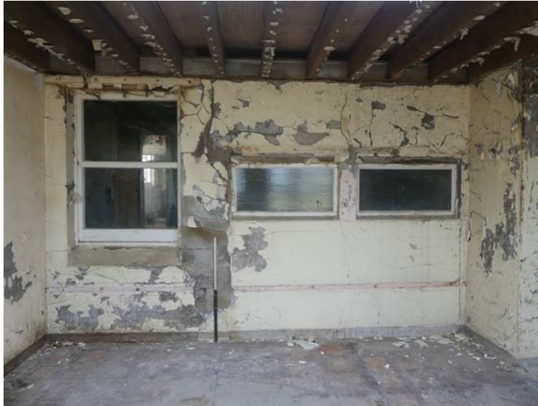
Plate 96: The south elevation of Room F12, viewed from the north
