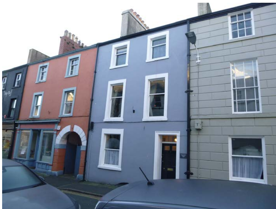
Plate 9: General view of the building and adjoining property to the east, from the north
