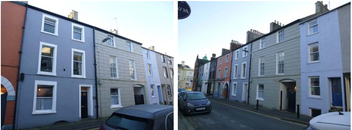
Plate 7 (left): The north elevation, viewed from the north-east
