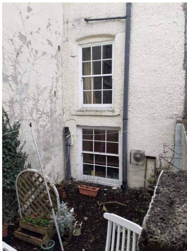
Plate 10: The south external elevation, viewed from the south-east
