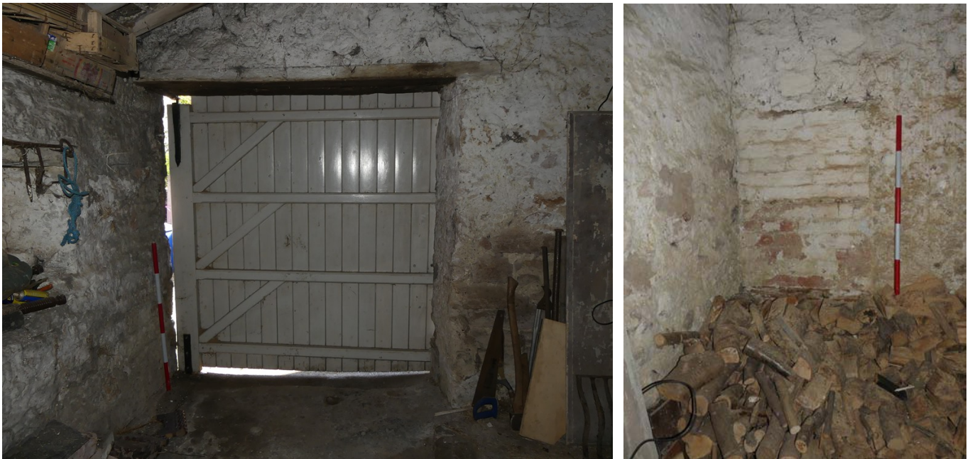
Plate 48 (left): Wagon door in the east elevation of Room G4
