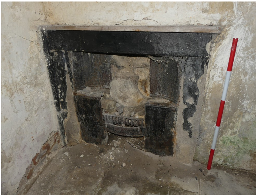
Plate 41 (left): Fireplace in Room G3
