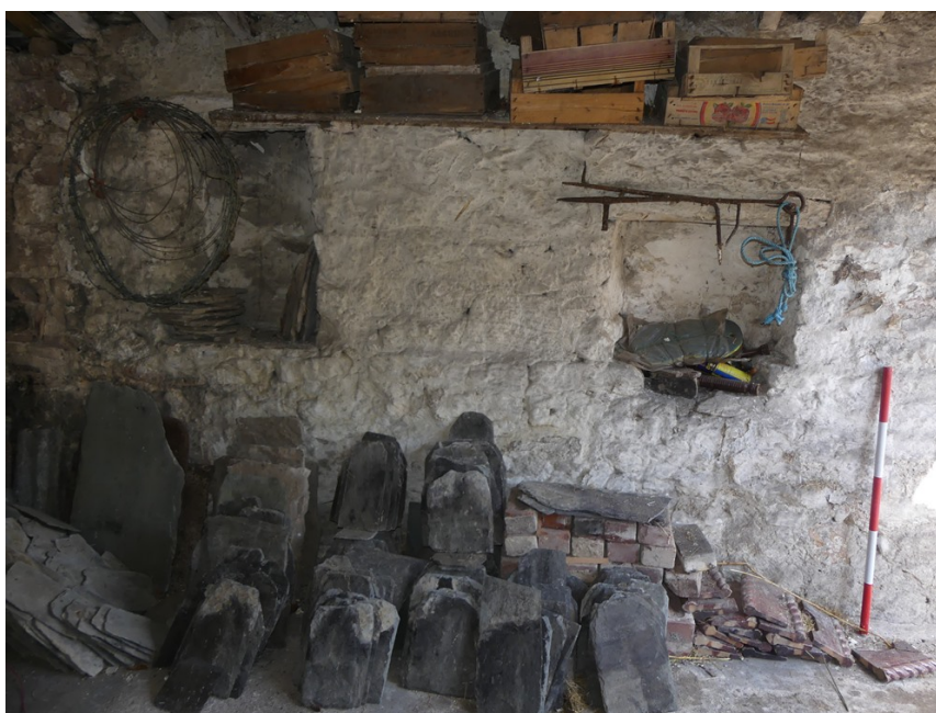
Plate 45: General view of the north elevation of Room G4
