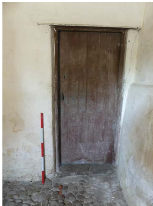
Plate 35: Doorway in the west elevation of Room G2
