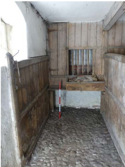
Plate 25 (left): Cobbled floor and brick channel in Room G2
