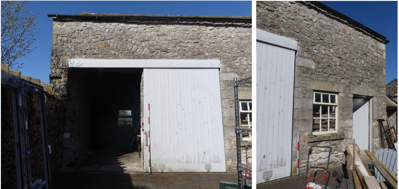
Plate 6 (left): Doorway at the south end of the east external elevation
