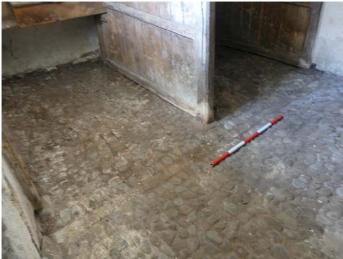
Plate 25 (left): Cobbled floor and brick channel in Room G2
