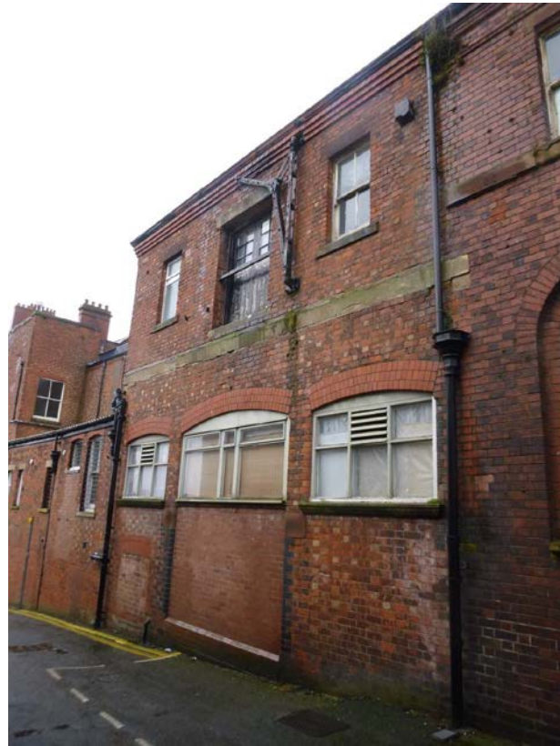
Plate 34: Detail of the blocked doorway and first floor loading doorway in the east external elevation
