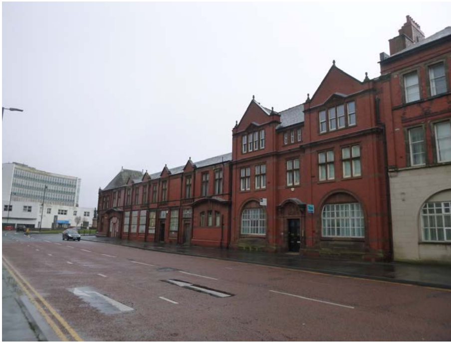
Plate 27: General view of the west external elevation
