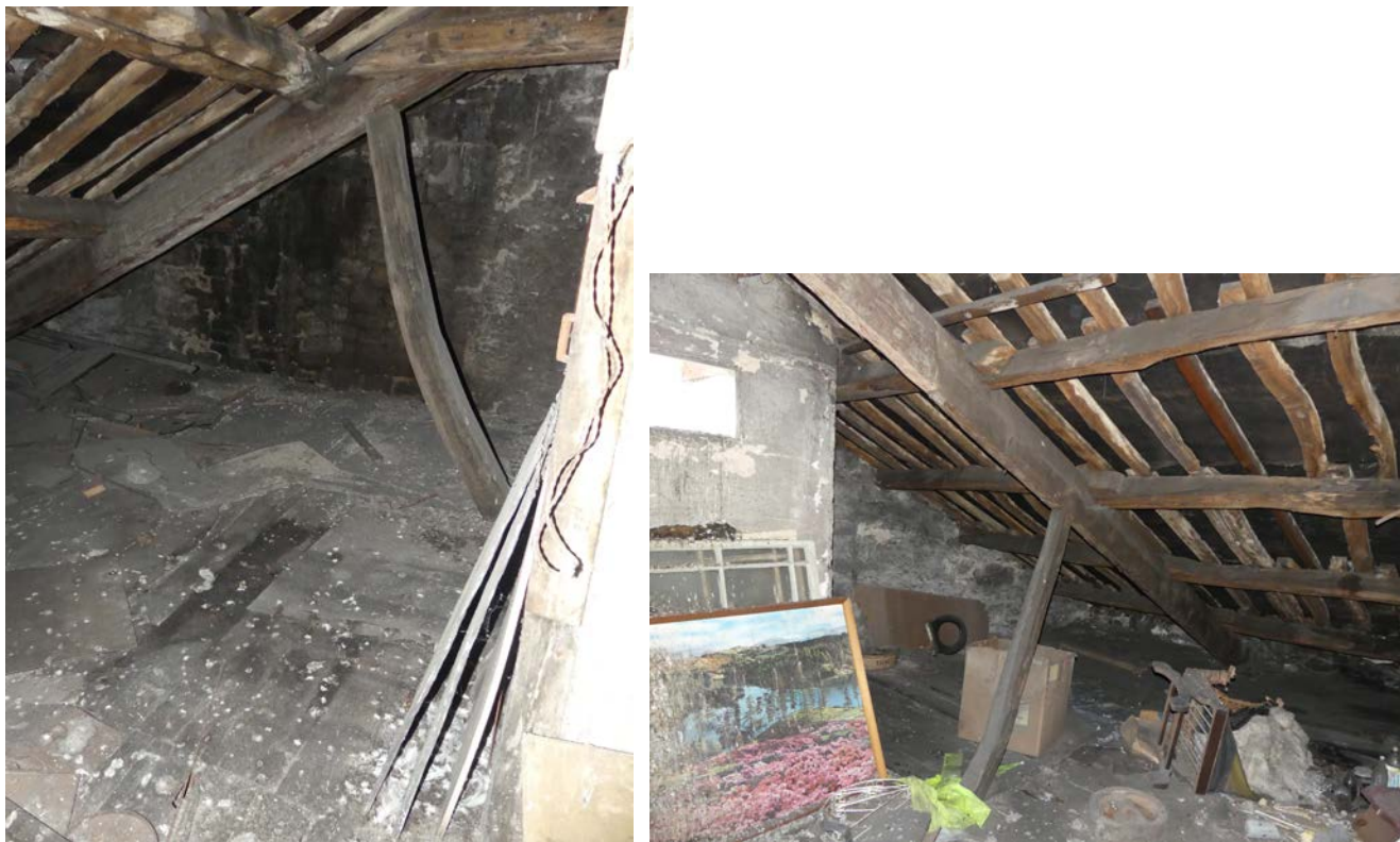
Plate 38 (left): Truss in the attic
