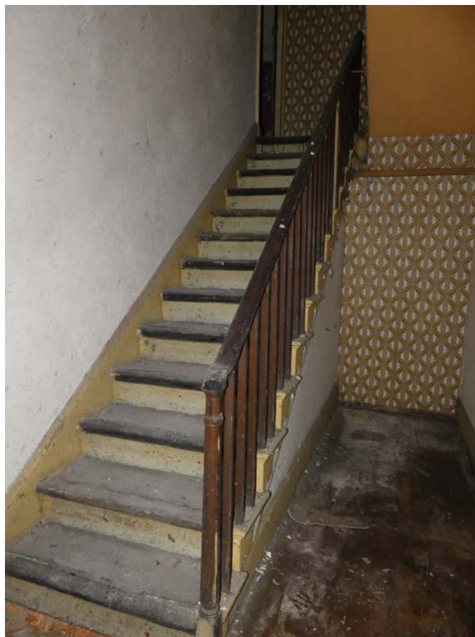
Plate 29: Staircase on the south side of the ground floor
