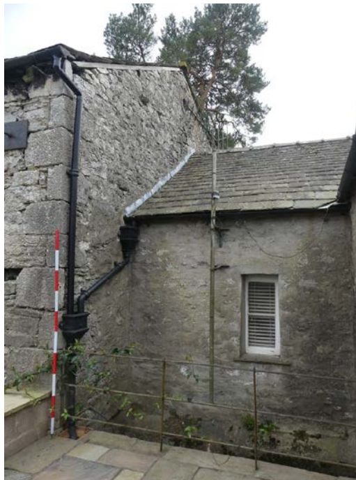
Plate 13: The north-west external elevation, viewed from the east
