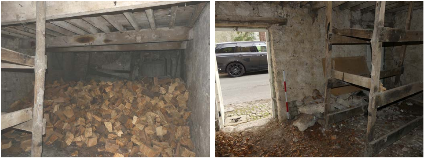
Plate 20 (left): General view of Room LF2 from the south-west
