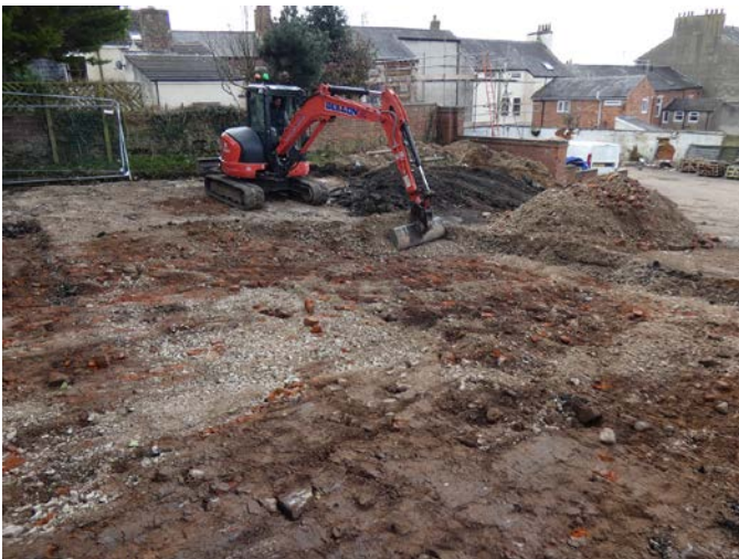
Plate 9 (left): Removal of tarmac ( 100 ) revealing demolition rubble ( 102 )
