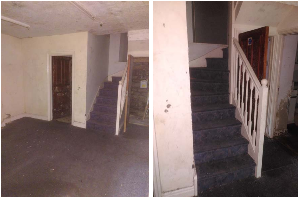
Plate 21 (left): General view of the main ground floor room of the house, viewed from the south-east
