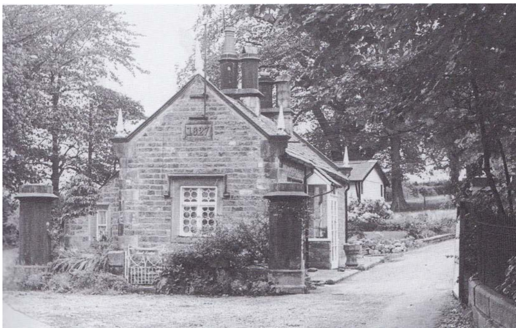
Plate 8: Photograph of the site (from Martin 2004, 219)
