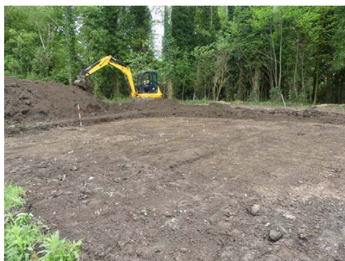
Plate 4 (left): Raised topsoil (1000) being removed along the east side of the site, viewed from the south-west
