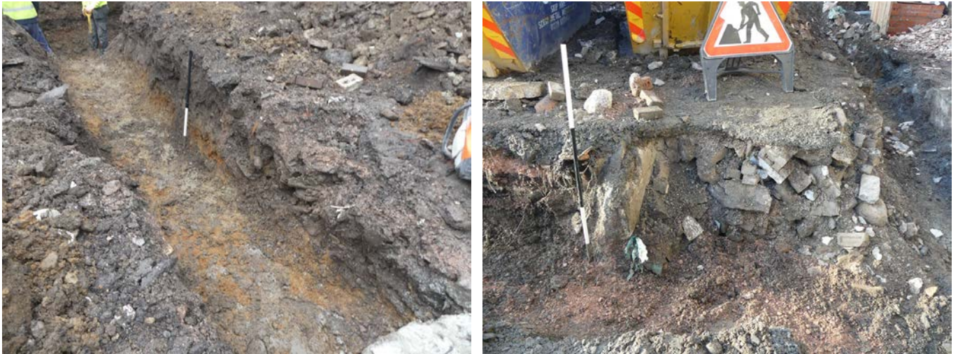
Plate 21 (left): Central foundation trench, viewed from the south
