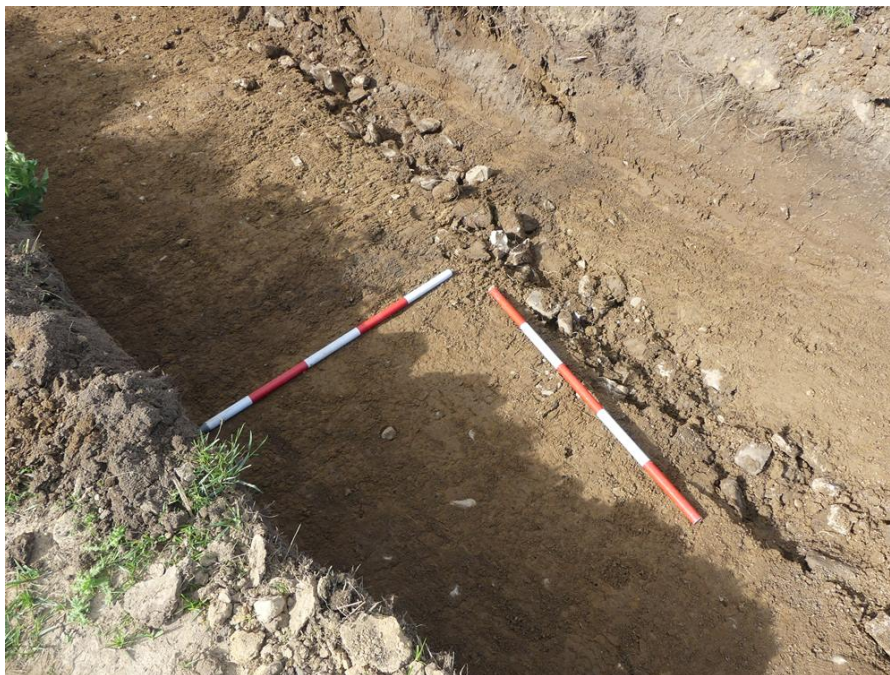
Plate 72: Drain 1003 cut by drain 1005, viewed from the south
