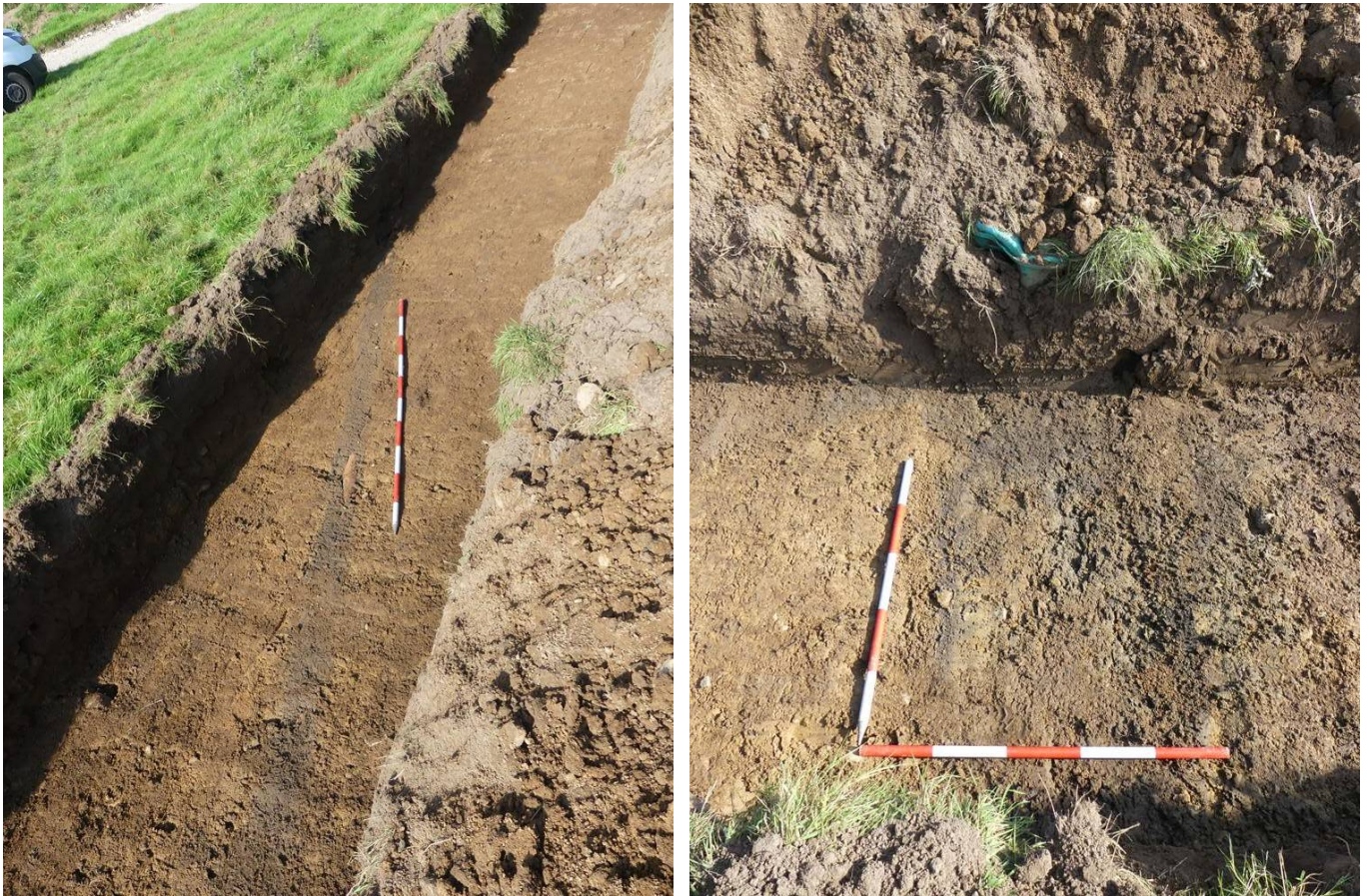
Plate 94 (left): Drain 1303 viewed from the east
