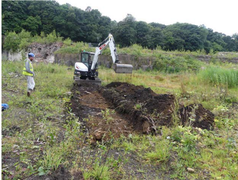
Plate 143: Working shot (Trench 3)
