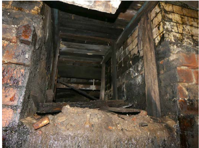
Plate 99 (left): Timber lined opening in the brick block in the north-east end room (lower floor) of the mill building, Area D
