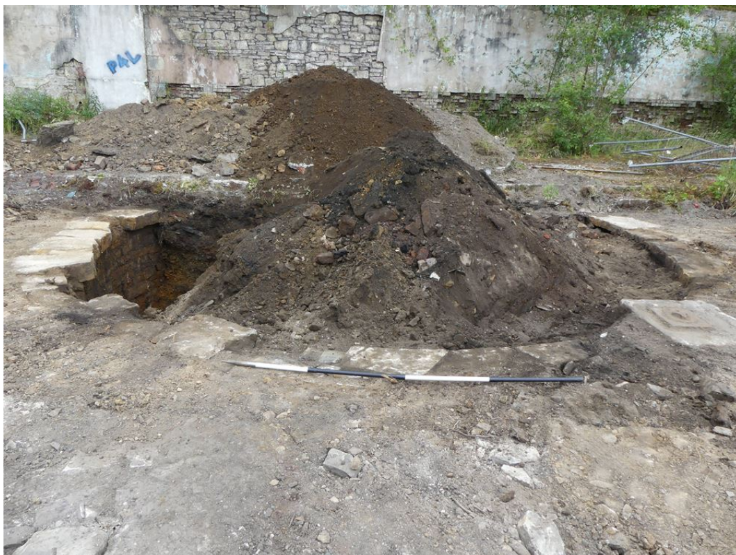
Plate 199: General view of 425 from the north-east
