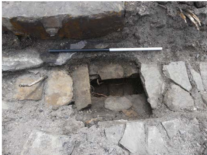
Plate 166: Capping stones removed from culvert 402, revealing the original structure 433
