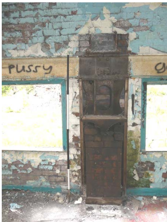
Plate 112 (left): North-east buttress on the north-west elevation of the north-east end room (upper floor) of the mill building, Area D
