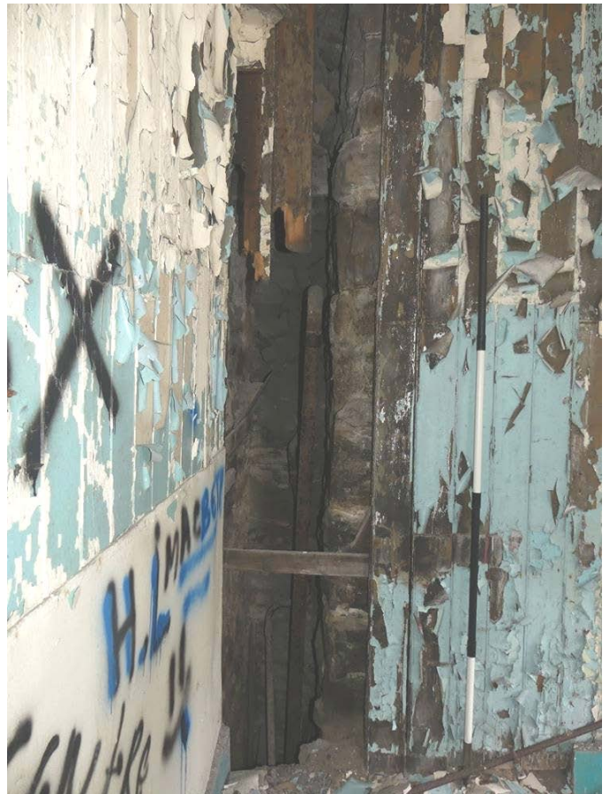
Plate 116 (left): Stud partition to the south-west end of the north-east end room (upper floor) of the mill building, Area D
