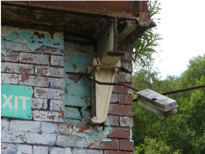
Plate 88 (left): Bracket and girder supporting a beam in the north-east external elevation of the mill building, Area D
