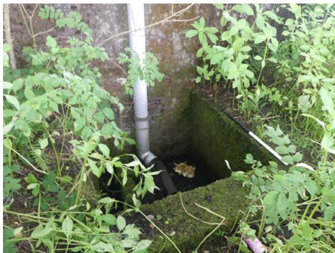
Plate 62: Pit to the north side of the east tank, Area B
