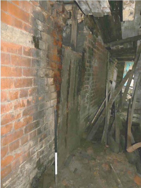
Plate 99 (left): Timber lined opening in the brick block in the north-east end room (lower floor) of the mill building, Area D
