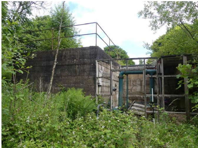
Plate 51 (left): Concrete tank and timber structure to the west of the central tank, Area B
