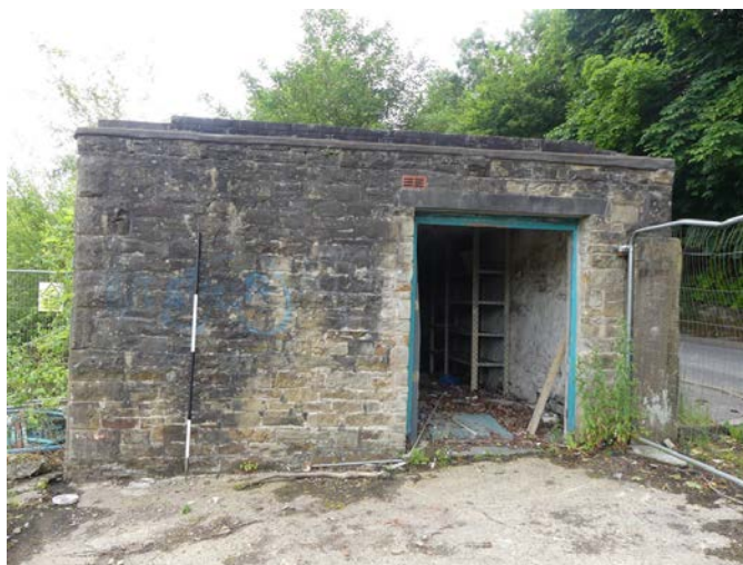
Plate 63: North-west external elevation of the substation, Area C
