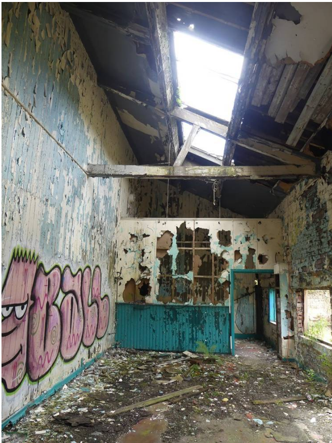
Plate 116 (left): Stud partition to the south-west end of the north-east end room (upper floor) of the mill building, Area D
