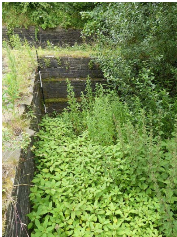
Plate 32: Plinth along the edge of one of the tanks in the west tank, Area B
