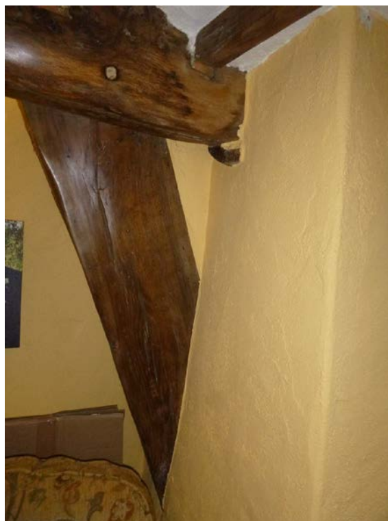
Plate 15 (left): The south-west end of the front (south-east) external elevation, viewed from the south Plate 16 (right): The base of the south-east cruck blade in the north-east part of the cottage, viewed from the south-west
