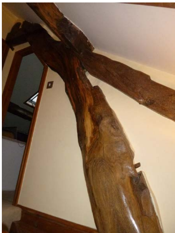
Plate 17 (left): The top of the north-west cruck blade in the north-east part of the cottage, viewed from the north Plate 18 (right): The collar of the cruck truss in the north-east part of the cottage, viewed from the north-east
