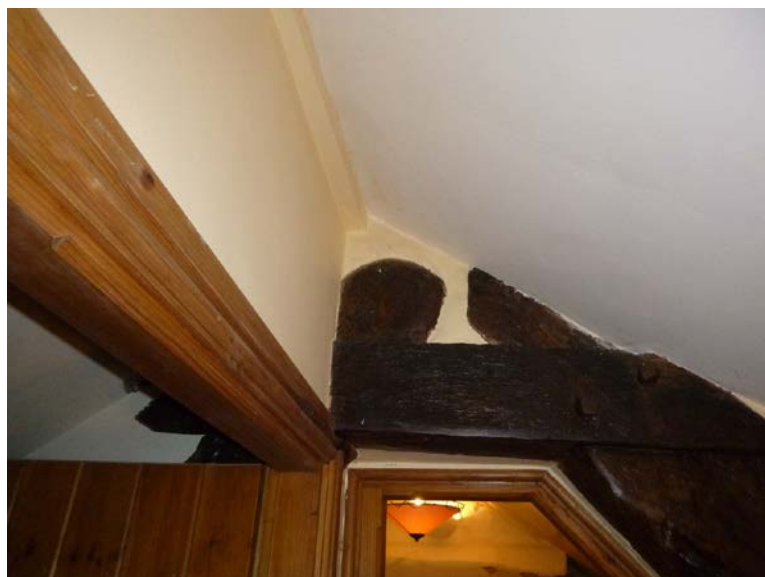
Plate 17 (left): The top of the north-west cruck blade in the north-east part of the cottage, viewed from the north Plate 18 (right): The collar of the cruck truss in the north-east part of the cottage, viewed from the north-east
