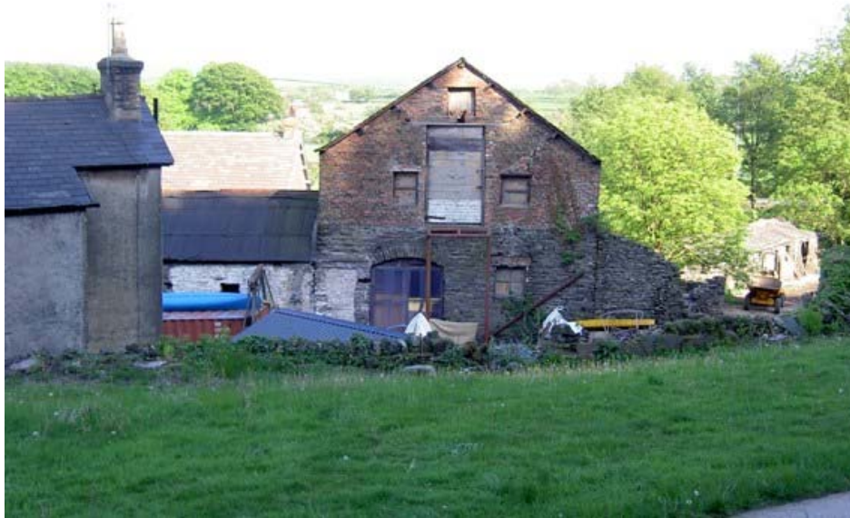
Plate 14: West external elevation
