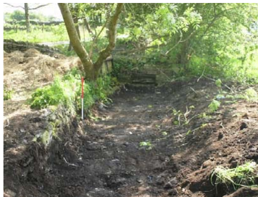
Plate 34: Channel containing culvert alongside east boundary
