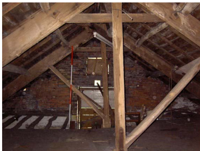
Plate 23: (left) Part of a truss on the attic floor showing pulley wheel incorporated into beam
