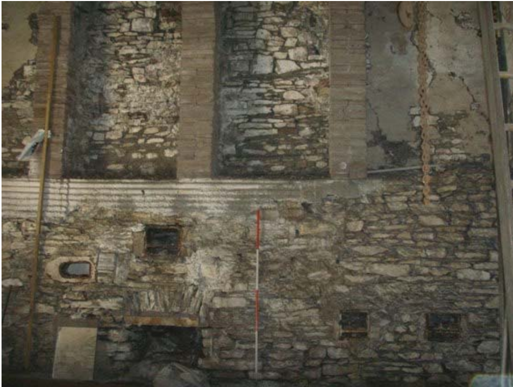
Plate 17: South internal elevation of the mill showing bearing boxes, aperture for the axle shaft, and tilt hammer head at ground floor level, and inserted concrete supports on the first floor
