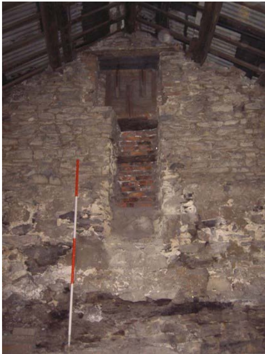
Plate 25: (left) Remains of flue in north end of northern extension
