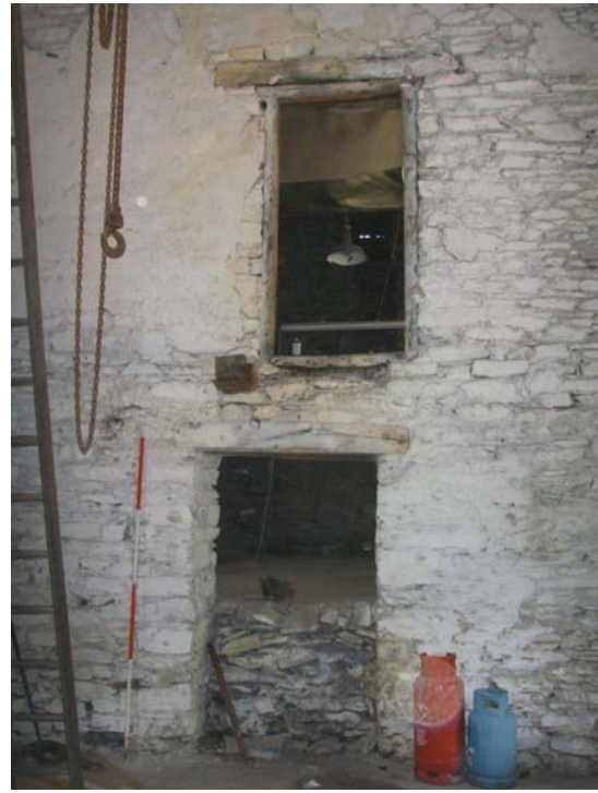
Plate 18: (left) Timber block, perhaps a bearing, attached to the south side of the east elevation
