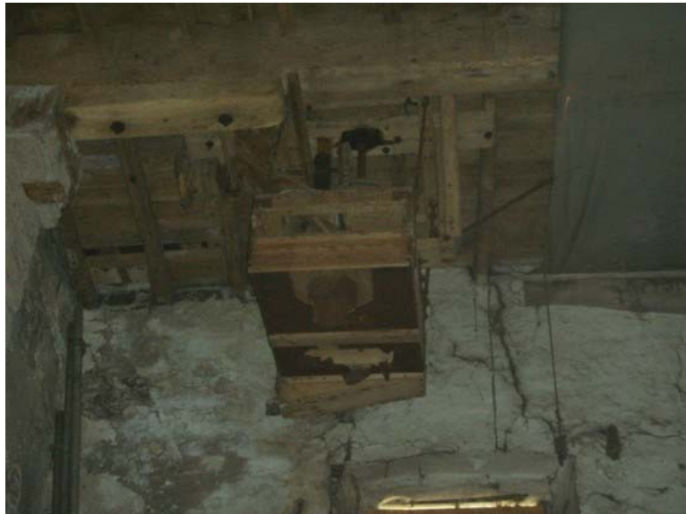
Plate 20: Timber box or hopper attached to first floor ceiling/second floor joists
