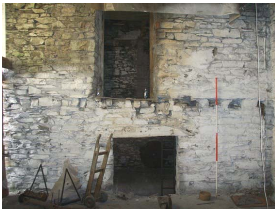
Plate 27: (left) South elevation of northern extension showing doorways and empty joist slots for first floor
