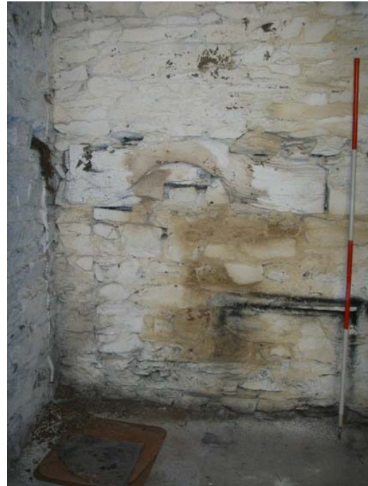
Plate 25: (left) Remains of flue in north end of northern extension
