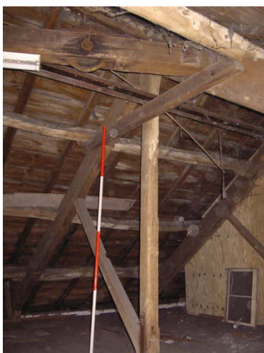
Plate 23: (left) Part of a truss on the attic floor showing pulley wheel incorporated into beam
