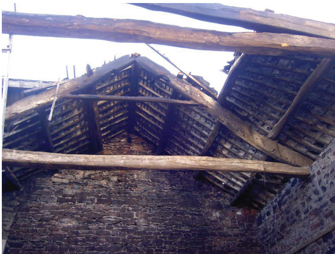
Plate 41: Southern roof truss, Building 9
