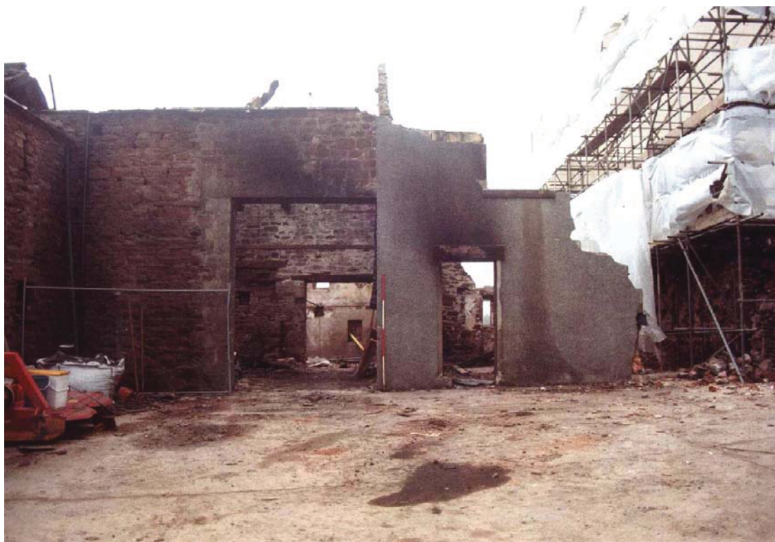
Plate 16: Rendered west elevation of re-built part of Building 6
