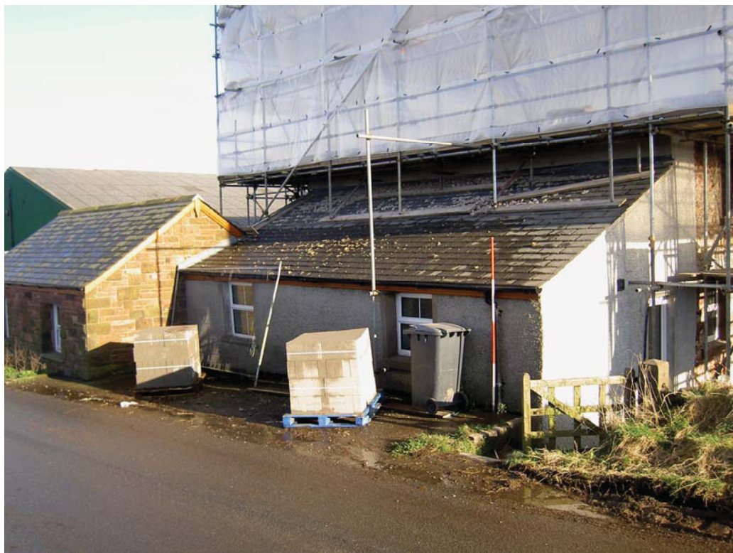
Plate 8: Building 2 from the north-west
