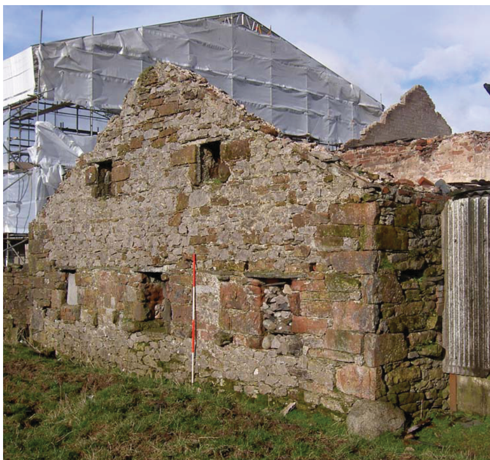
Plate 24: West elevation of Building 8
