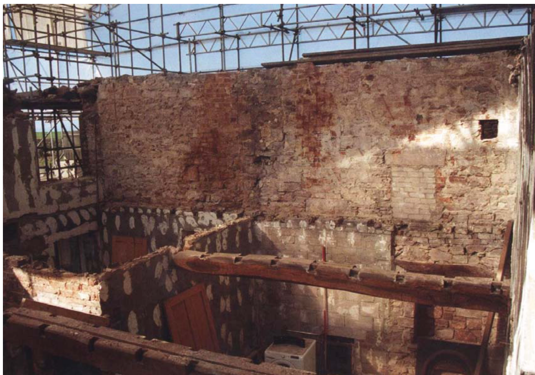
Plate 32: North elevation of Building 4
