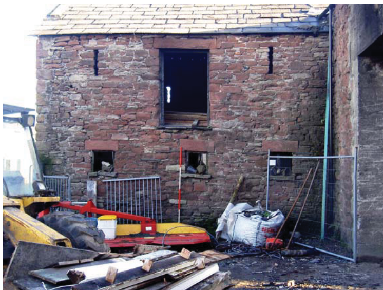
Plate 25: Building 10 from the north
