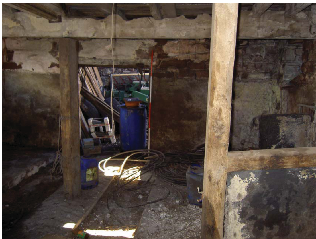
Plate 44: Stall partitions in shippon of Building 10
