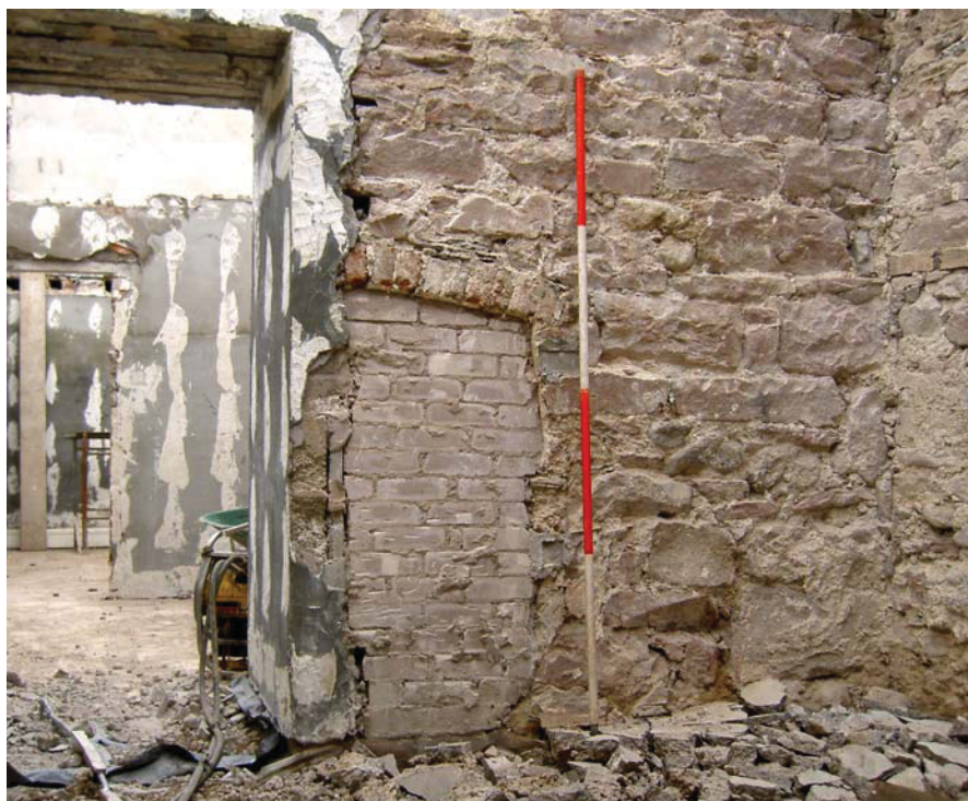
Plate 30: Doorway inserted through blocked fireplace, South elevation Building 3
