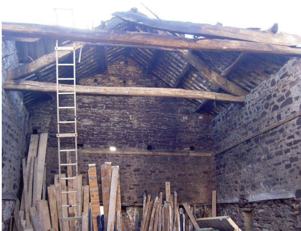
Plate 40: South elevation of Building 9
