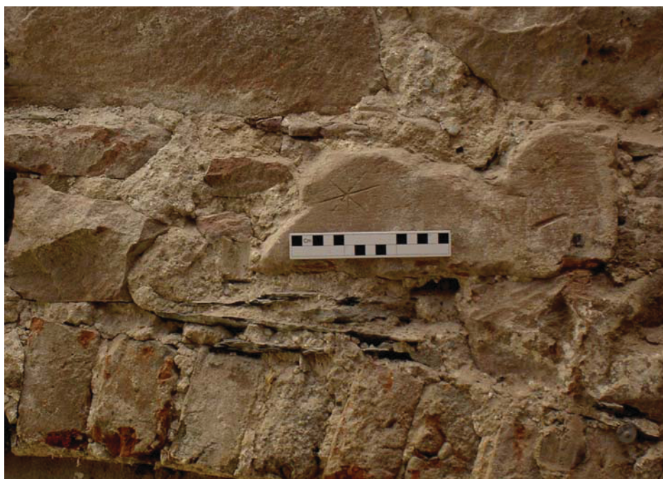
Plate 31: Masons mark over blocked fireplace, South elevation of Building 3
