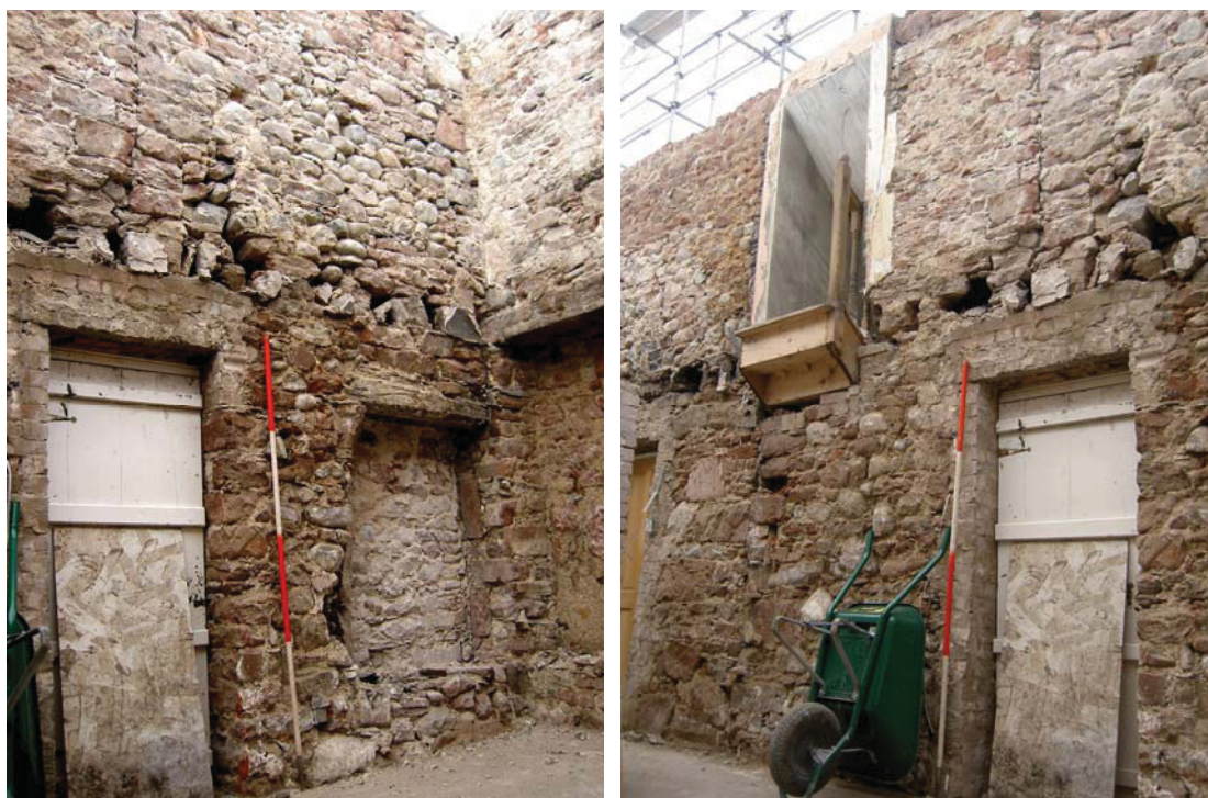
Plate 27: (left) Inserted door and blocked window in north elevation of Building 3
