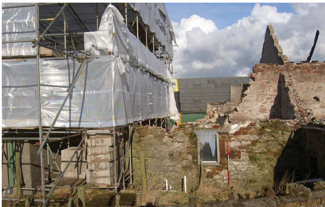
Plate 23: West elevation of Building 7
