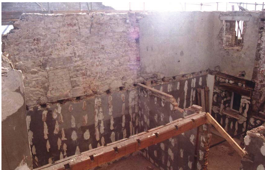
Plate 33: South elevation of Building 4
