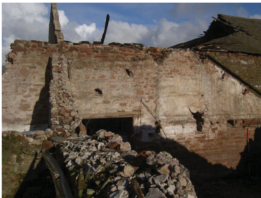
Plate 43: Gable scar of Building 8 on West elevation of Building 9
