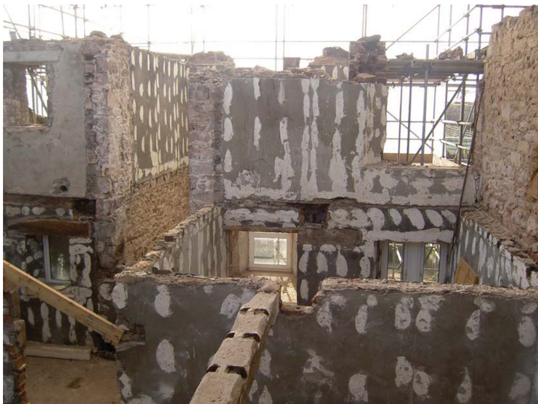
Plate 34: West elevation of Building 4
