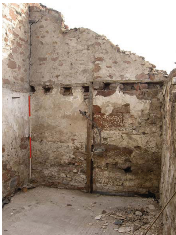
Plate 42: Blocked door of Building 8 in South elevation of Building 7
