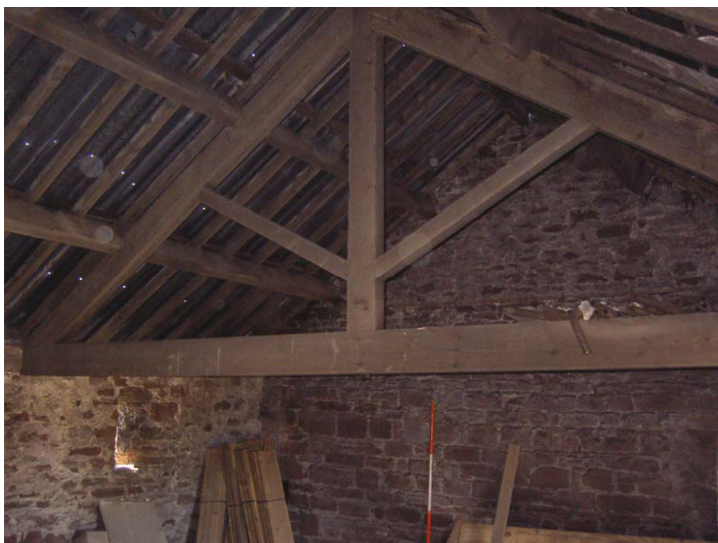
Plate 45: East side of truss in hayloft, Building 10
