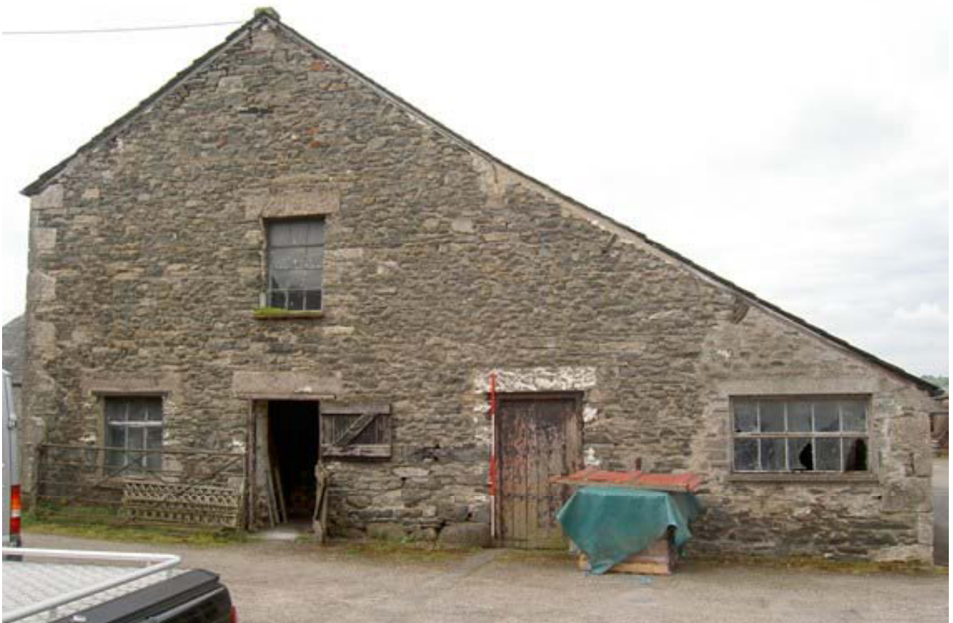
Plate 7: East elevation (north part)
