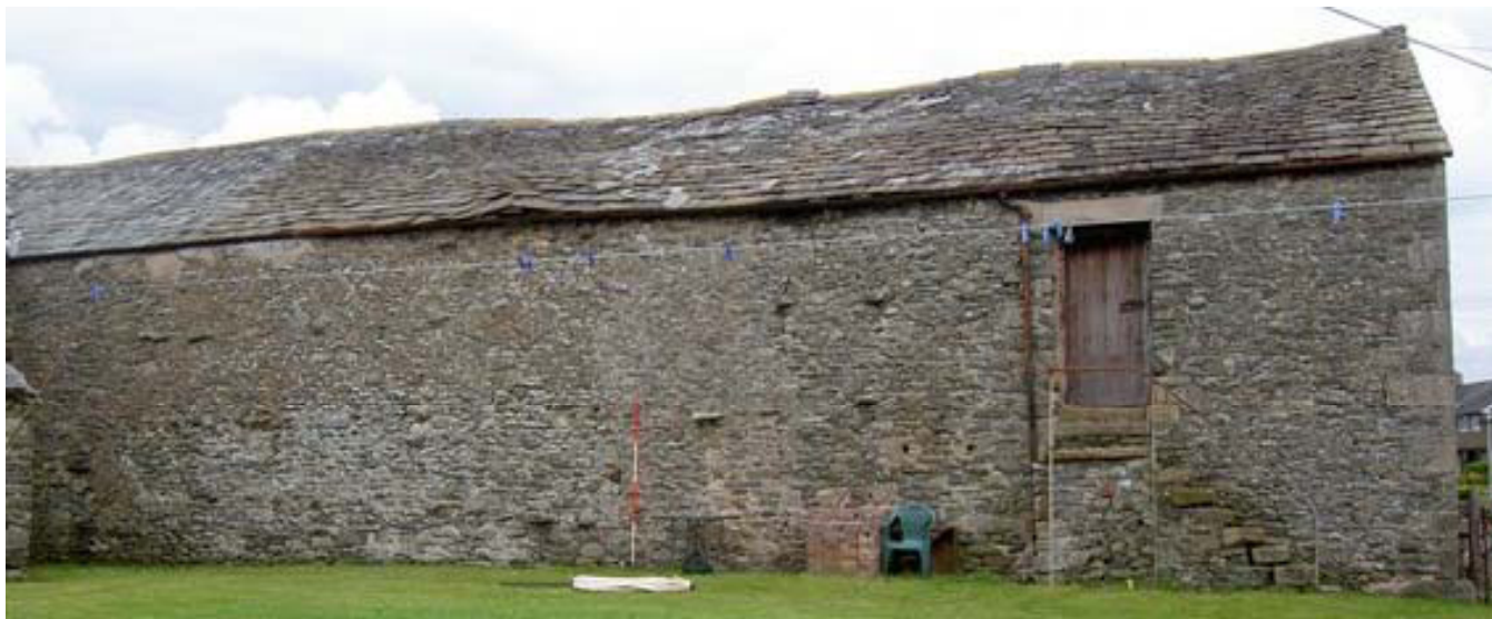
Plate 11: South external elevation of Rooms 1a, 2 and 8
