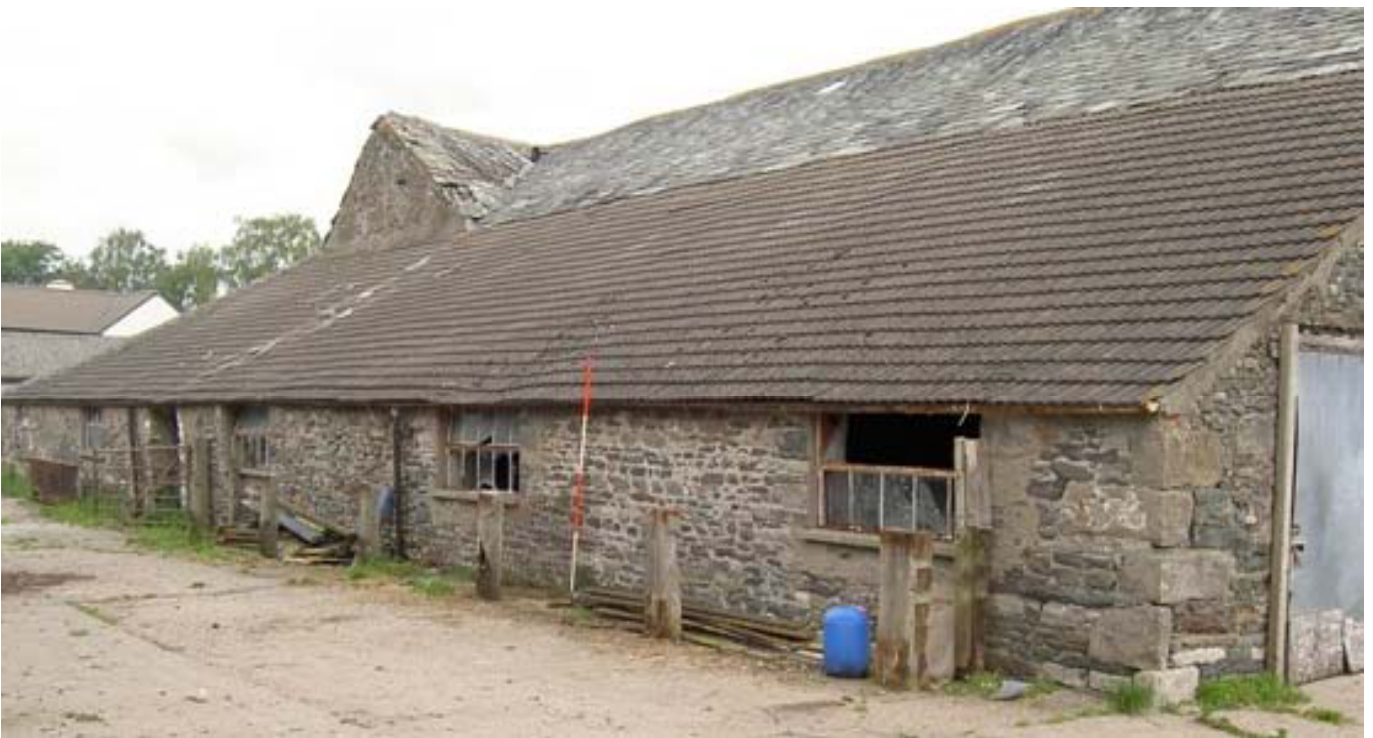
Plate 13: South end of the west elevation
