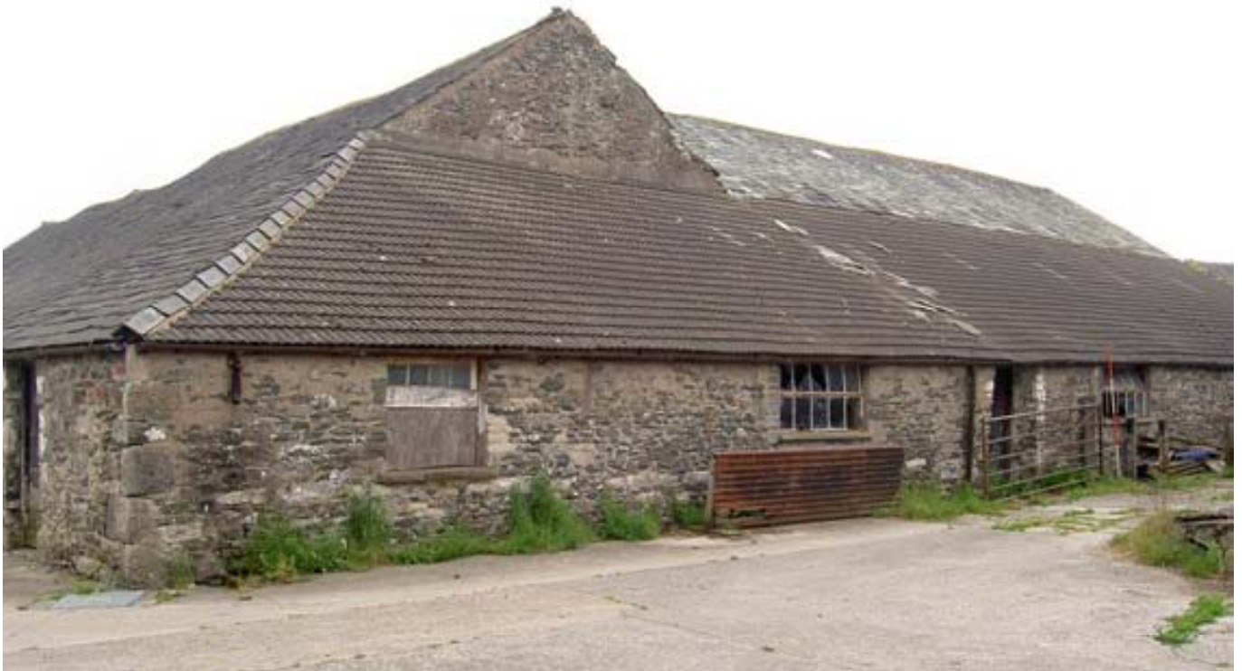
Plate 12: North end of the west elevation
