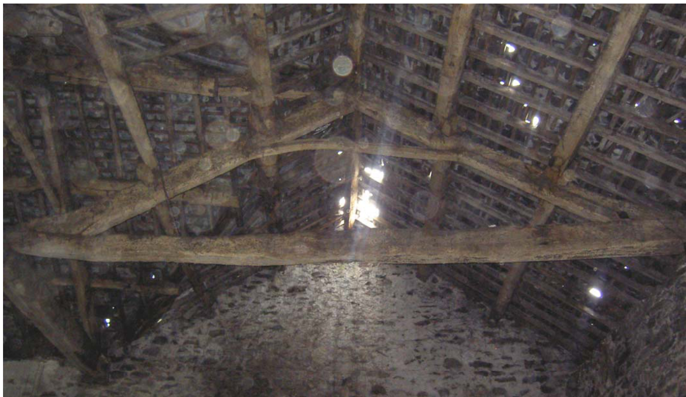
Plate 14: West truss, Room 1a
