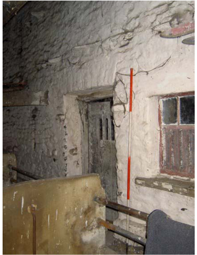
Plate 24: (left) Blocked doorway under a drip course at the west end of the south elevation, Room 3
