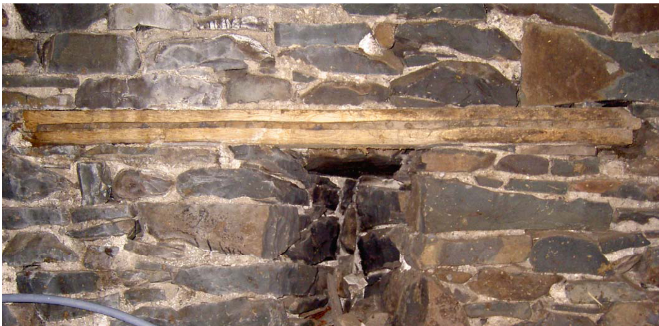
Plate 20: Re-used partition rail over slot vent, east elevation of Room 1b
