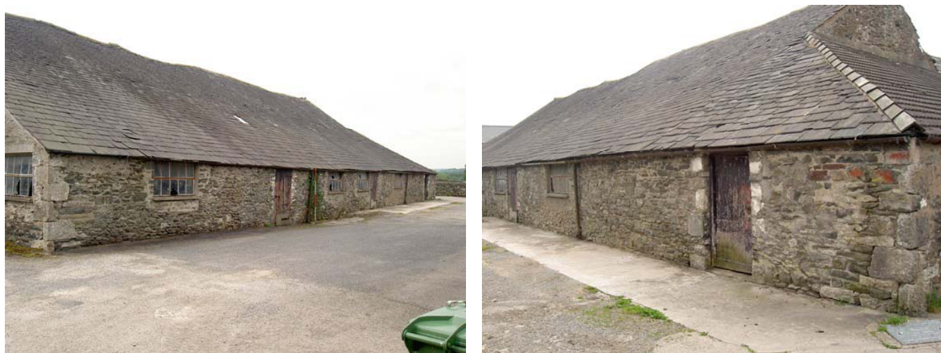
Plate 5: (left) North elevation, east end
