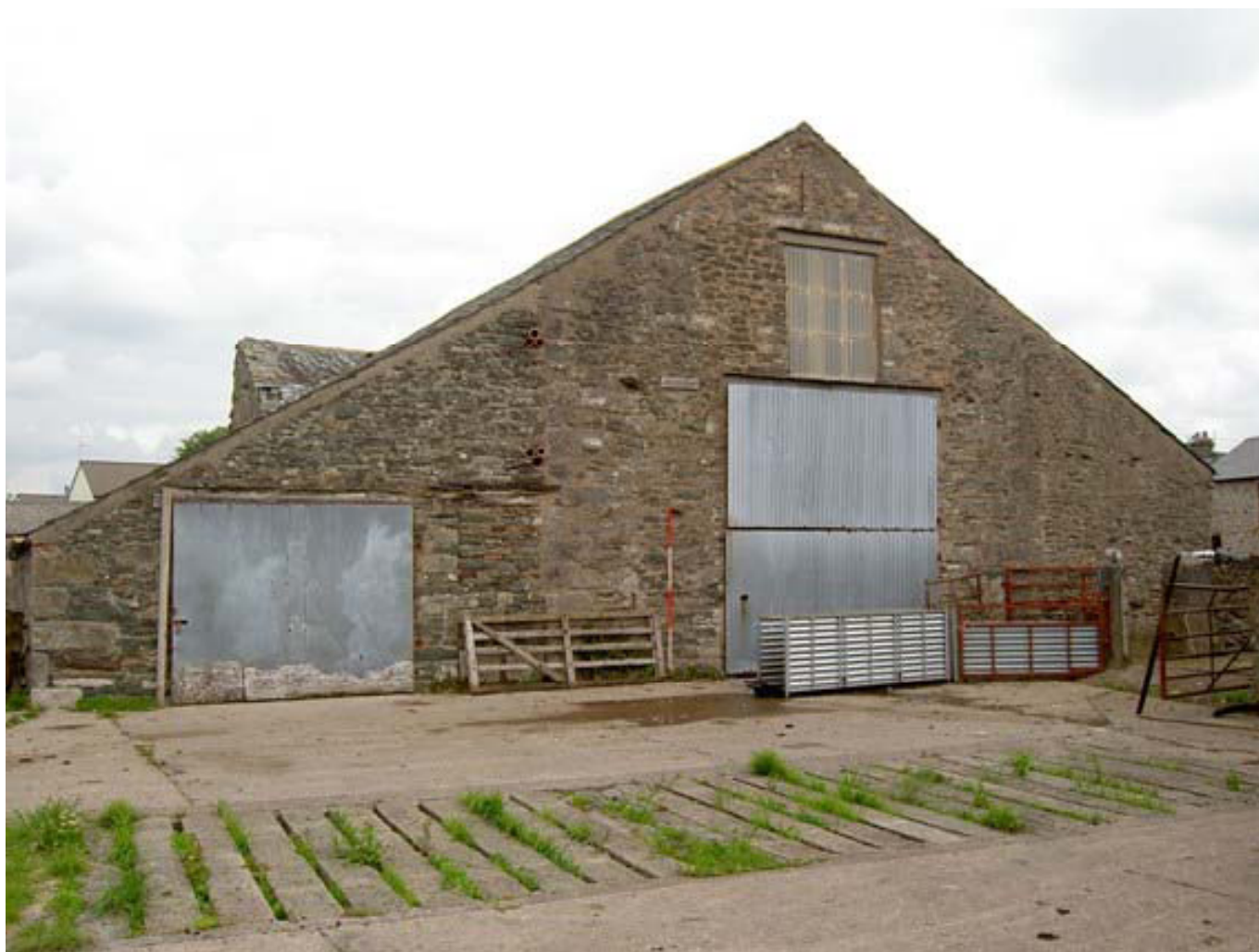
Plate 10: South elevation (west part)
