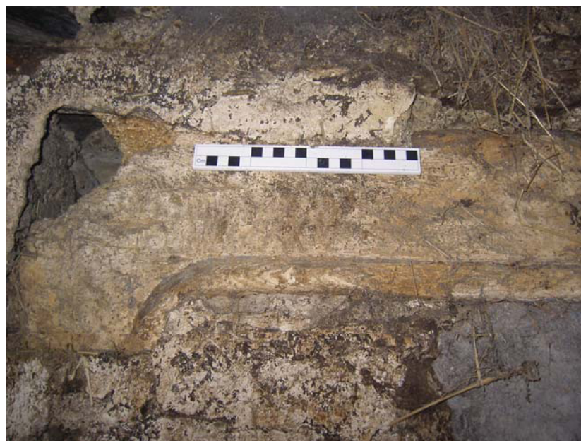
Plate 15 (left): Blocked doorway in the south-west end of the barn with re-used timber with moulded decoration (photograph by Greenlane Archaeology Ltd)
