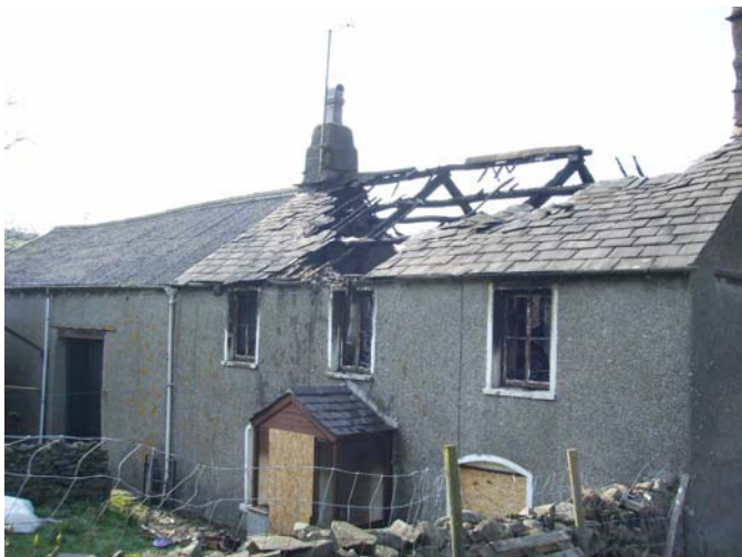
Plate 13 (left): North-west elevation, showing the roof trusses (photograph taken by Dan Elsworth)
