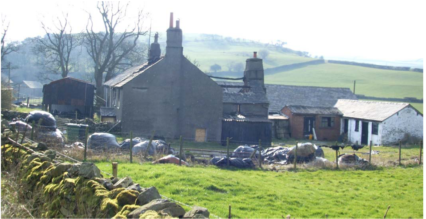
Plate 9: North-east side of farmhouse, showing wing to the rear (photograph by Dan Elsworth)
