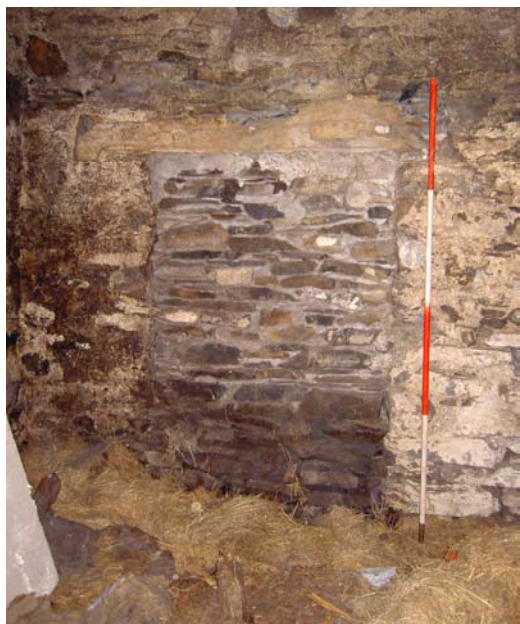
Plate 15 (left): Blocked doorway in the south-west end of the barn with re-used timber with moulded decoration (photograph by Greenlane Archaeology Ltd)
