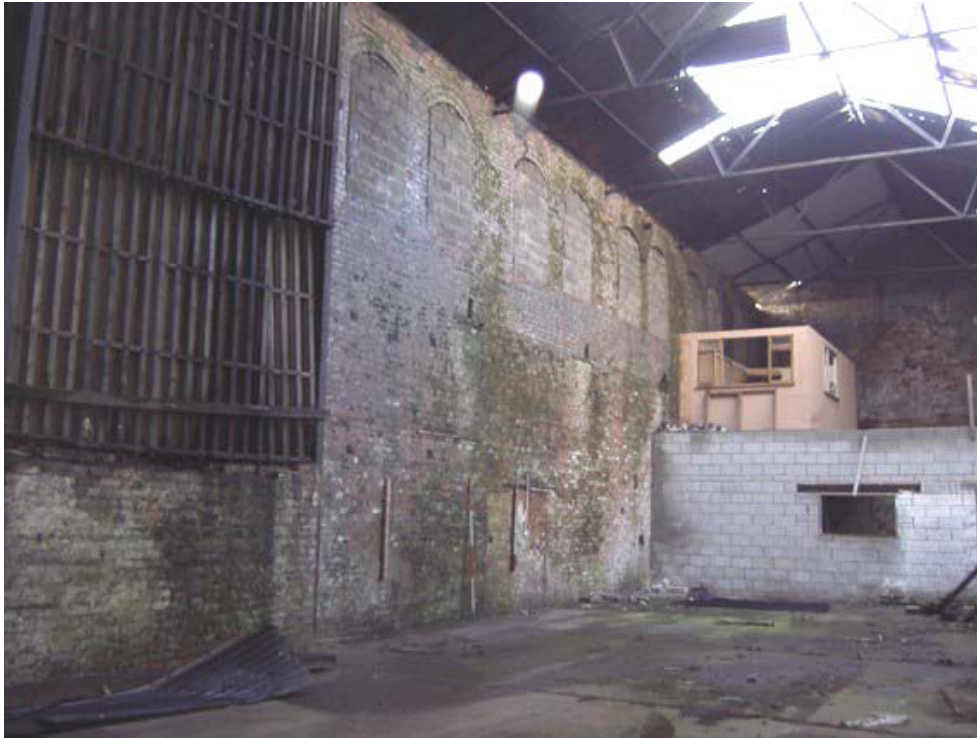
Plate 37: Internal south elevation of Building 3
