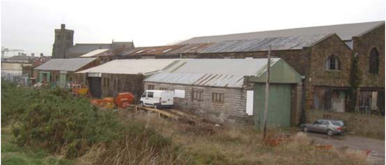
Plate 24: South external elevation of Building 3
