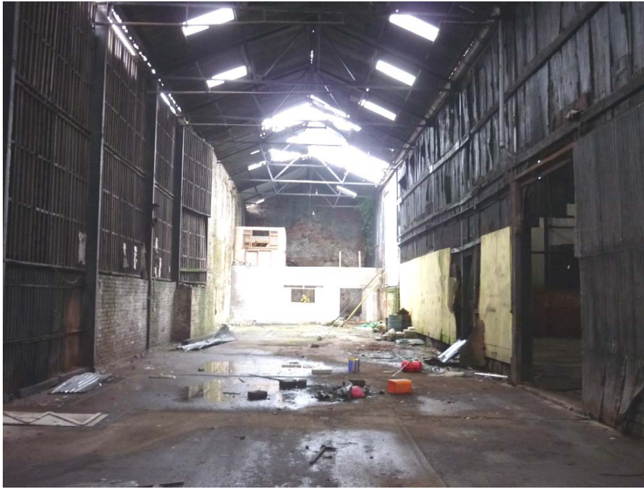
Plate 33: General view of the inside of Building 3, facing west
