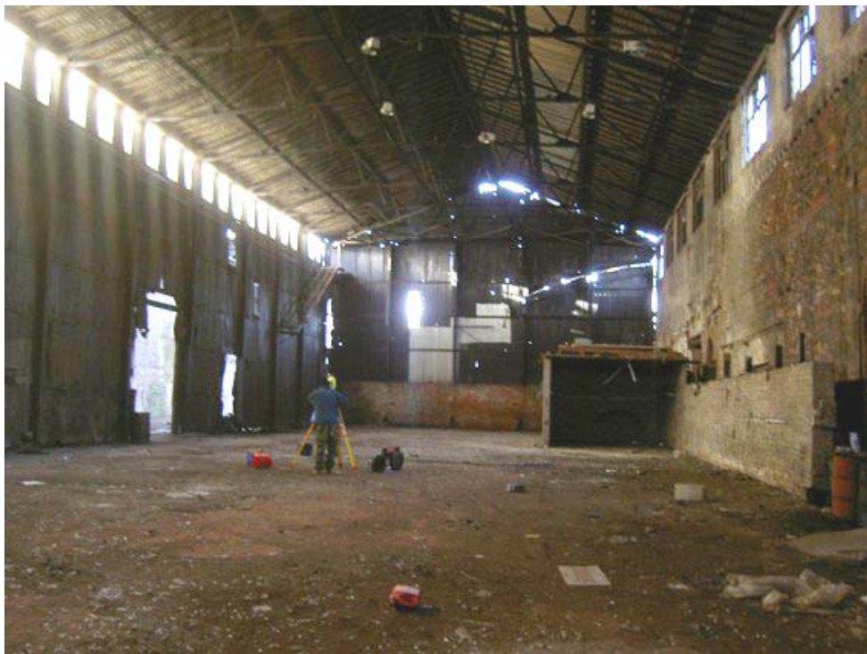
Plate 31: General view of the west end of Building 2
