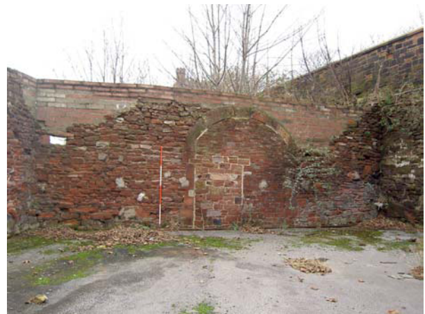
Plate 25 (left): Buttresses against the west end of the northern boundary wall
