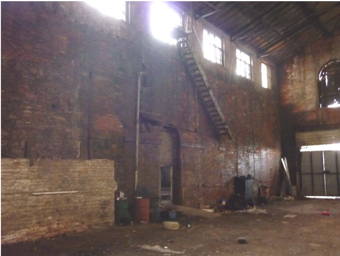
Plate 30: Ladder in the north-east corner of Building 2
