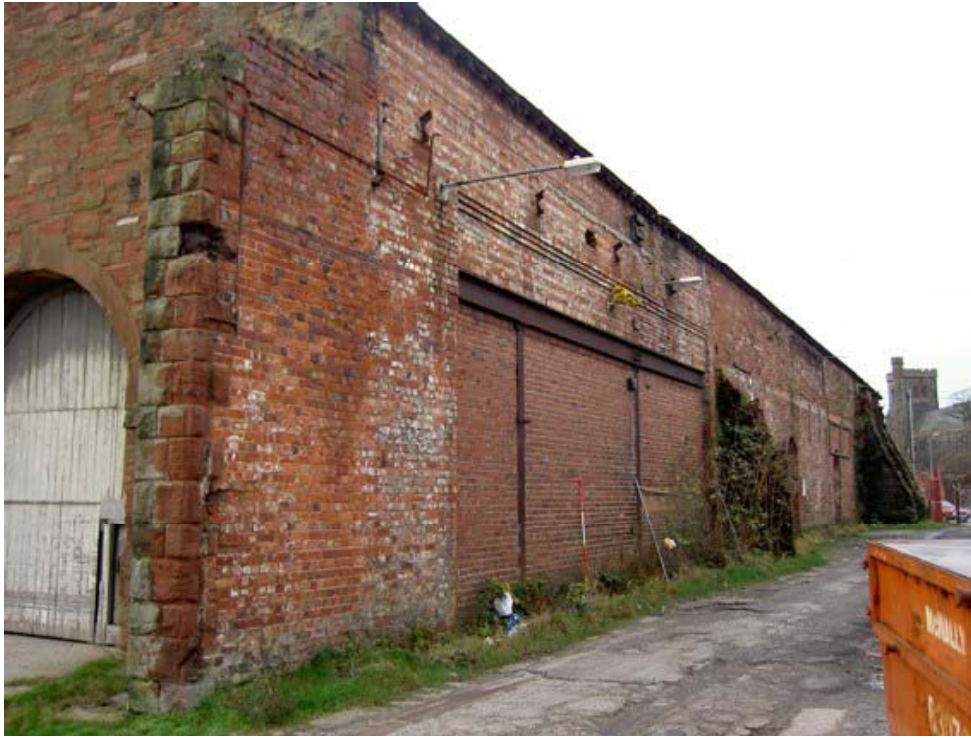
Plate 18: North external elevation of Building 1
