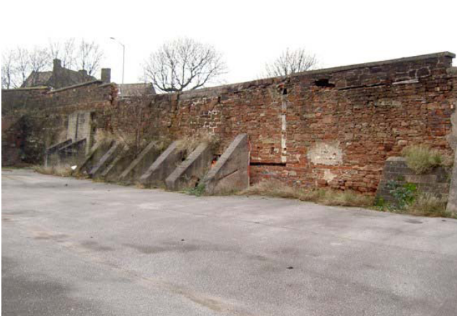
Plate 25 (left): Buttresses against the west end of the northern boundary wall
