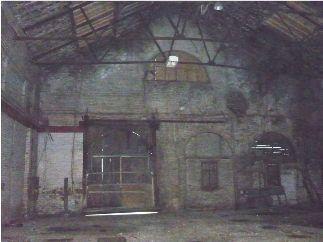
Plate 29: Internal east elevation of Building 1
