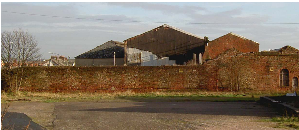
Plate 28: West external elevation of Buildings 1-3 and the boundary wall
