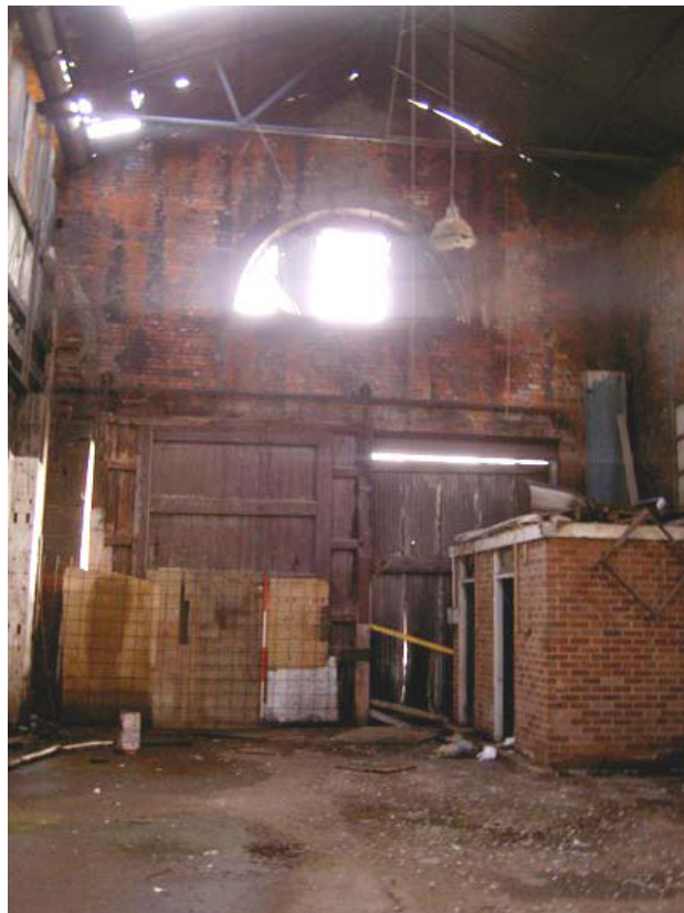
Plate 38: Internal east elevation of Building 3
