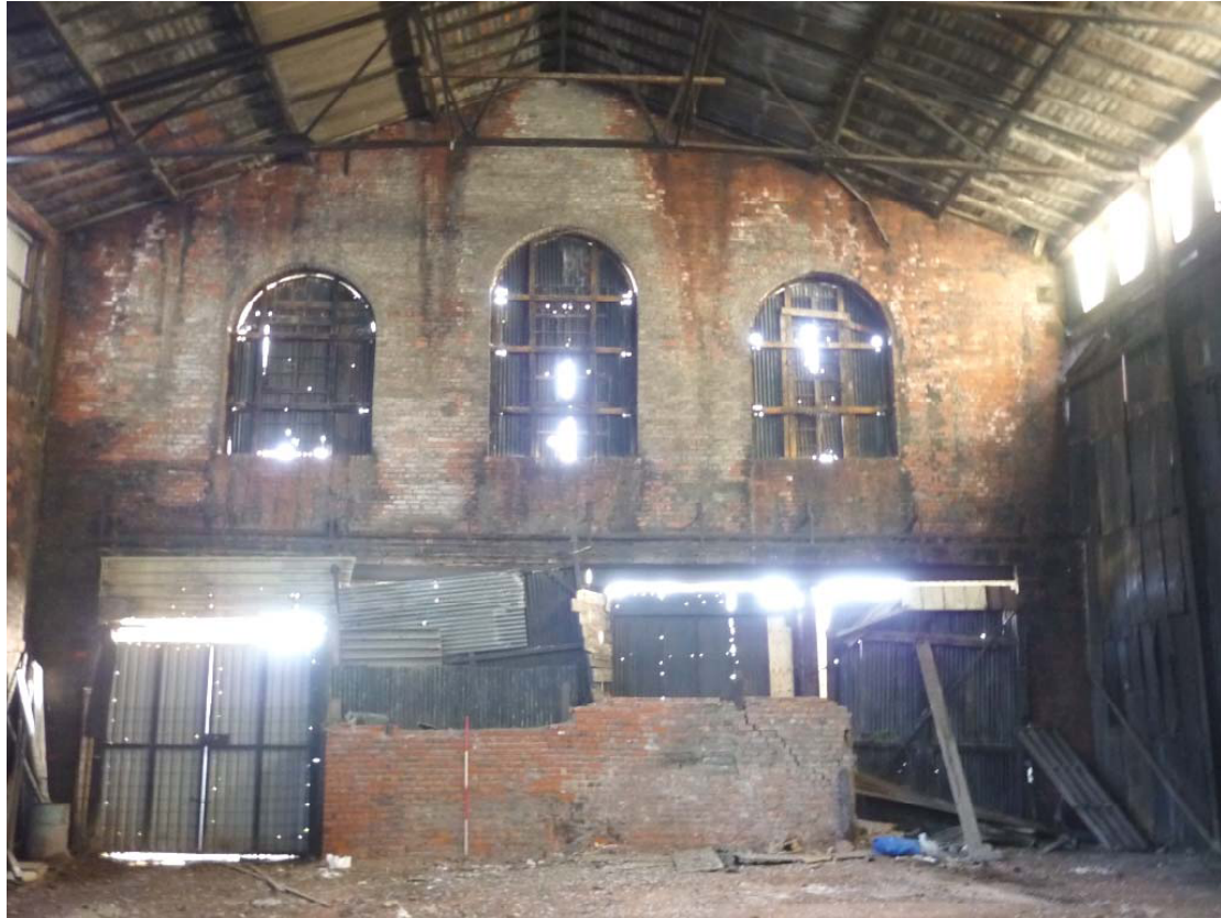
Plate 32: Internal east elevation of Building 2
