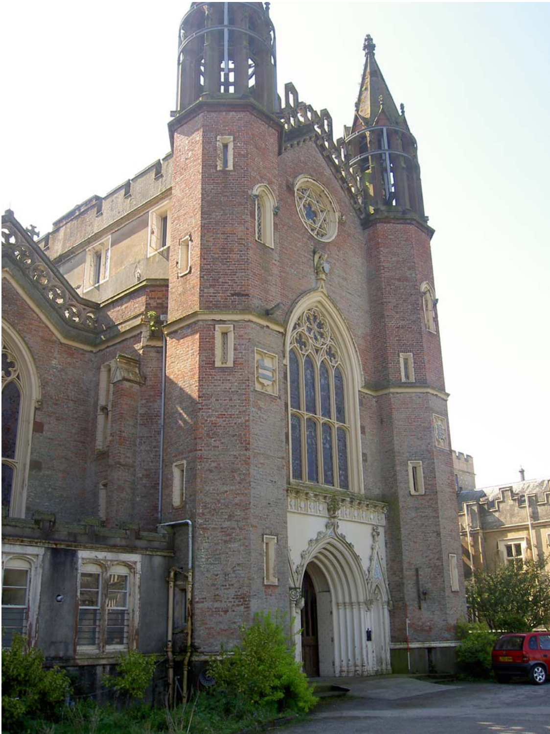
Plate 47: Phase 3 toilet block on the east side of the north entrance
