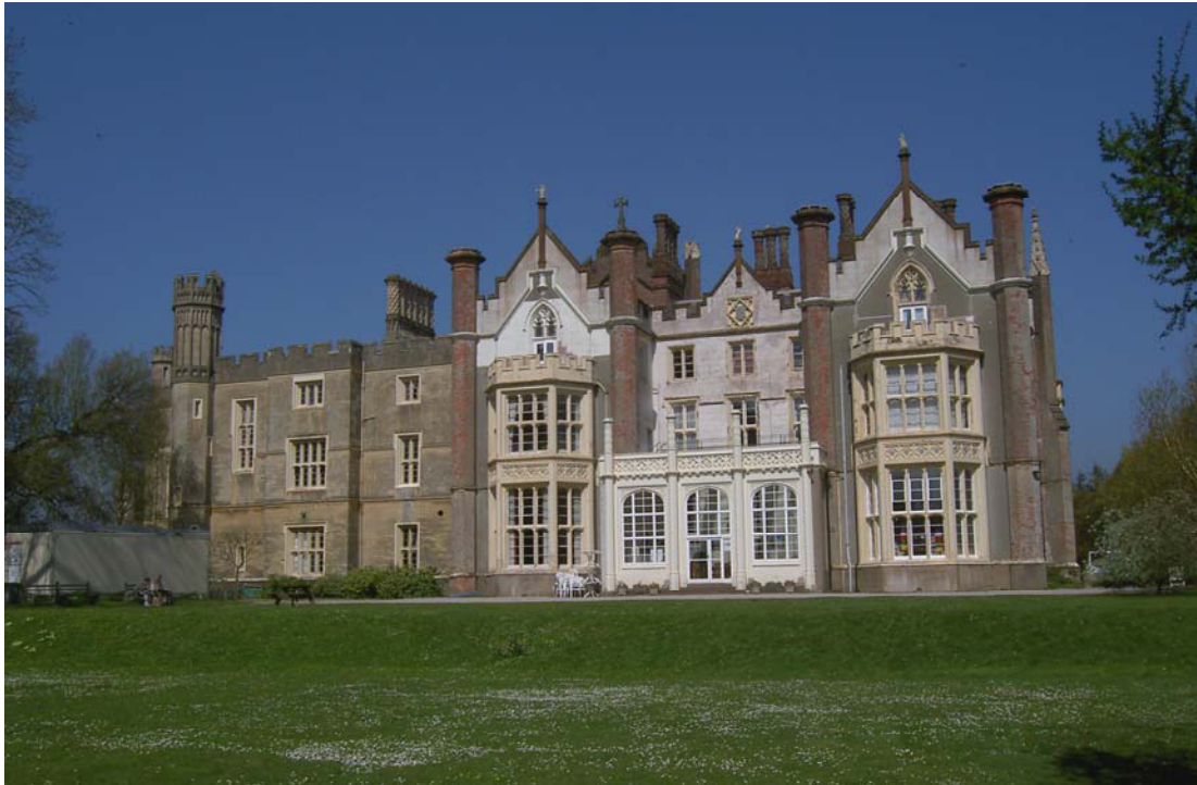
Plate 41: The two southernmost elements of the building, from the south
