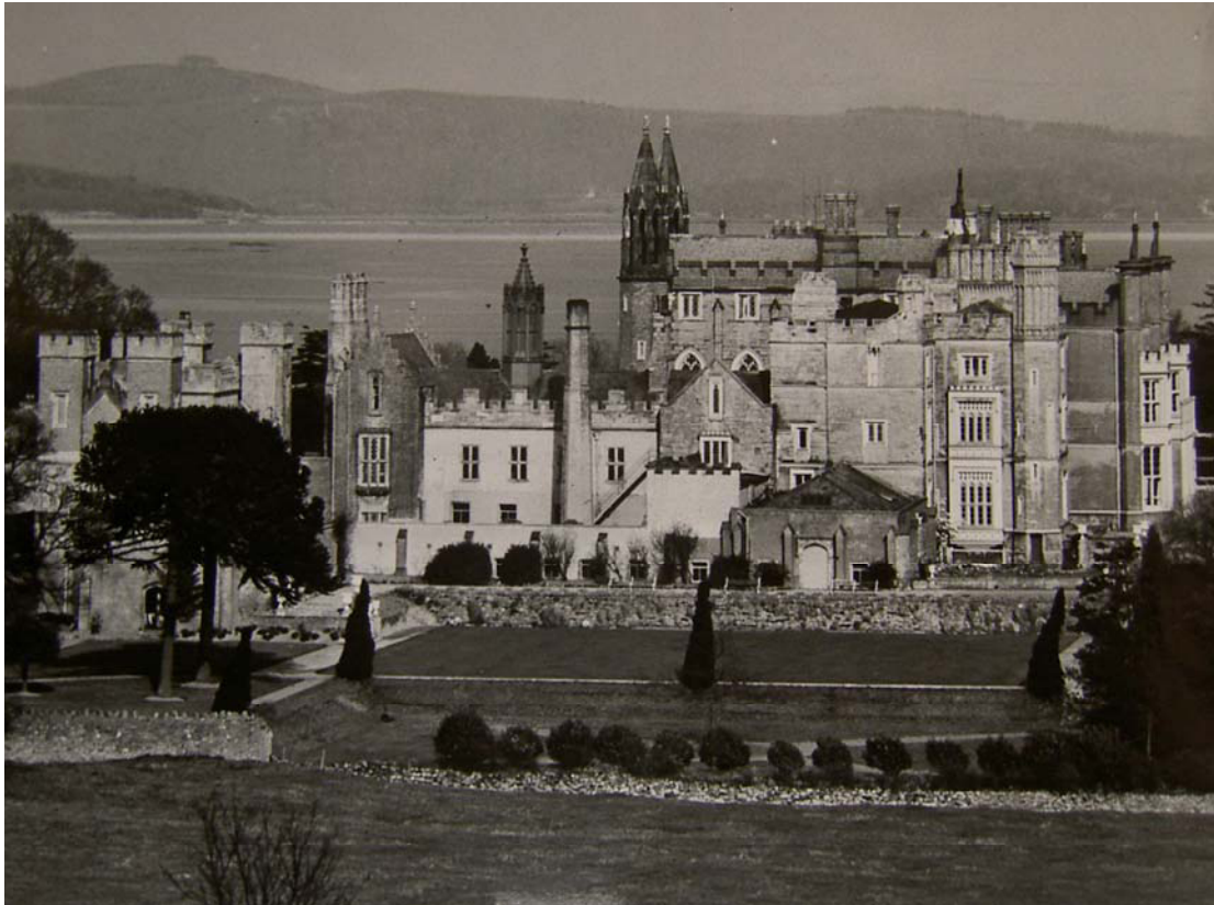
Plate 48: Phase 4 photograph showing boiler house chimney (CRO(K) WDX 427/2 1928)
