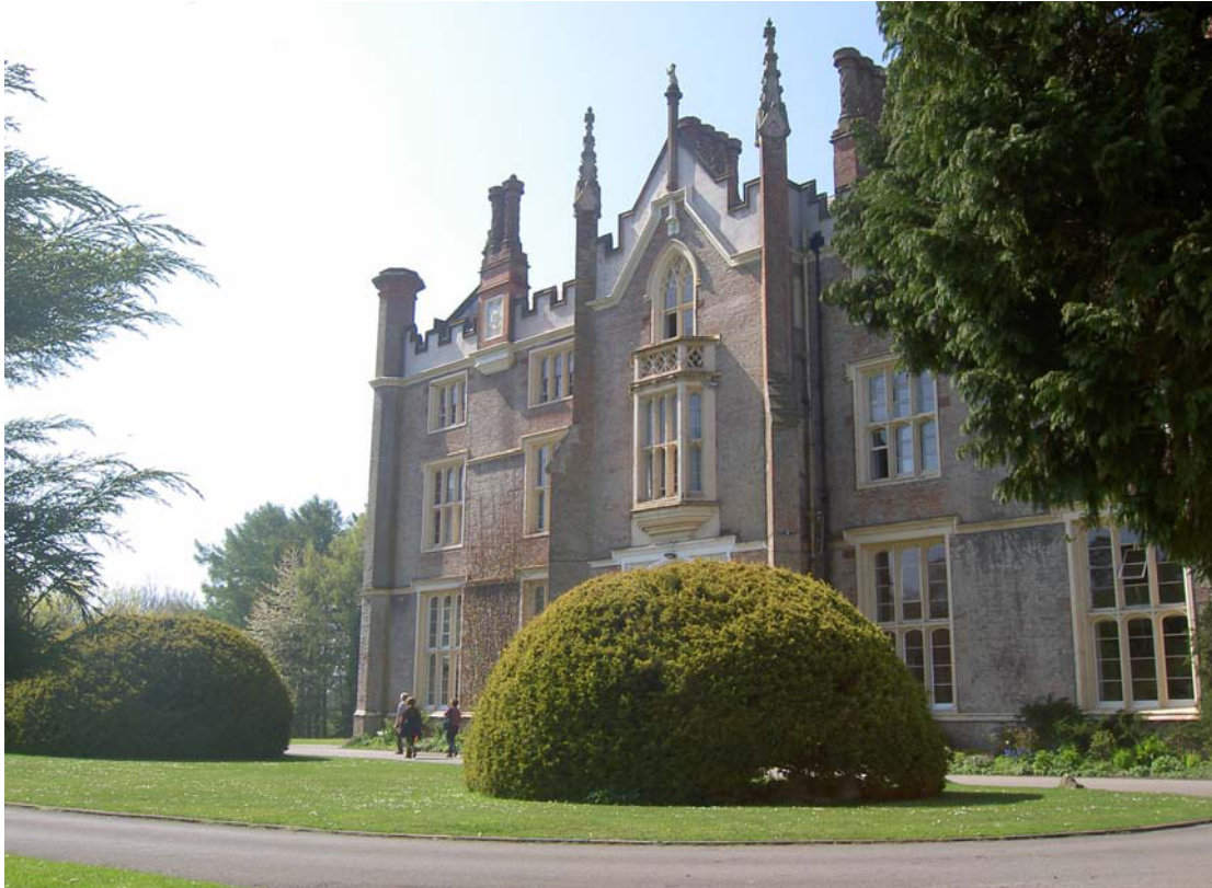
Plate 43: Main entrance way from the north-east
