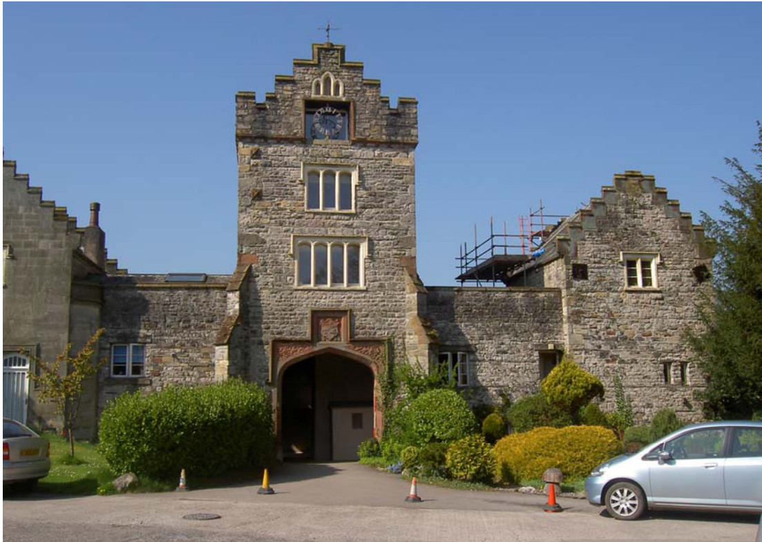
Plate 44: Phase 2 clock tower, from the east side
