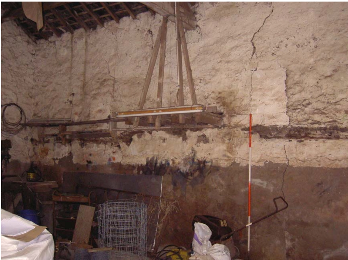
Plate 24: Relict upper floor, east elevation of Building 9
