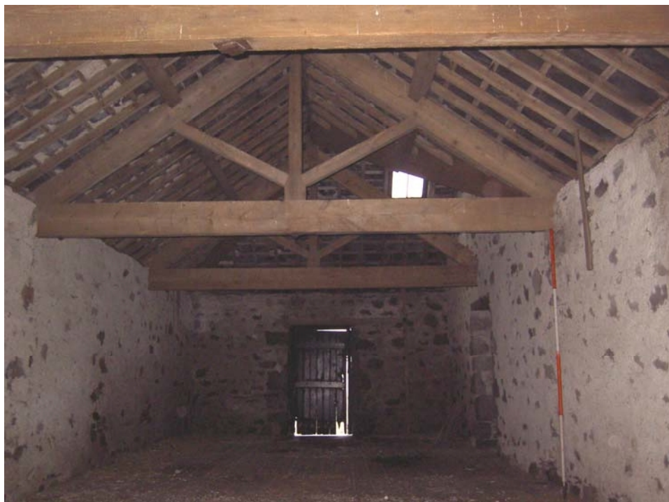
Plate 17: Roof timbers in Building 1, looking west
