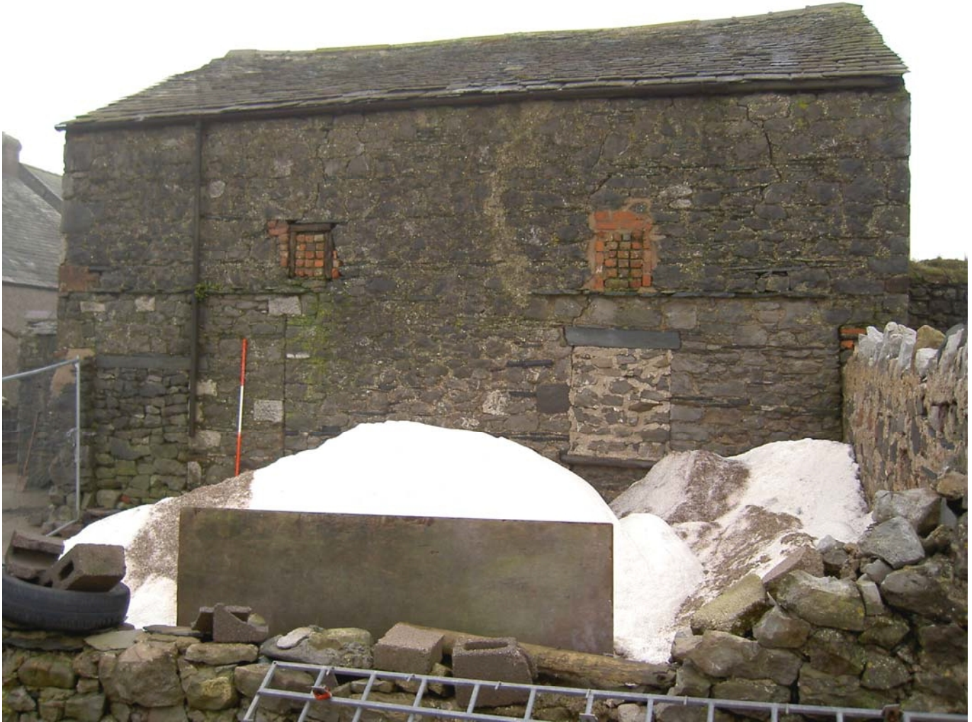
Plate 14: West elevation, Building 9
