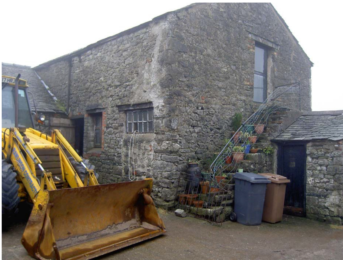
Plate 15: South-west corner of Building 9
