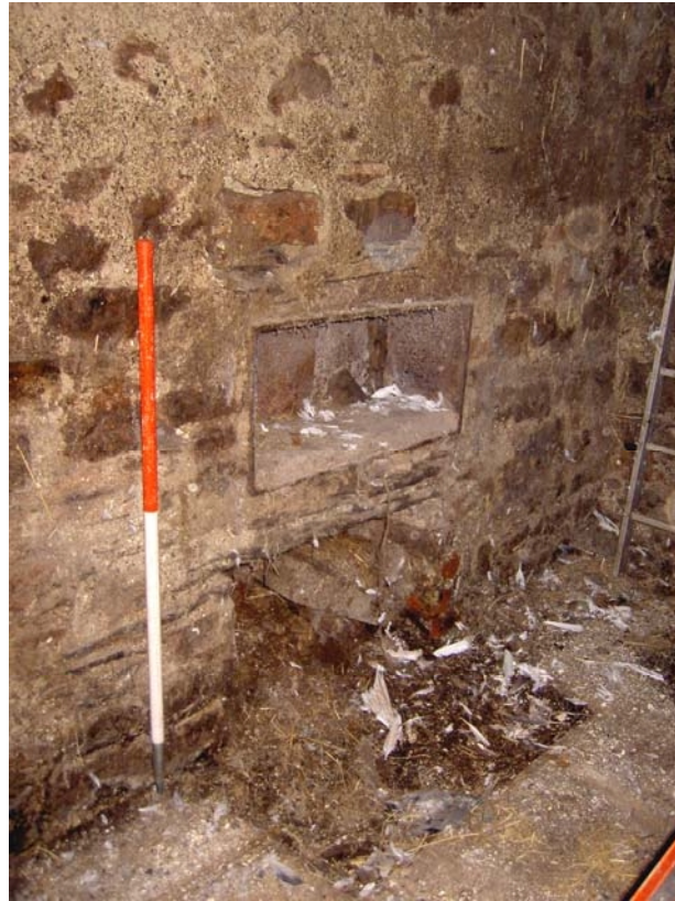
Plate 19: Bearing box in the west internal elevation of Building 2
