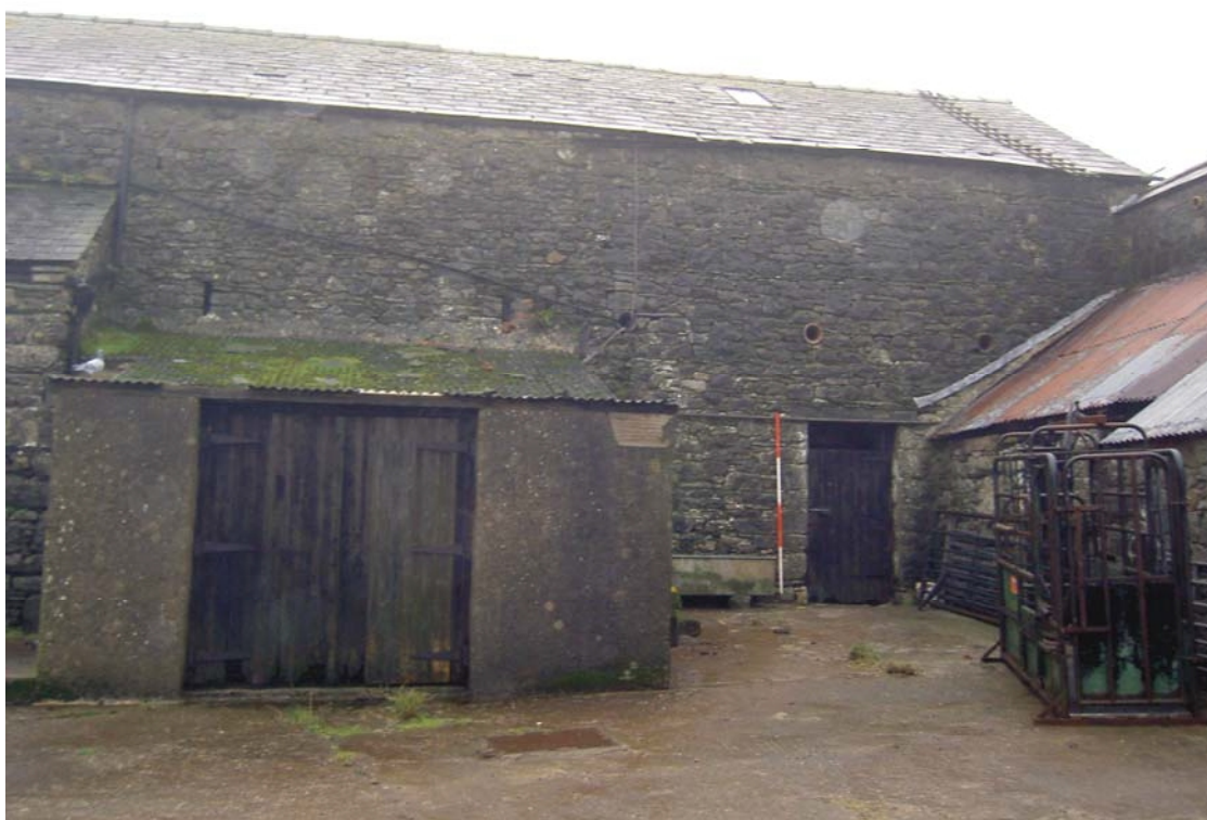
Plate 11: Building 4 viewed from the east, with Building 2/2a in background
