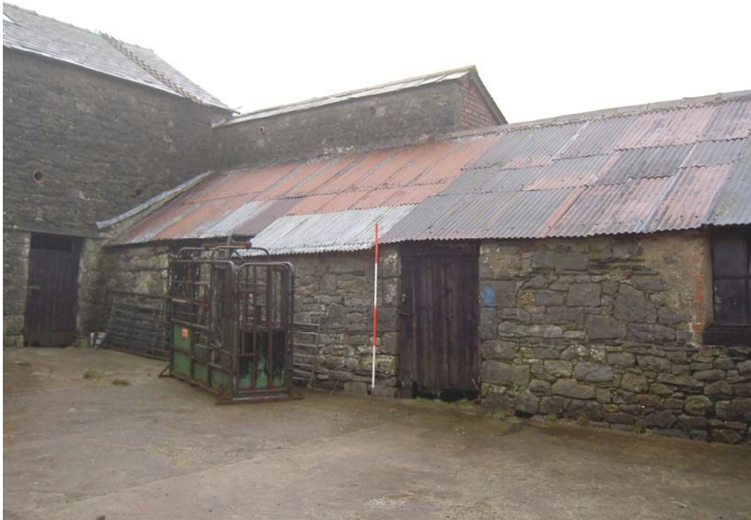
Plate 12: Cattle sheds (Buildings 5, 6 and 7) viewed from the south-west
