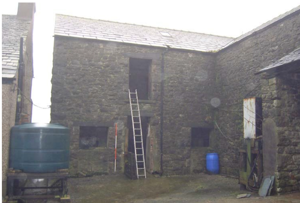
Plate 9: North elevation of Building 1
