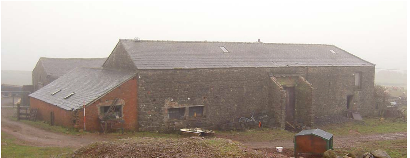
Plate 10: West elevation showing Buildings 3, 2a, 2 and 1 from left to right
