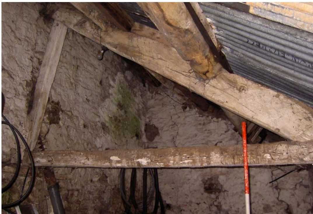
Plate 23: Re-used cruck blade in Building 7, viewed from the east
