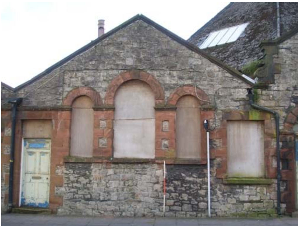
Plate 26: Central part of the north external elevation
