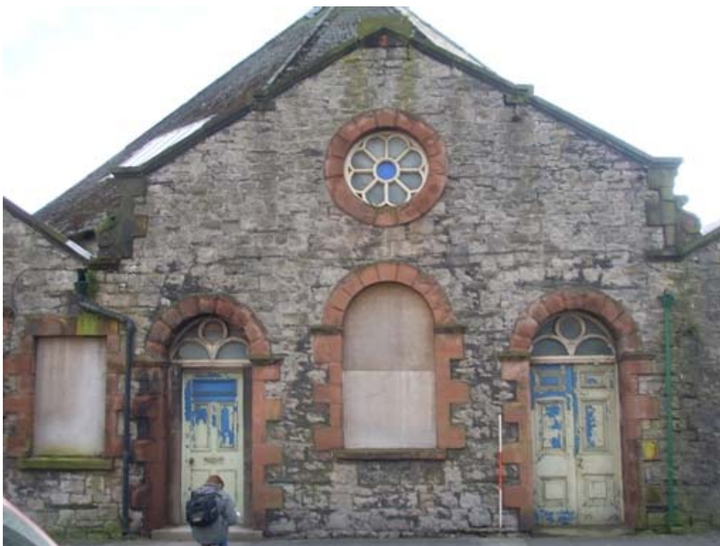
Plate 27: East end of the north external elevation
