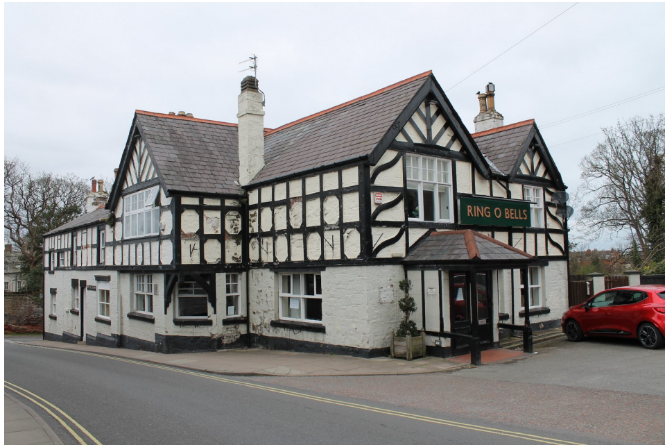
Plate 1 - View of the eastern elevation of the Ring O' Bells looking northwest.
