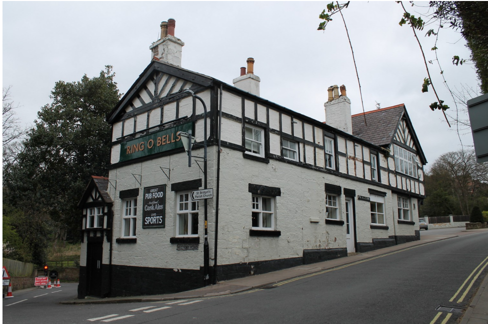
Plate 5 - View of the southern and western one and a half storey elevations of the Ring O' Bells looking northeast from Village Road.
