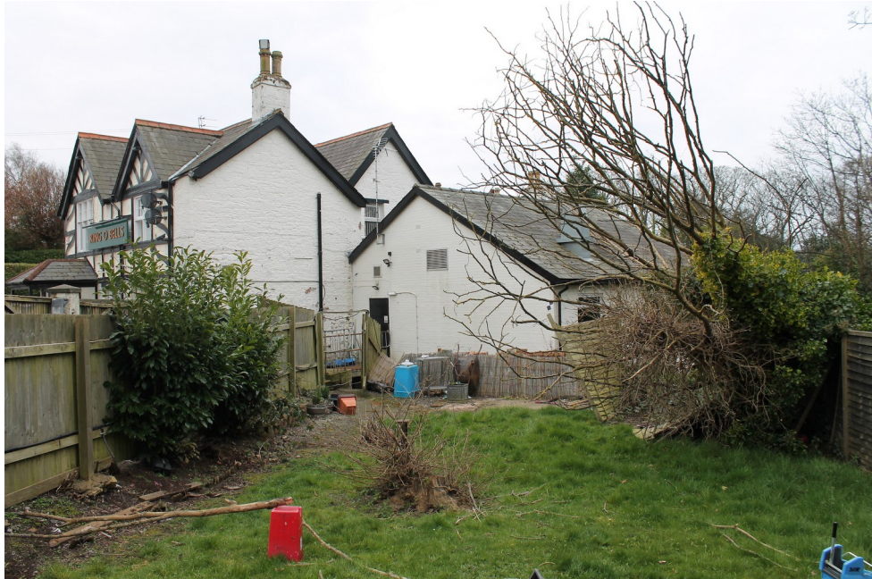
Plate 3 - View of the modern brick extension (built c.1974) on the northern elevation of the Ring O' Bells looking southwest from the end of the garden.
