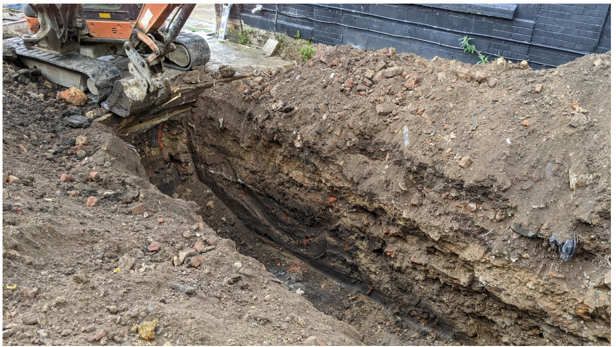
Plate 1: West-facing working shot showing section of Trench 1.
