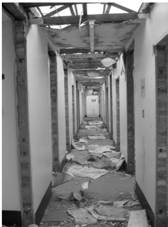
Plate 3 - Interior of building 144, facing south
