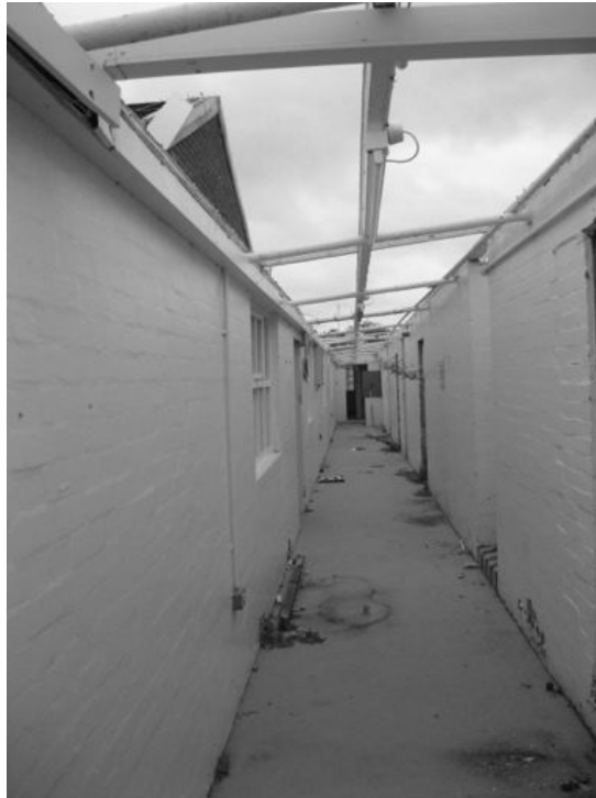
Plate 12 - Interior corridor looking east
