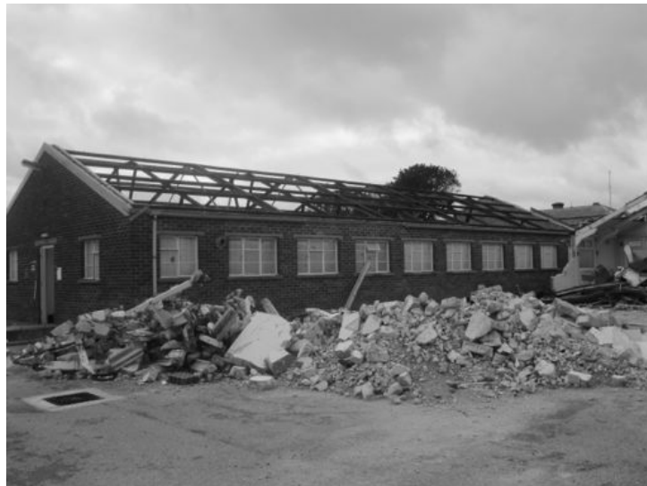
Plate 2 - West facing elevation of building 144
