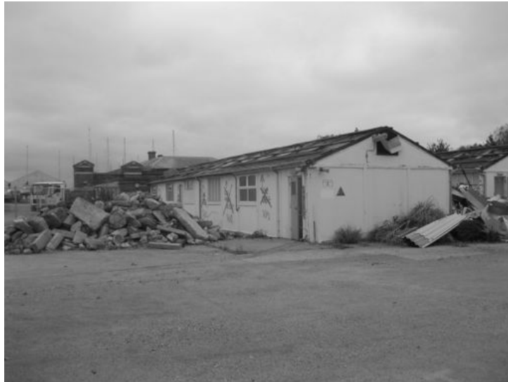
Plate 6 - North and east facing elevations of building 142
