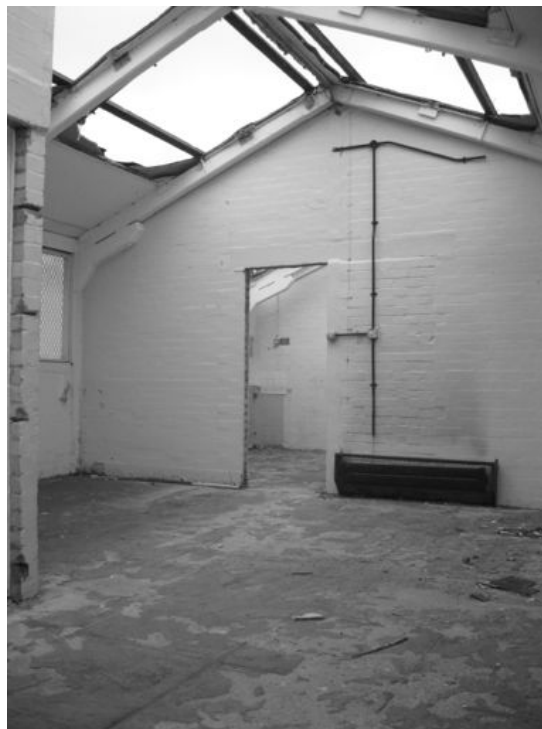
Plate 7 - Interior of building 142 looking northwest
