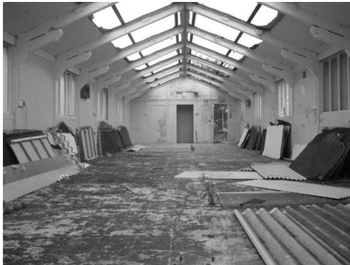
Plate 5 - Interior of building 143, looking north
