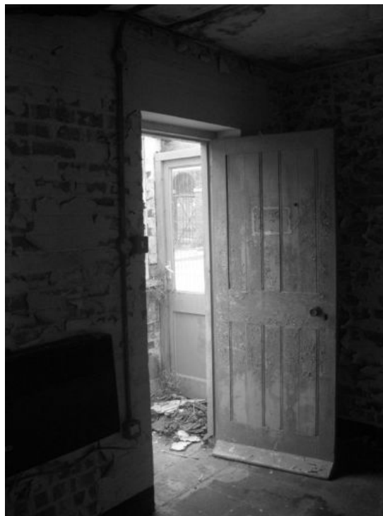
Plate 9 - Interior of building 141 looking southeast
