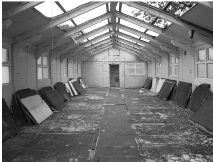
Plate 14 - Interior of building 72, looking south
