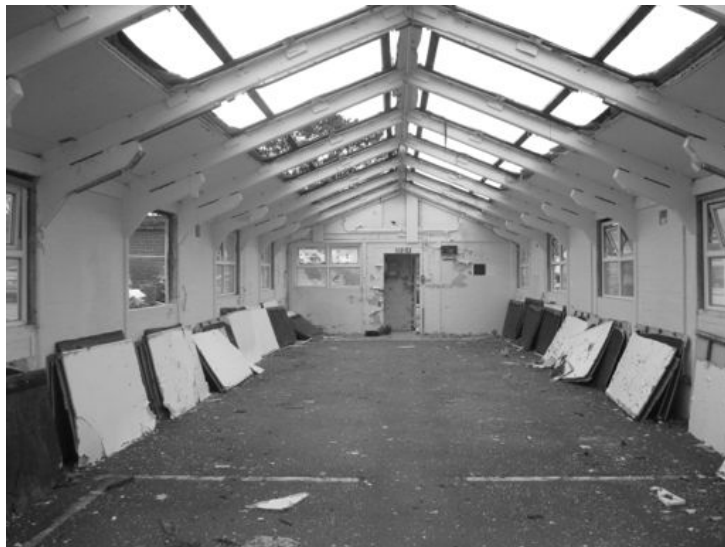
Plate 16 - Interior of building 73, looking south
