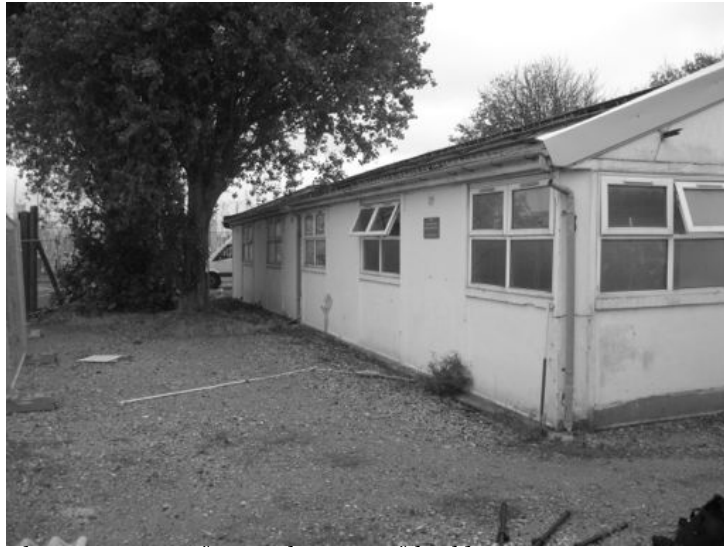
Plate 13 - West facing elevation of building 72
