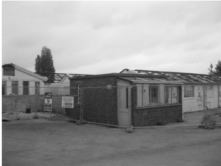
Plate 8 - Exterior of Building 141
