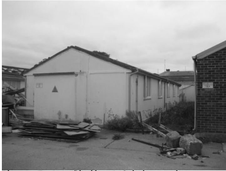
Plate 4 - Exterior of building 143, looking southeast
