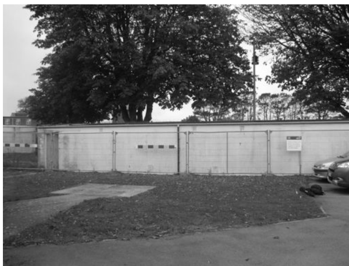
Plate 19 - East facing elevation of building 48
