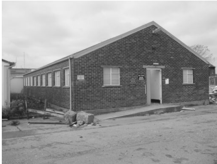
Plate 1 - North and east facing elevations of building 144
