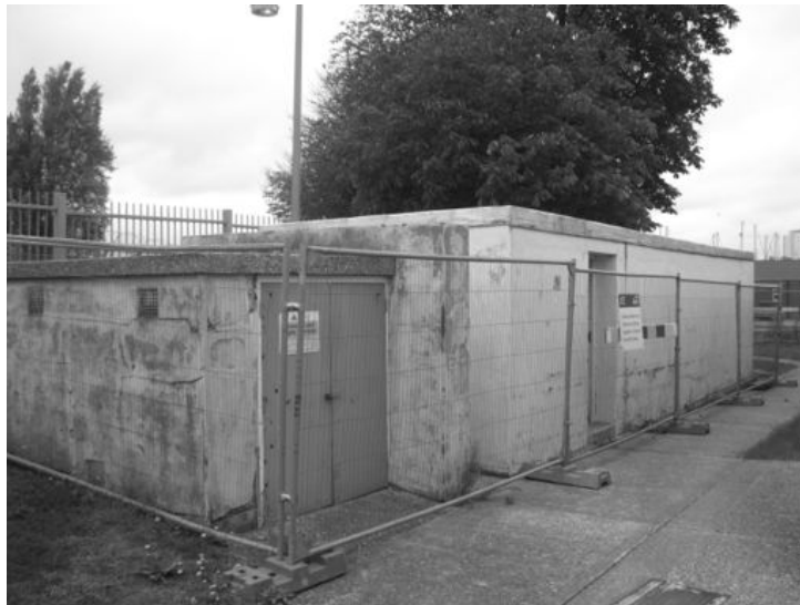
Plate 18 - Building 47 looking northwest
