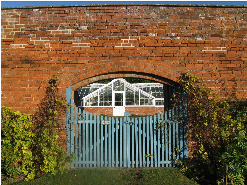
Plate 10 - Double doorway (H) looking north
