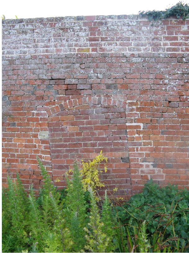
Plate 5 - Blocked doorway (B) looking east
