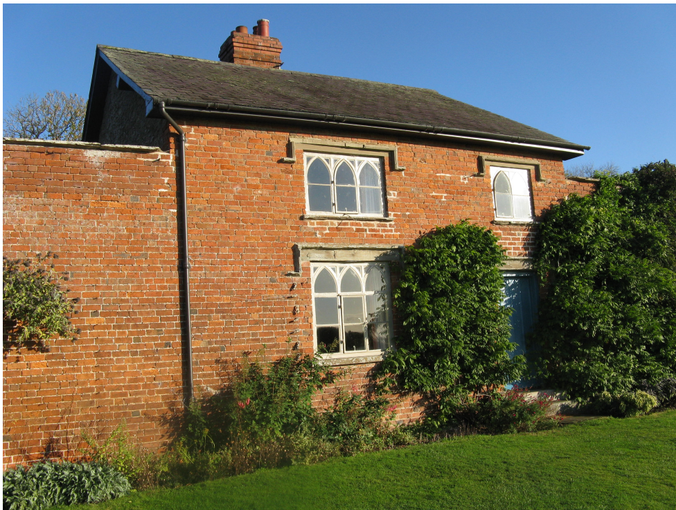
Plate 11 - Cottage (K) looking north
