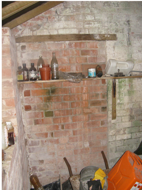
Plate 2 - Blocked doorway in (P) looking east
