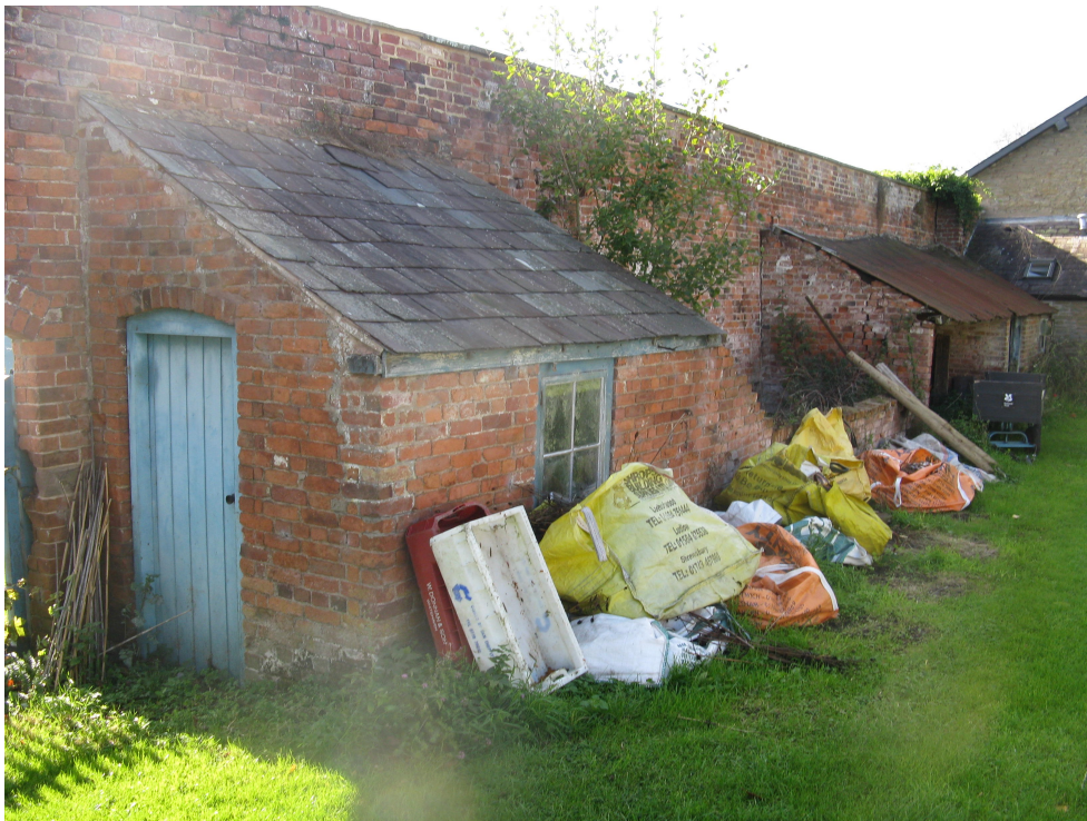
Plate 9 - Boiler house (T) looking west
