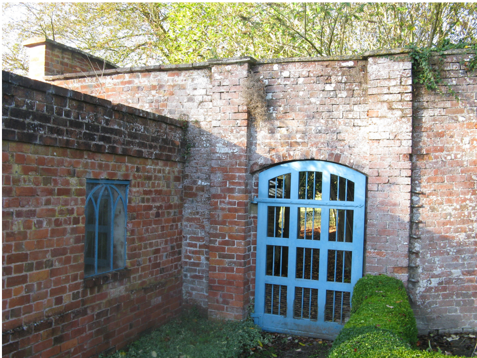
Plate 12 - Doorway (M) looking west
